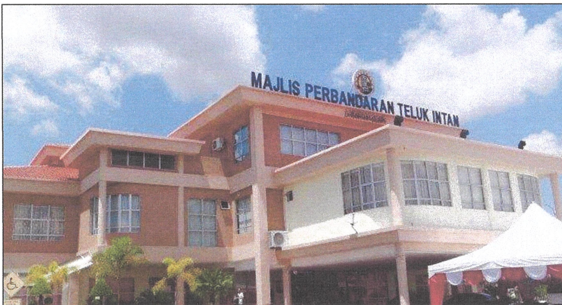
Image 1 : Building of Majlis Perbandaran Teluk Intan
