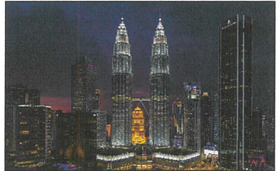
Figure 2: Petronas Twin Tower
