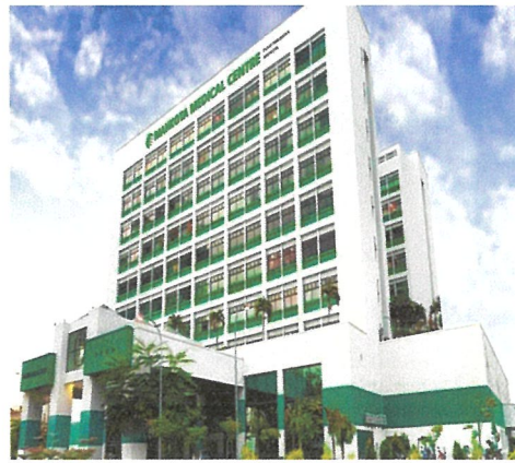
Figure 2.0 (a) shows a building of Mahkota Medical Centre.
