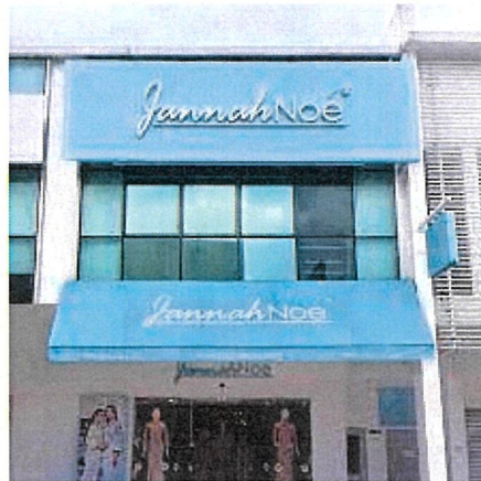
Figure 8.0 One of the outlet of JannahNoe
