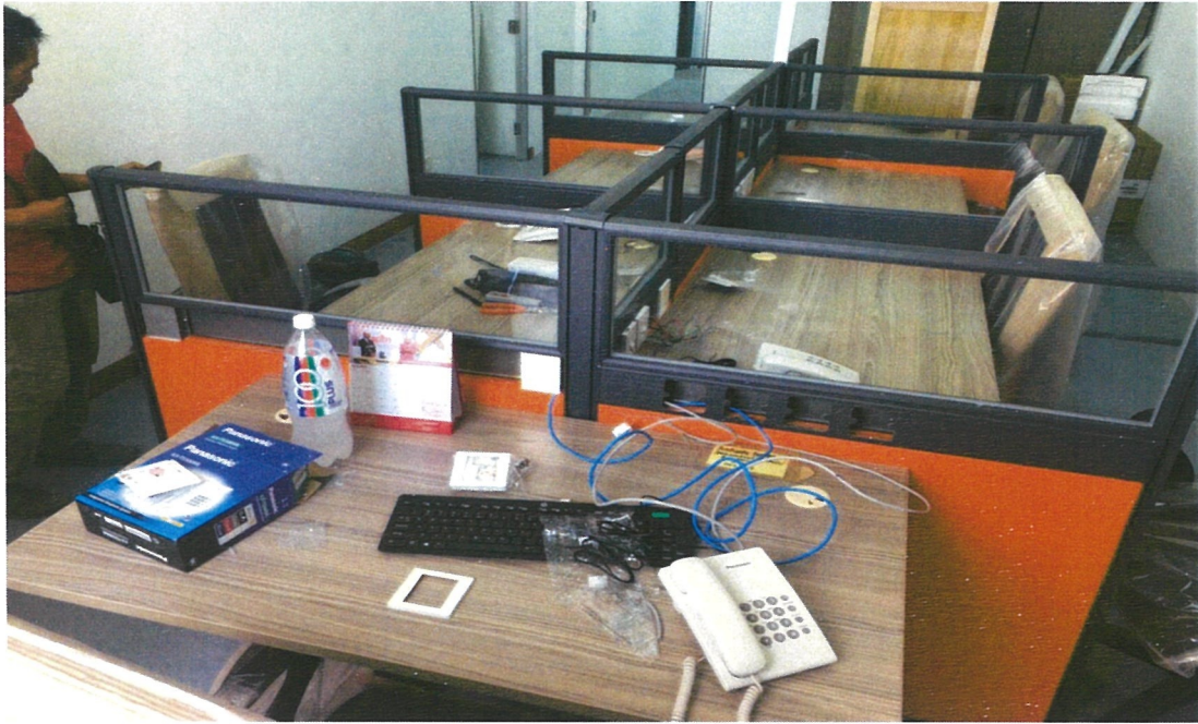
FIGURE 10: SUPPLY AND INSTALL OFFICE PARTITION AT SW CORP AT MASAI, JOHOR.
