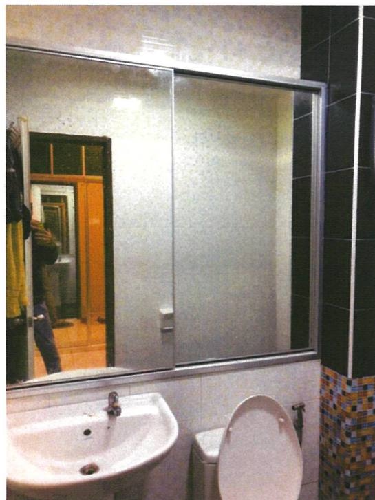
FIGURE 7: REPAIRING TOILET MIRROR CABINET
