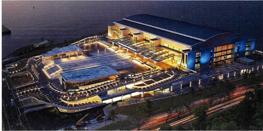
Figure 4: Building of SICC from above angle
