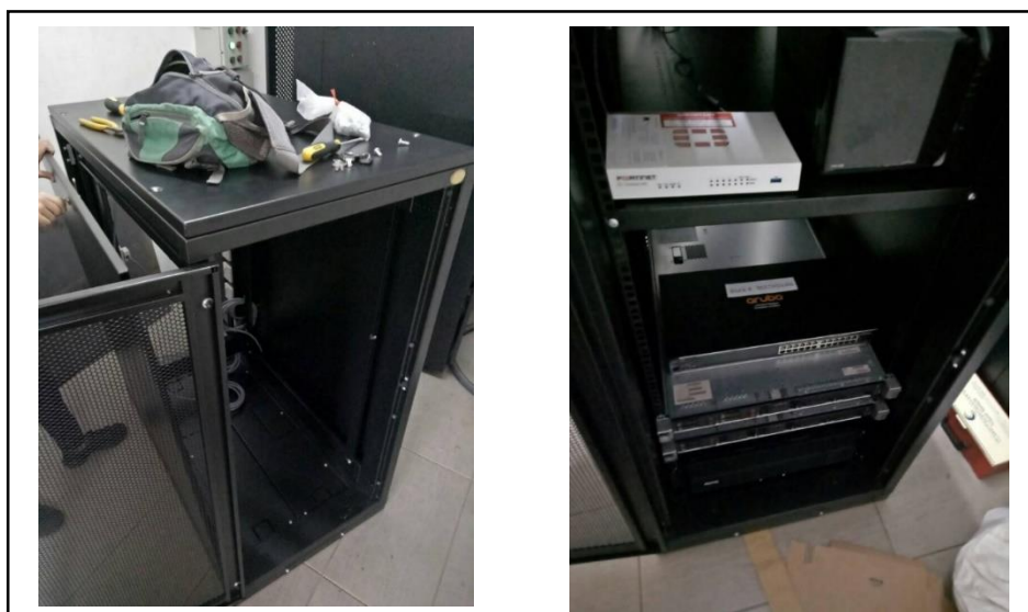
Figure 2.7 Before and After installation
