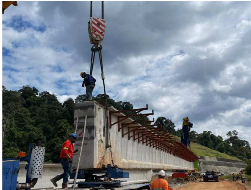
Figure 3.15: Rigger Is Inserting The Sling Into The Beam
