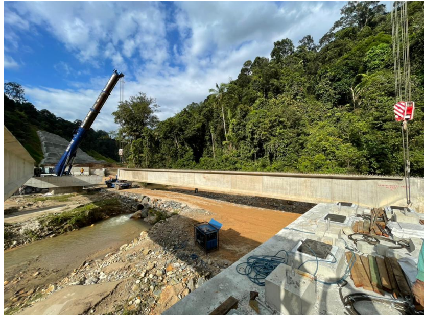
Figure 3.19: Placing Beam on its Position
