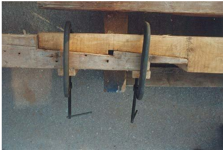
Figure 3.9 Timber Wedges
