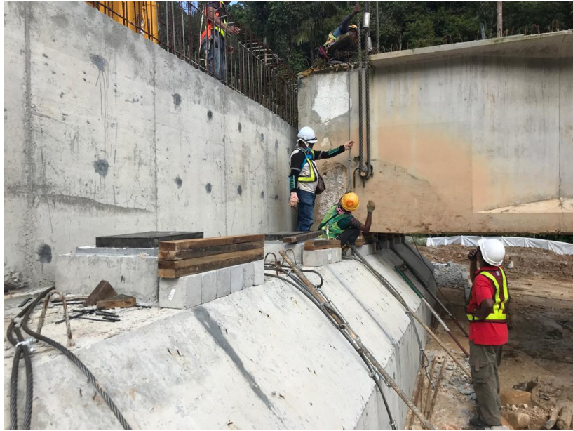
Figure 3.23: Removing Sling From the Beam
