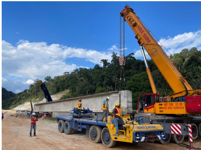
Figure 3.16: Preparing The Beam To The Launching Site
