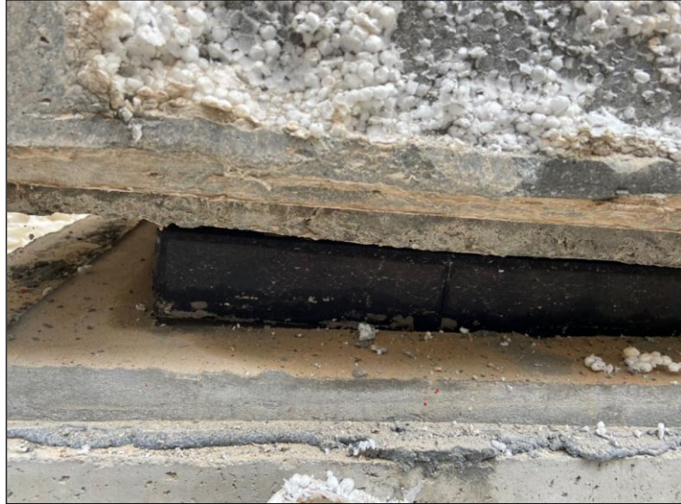
Figure 3.7: Bearing Pads
