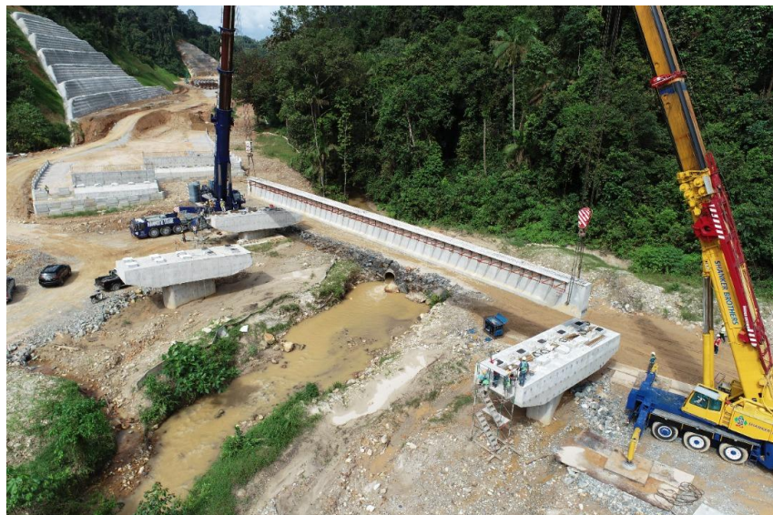
Figure 3.18: Placing Beam on its Position
