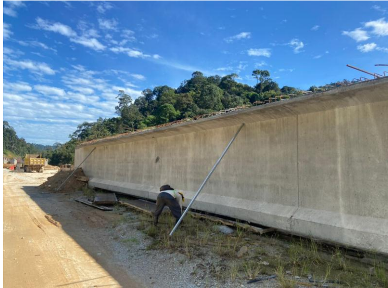
Figure 3.10: Post-Tensioned Beam (PTT)
