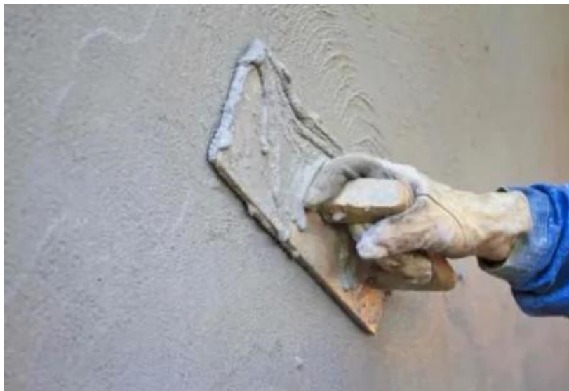
Figure 3.3.1.1 Example photo of plastering
