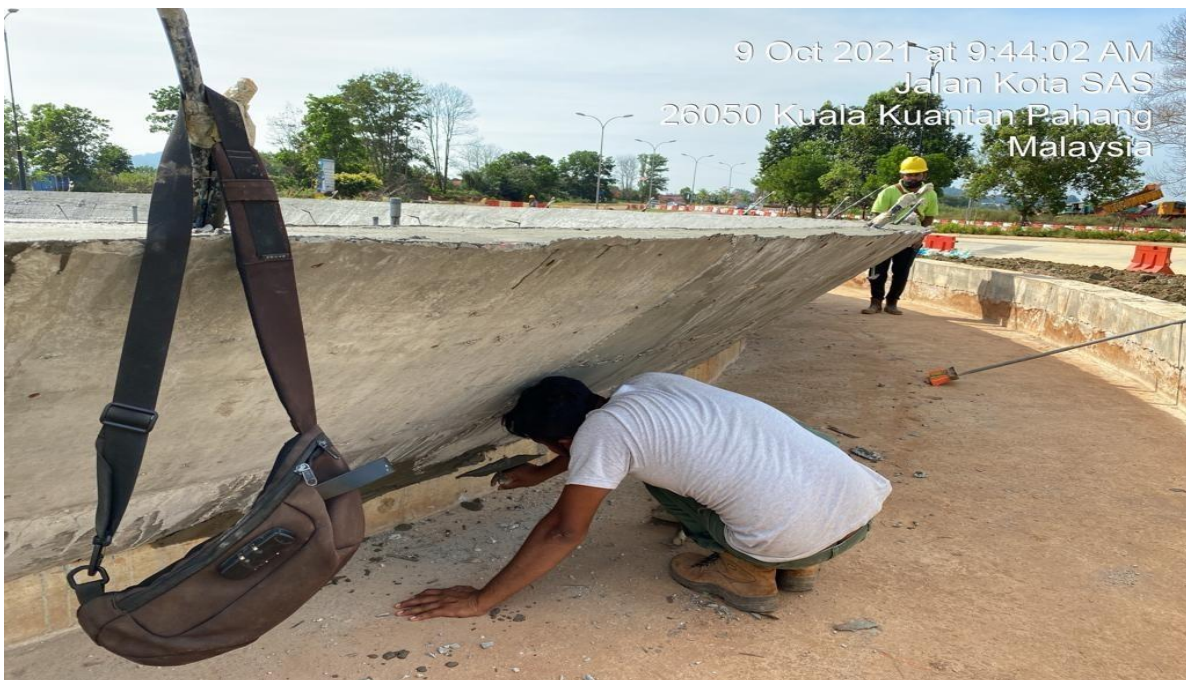
Figure 3.2.1.1 Plastering Works by workers
