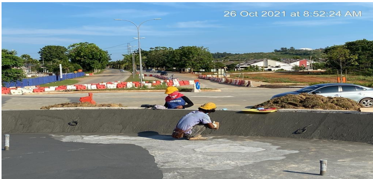
Figure 3.2.2.2 Installation waterproofing Formdex Uniflex Application
