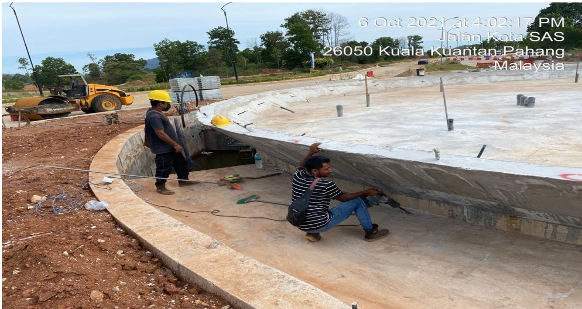
Figure 3.2.2.1 Surface preparation
