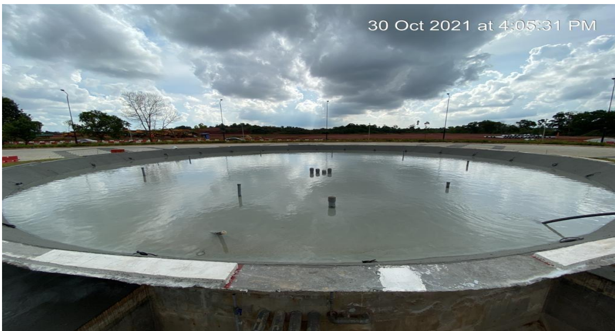
Figure 3.2.2.3Ponding test
