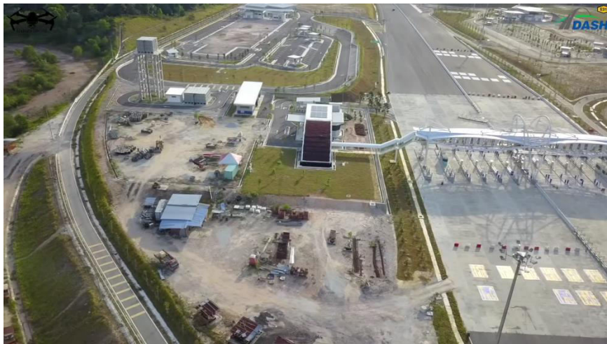
Figure 1 : View of Denai Alam Toll Plaza (TP1) taken a drone
