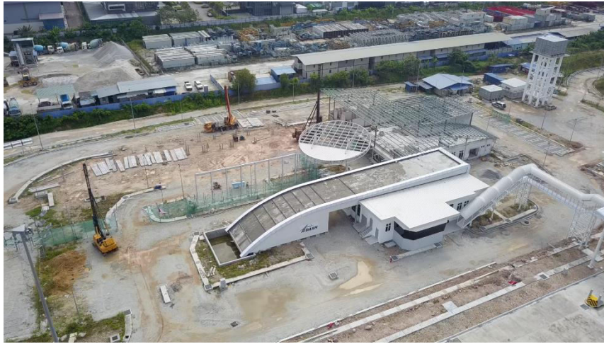
Figure 2 : View of RRIM Toll Plaza (TP2) taken from a drone
