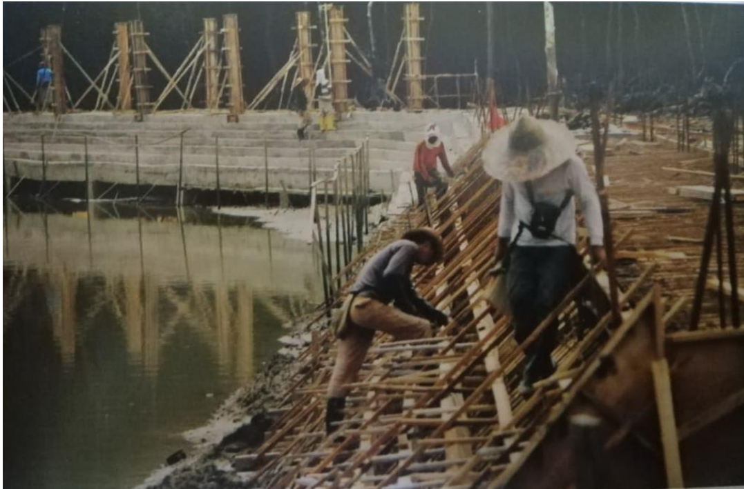
Figure 2.9 Renovation works at Merlimau Jetty
