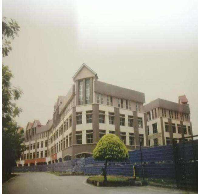
Figure 2.7 Building refurbishment works at Pulau Melaka.
