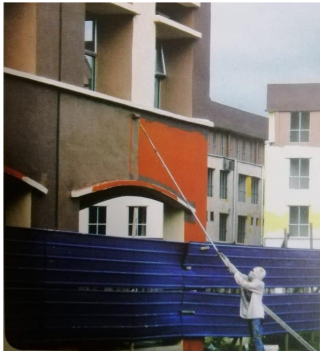
Figure 2.6 Building refurbishment works at Pulau Melaka.
