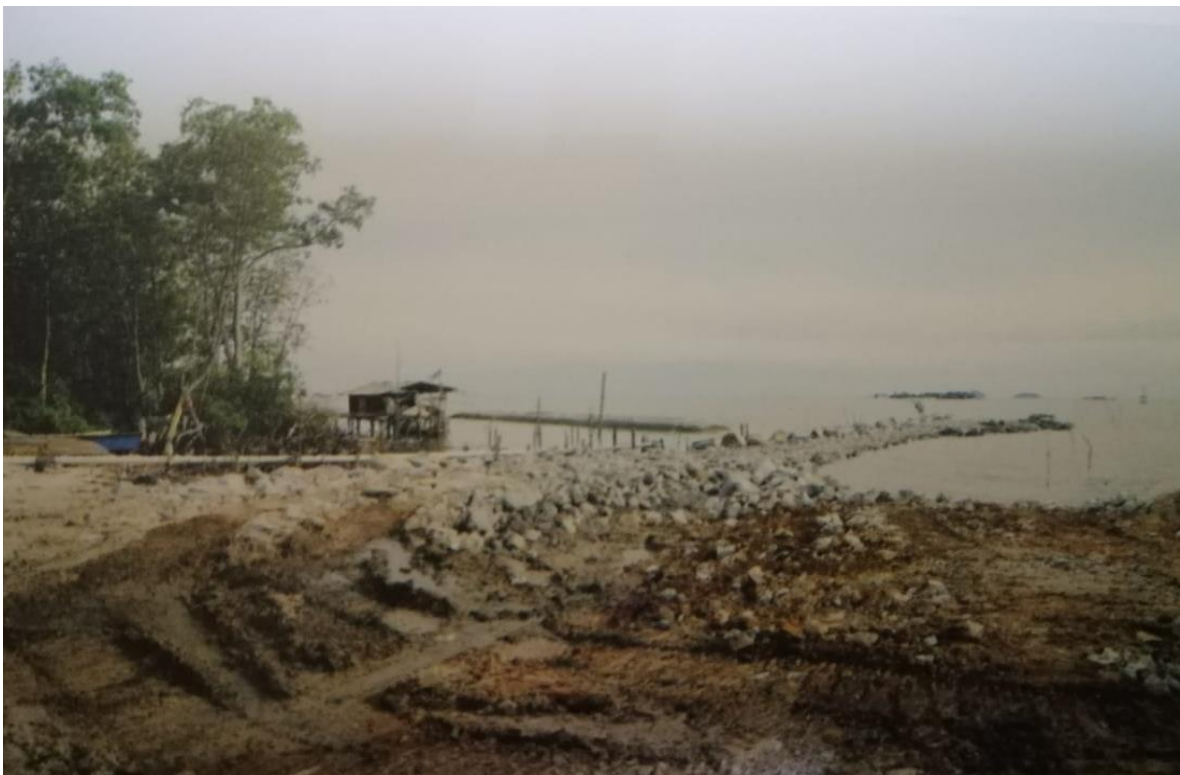
Figure 2.8 Sea reclamation work.
