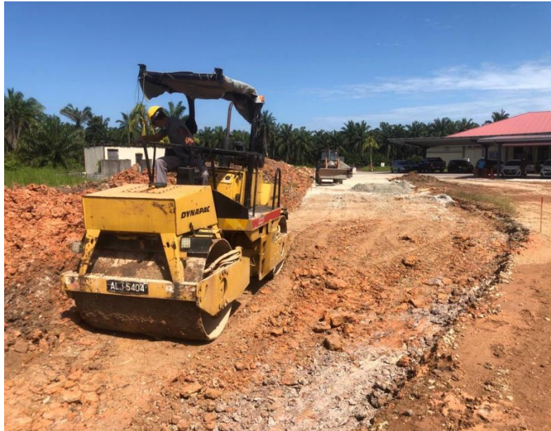
Figure 3.2.6. Compacting The Crusher Run
