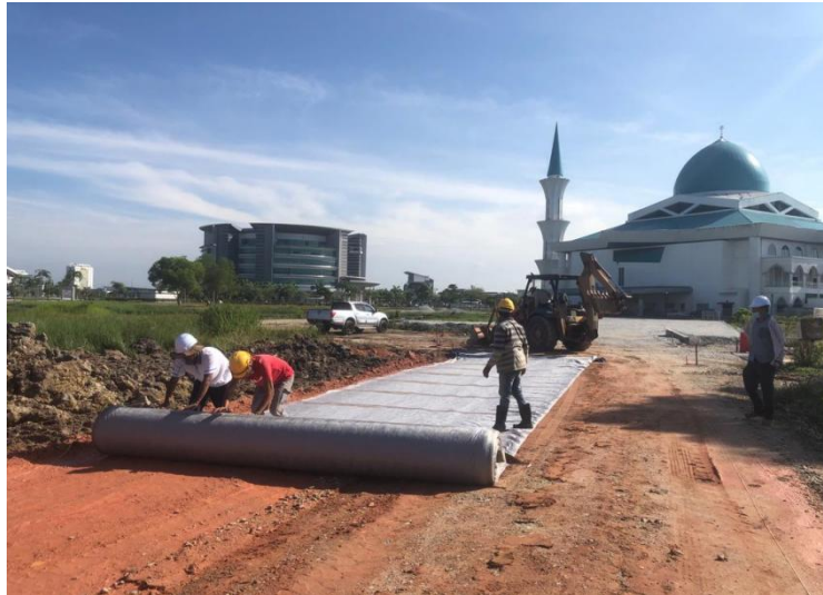
Figure 3.2.5. Laying The Geo-textiles
