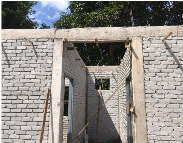
Figure 3.25: finishing brickwork of bathroom section
