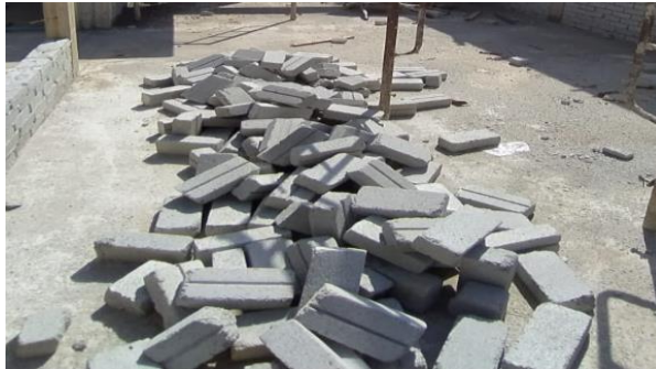
Figure 3.4: the brick lifted at the construction work
