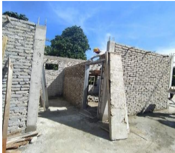
Figure 3.24: brickwork process of bedroom 2
