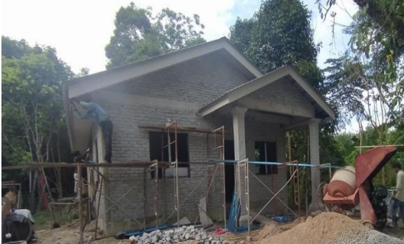
Figure 3.30: brickwork on the top of roof beam
