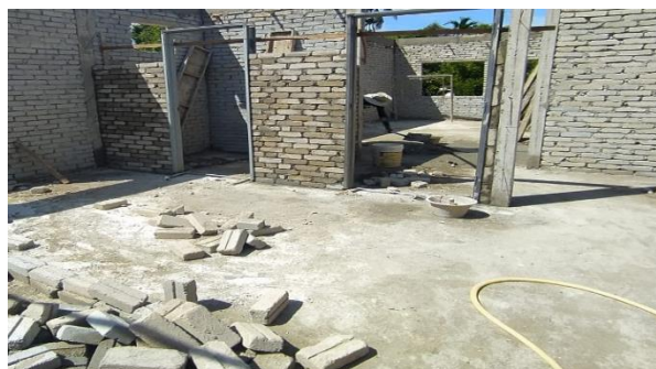
Figure 3.18: brickwork process of bathroom in master bedroom
