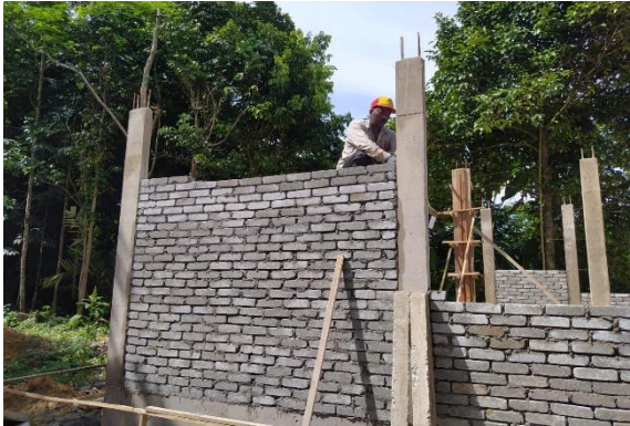
Figure 3.19: brick laying at kitchen section
