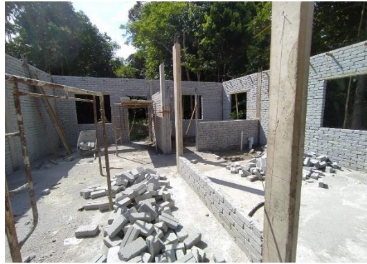
Figure 3.21: brickwork process for bedroom 1
