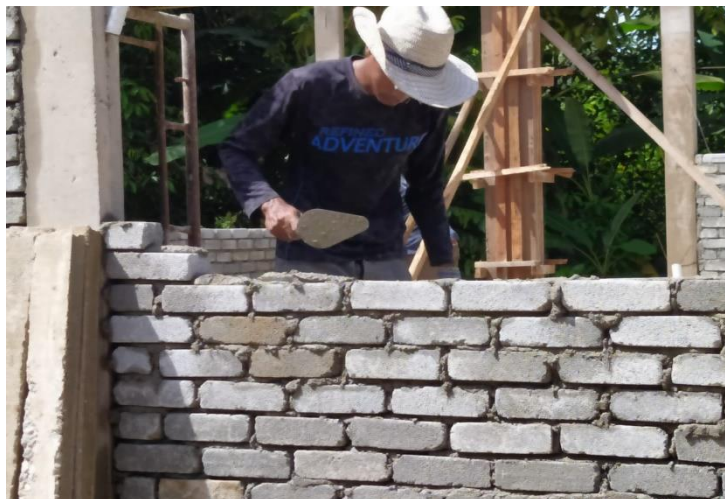
Figure 3.7:bricklaying process
