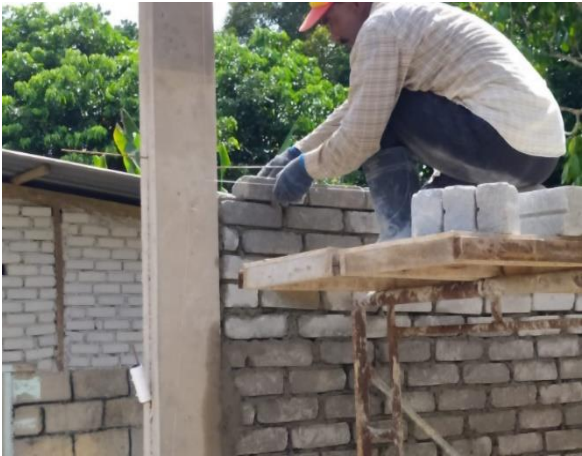
Figure 3.20: brick laying interior side
