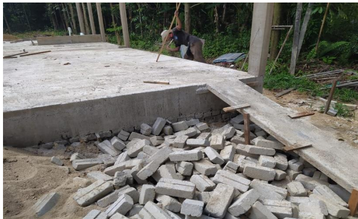
Figure 3.3: the floor that has been cleaned before start the bricklaying process
