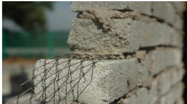
Figure 3.8: exmate wire in the layer of brick wall
