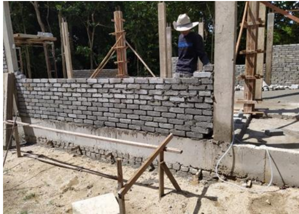
Figure 3.16: brickwork at the beginning of the master bedroom
