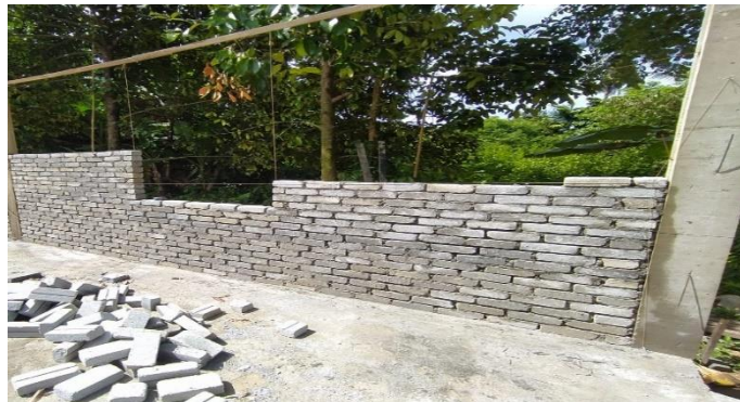
Figure 3.28: brickwork at living area
