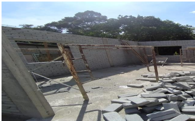
Figure 3.26: brickwork at dining area
