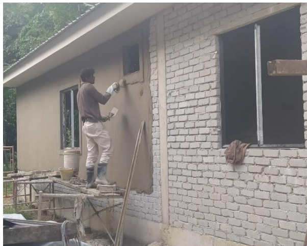
Figure 3.12: the plastering work to exterior wall had been taken
