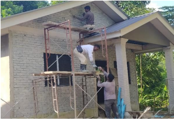
Figure 3.31: final inspection of brick laying before plastering process
