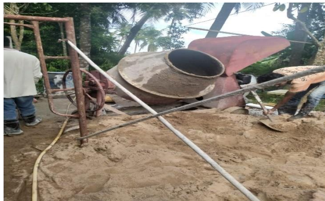
Figure 3.5: mortar are mixed using concrete mixer
