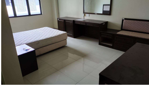
Photo 3.1: Photo shows a completed installation of ceramic tiles.
