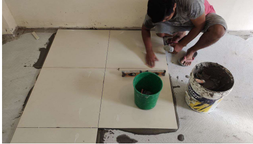
Photo 3.30: Photo of the installation of tiles
