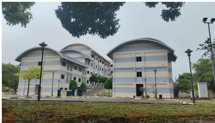
Photo 1.1: Photo Shows a Building of Akademi Audit Negara (Hostel)
