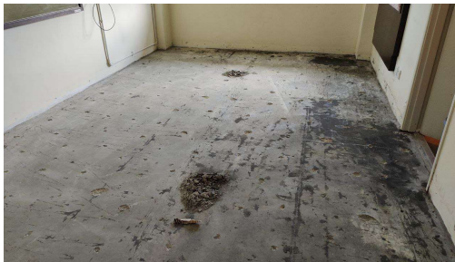
Photo 3.28: Photo of the floor that have been hack.
