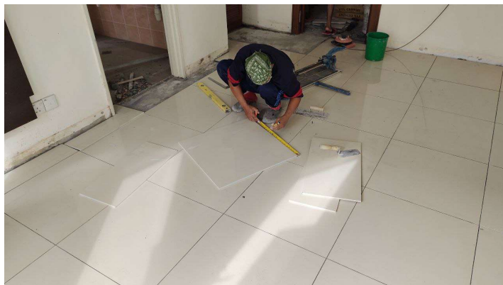
Photo 1.3: Photo shows tiles installation
