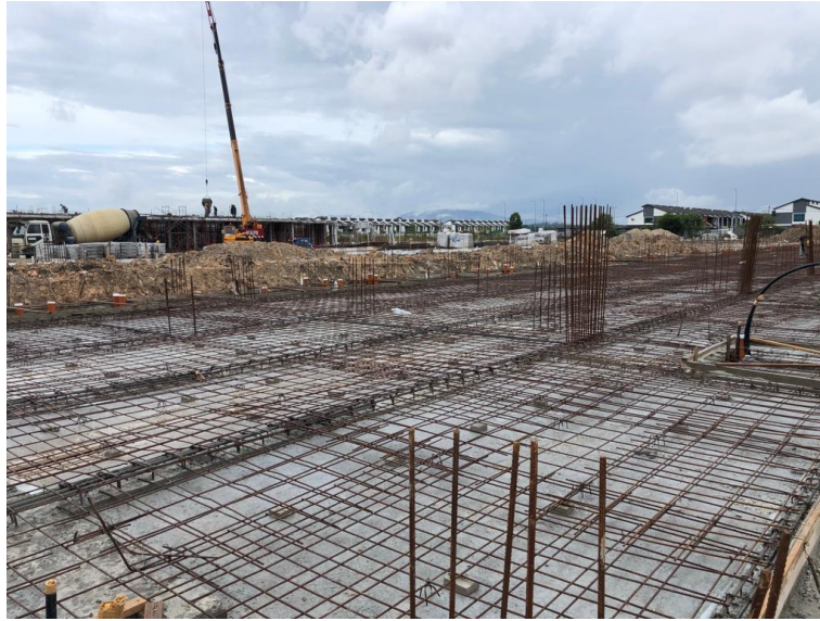
Figure 46: Image shows completed BRC installation for ground floor slab.
