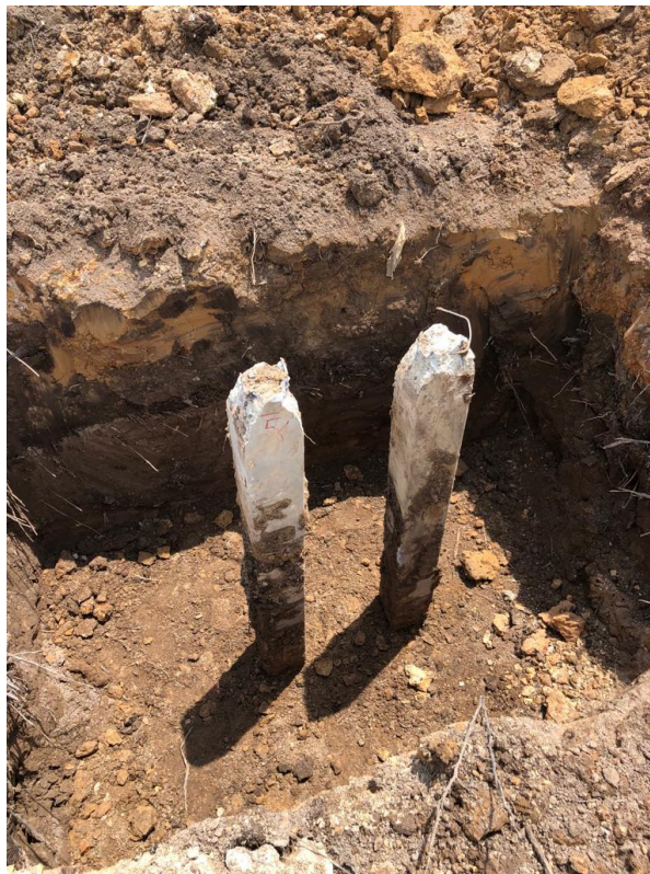
Figure 28: Image shows excavated pile cap point.
