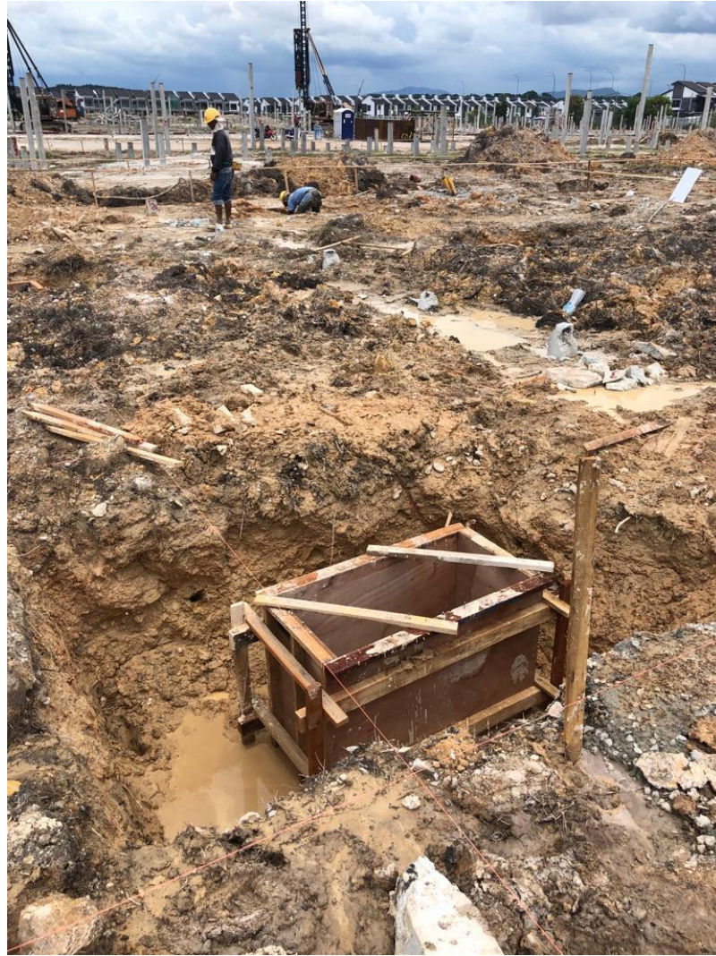
Figure 30: Image shows installation of pile cap formwork.
