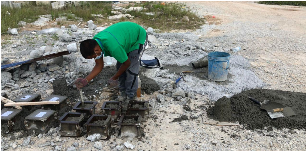
Figure 16: Image shows concrete cube filling and slump test on site
