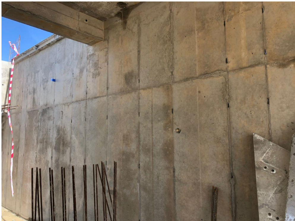
Figure 60: Image shows shear wall after opening of aluminium formwork.
