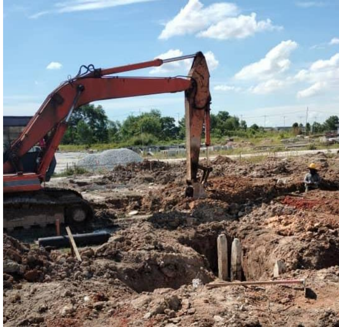
Figure 27: Image shows excavation works for pile cap.
