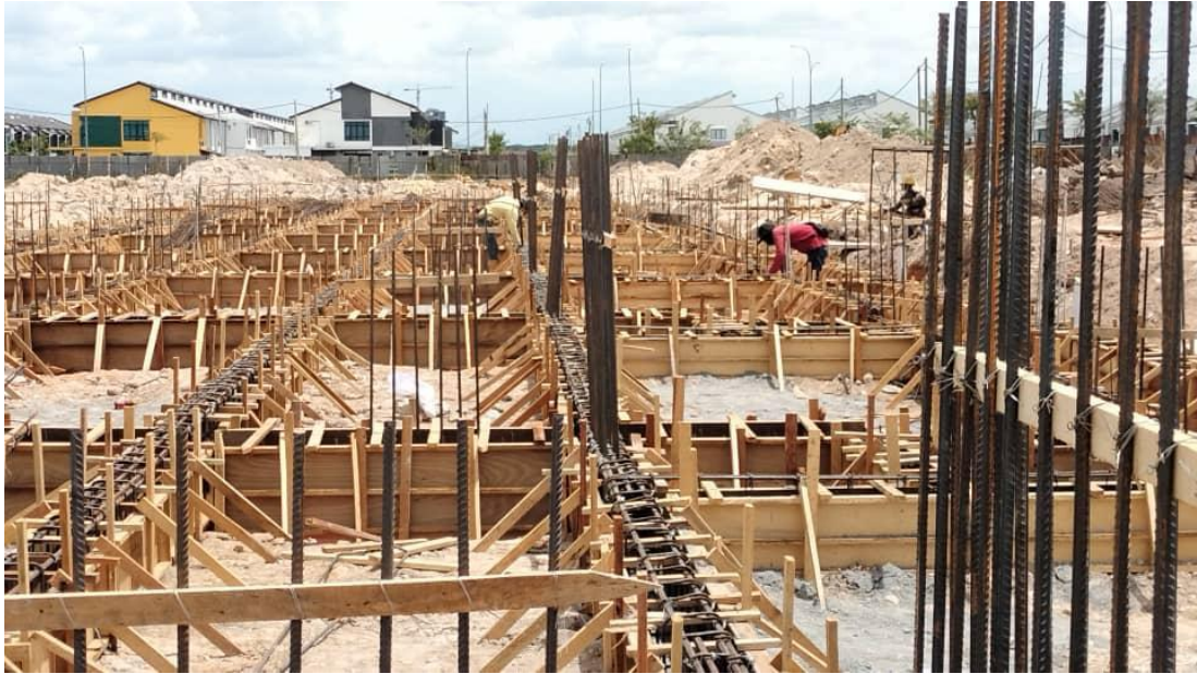
Figure 37: Image shows the completed installation of reinforcement bars for ground beam.
