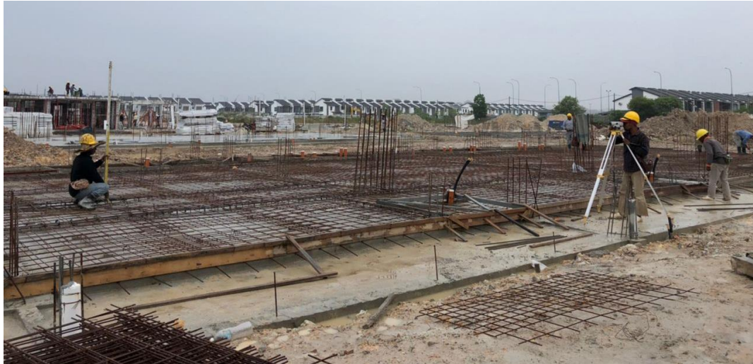
Figure 47: Image shows levelling taken for ground floor slab top surface.
