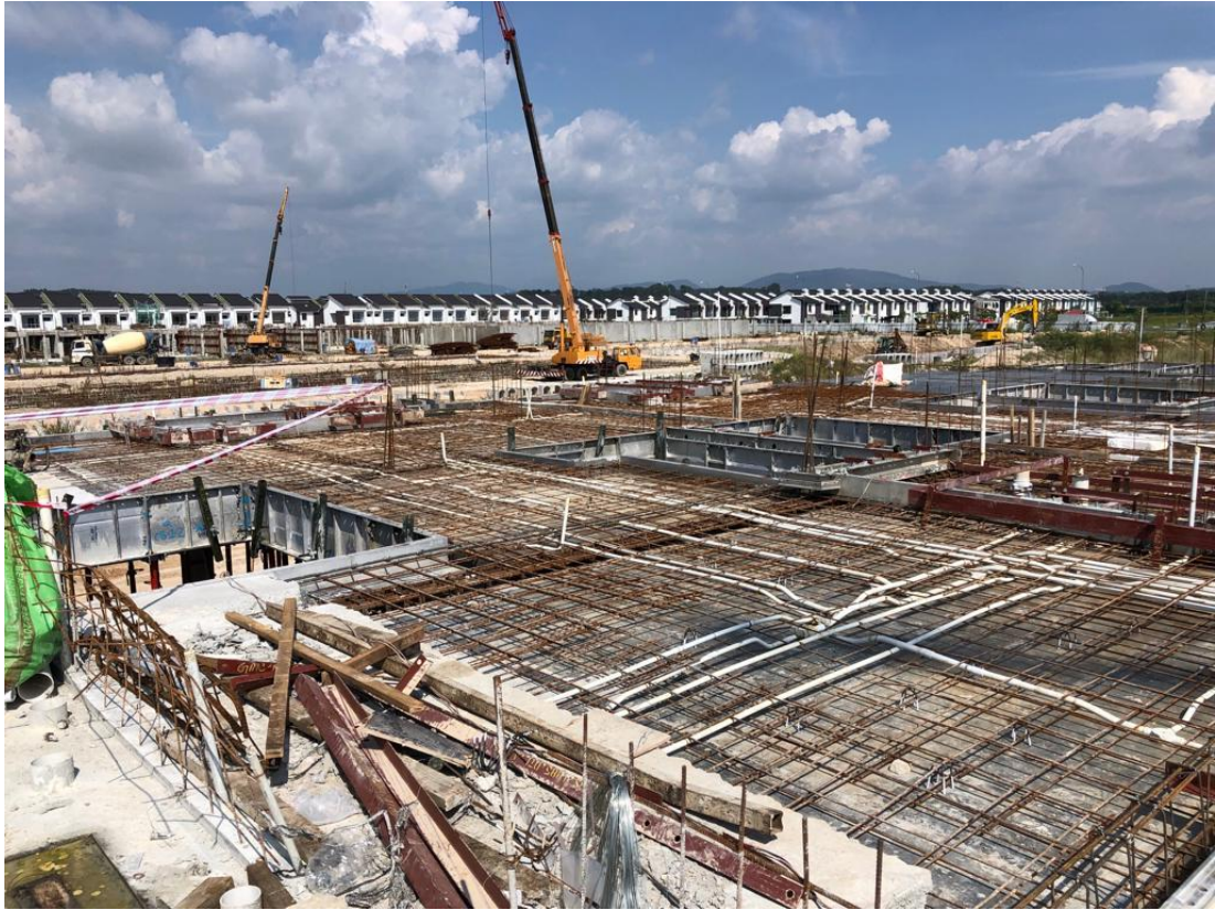
Figure 58: Image shows the completion of 1st floor beam and slab.
