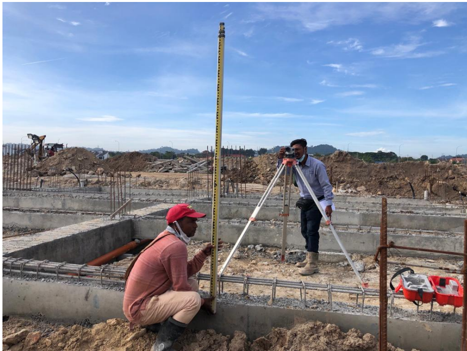
Figure 40: Image shows the process of levelling for ground floor slab.
