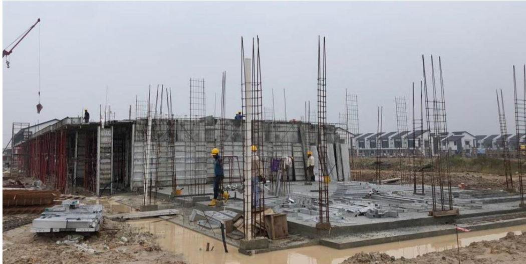
Figure 51: Image shows completed installation of reinforcement bars for ground column.
