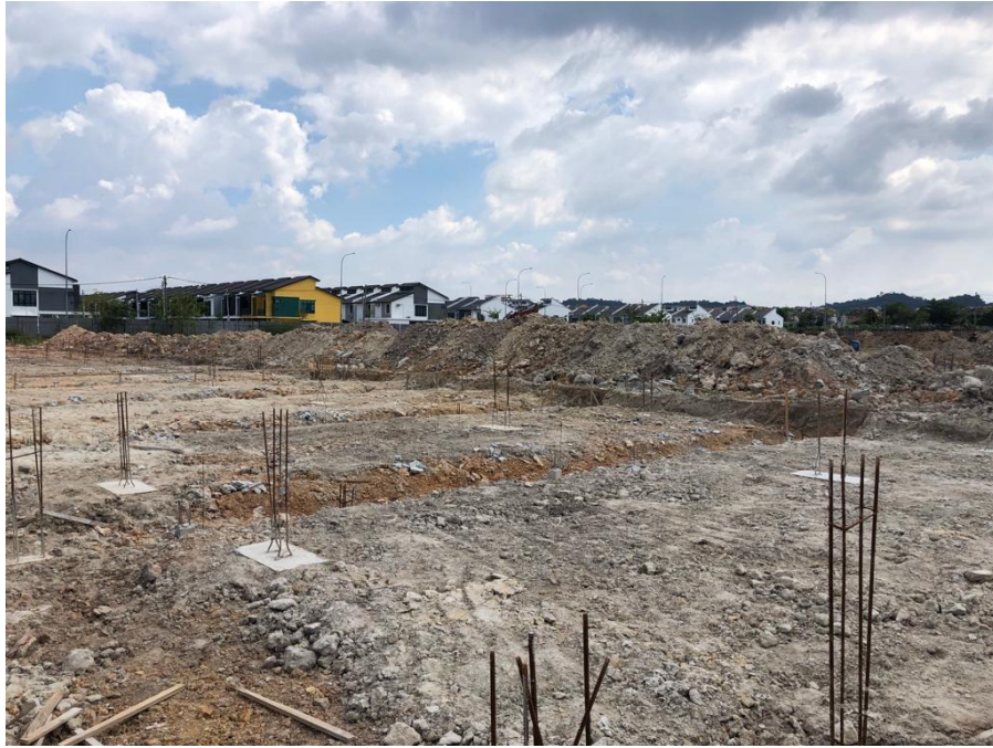
Figure 34: Image shows the excavation site for ground beam works.
