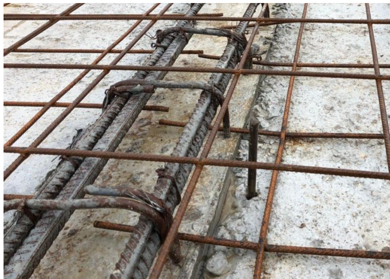
Figure 48: Image shows the steel bar indicator for mason workers.
