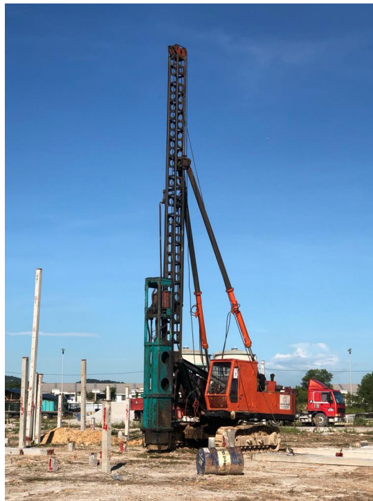
Figure 6: Image shows a piling frame used in this project.
