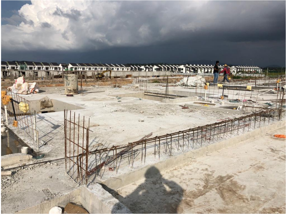
Figure 61: Image shows completed 1st floor slab.
