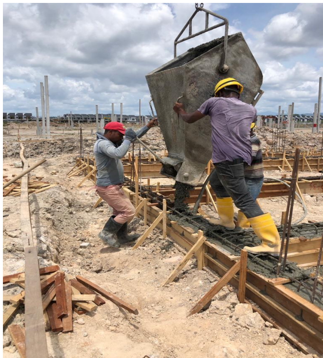
Figure 38: Image shows the concreting process of ground beam.
