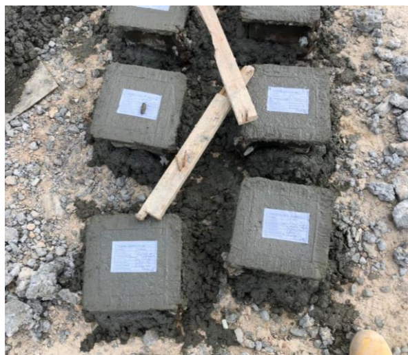
Figure 17: Image shows concrete cube to be submitted to the laboratory for strength test.
