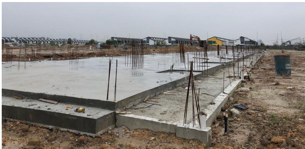
Figure 49: Image shows completed ground floor slab.
