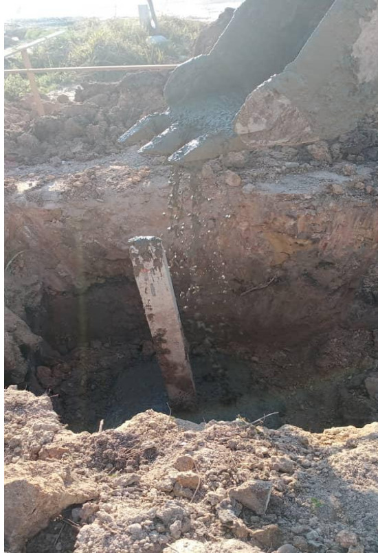
Figure 29: Image shows lean concreting of pile cap.
