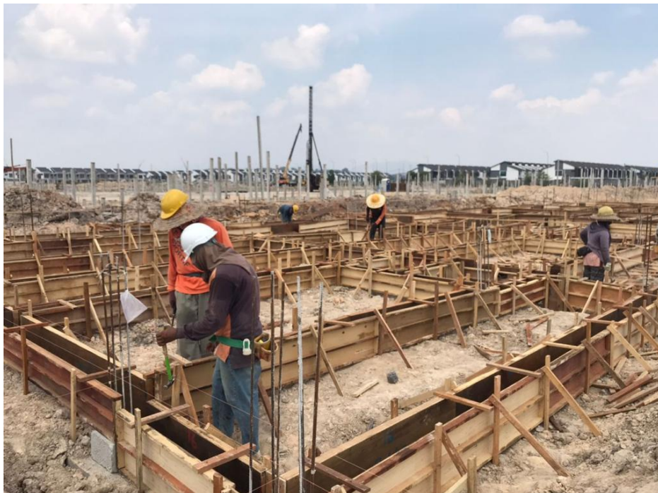
Figure 35: Image shows installation formwork ground beam.
