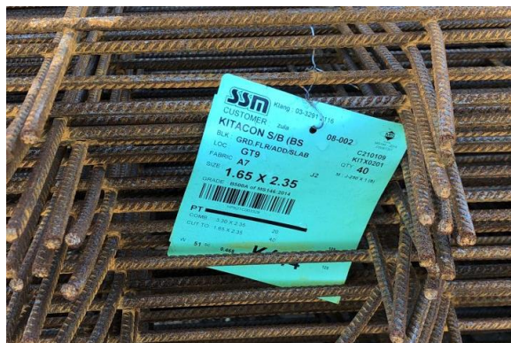
Figure 45: Image shows 'tag' attached to BRC delivered on site.
