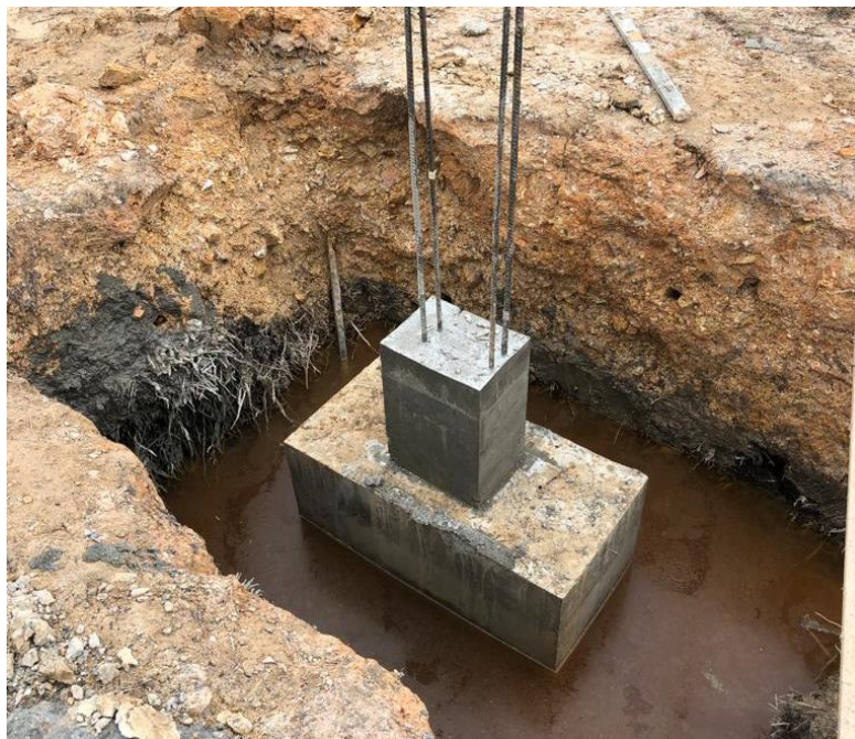
Figure 32: Image shows a completed pile cap.
