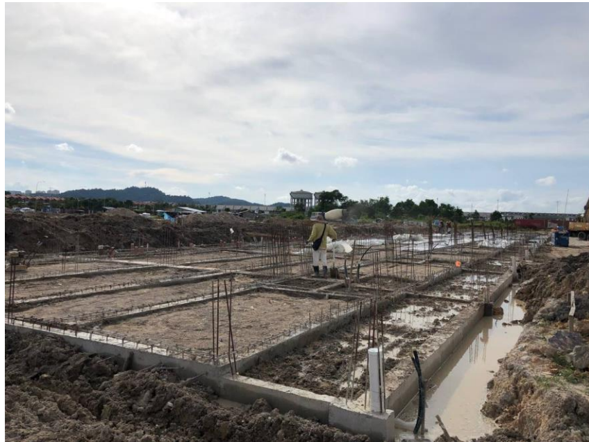
Figure 41: Image shows compacted 'backfilled' earth for ground slab.
