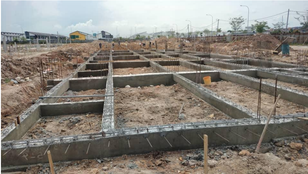
Figure 39: Image shows the completed ground beam of 6 units.
