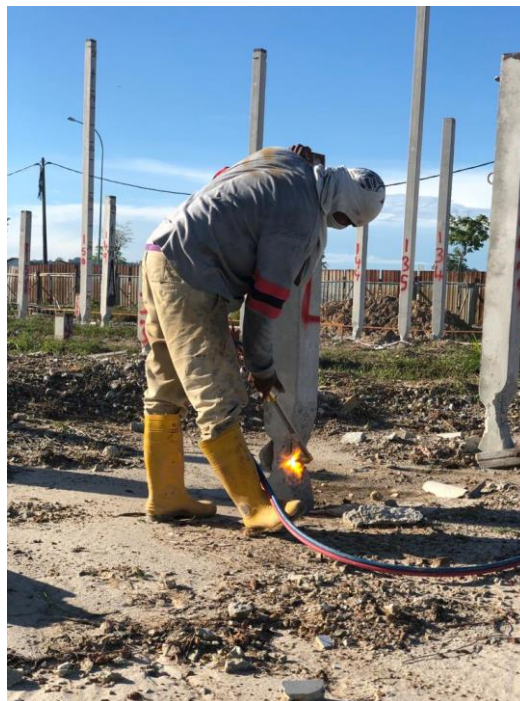
Figure 15: Image shows piling cutting works
