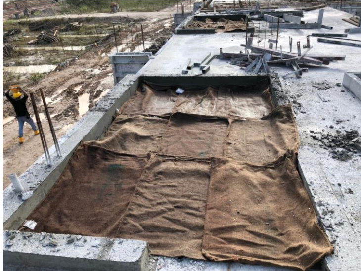
Figure 23: Image shows the curing of Bathroom.
