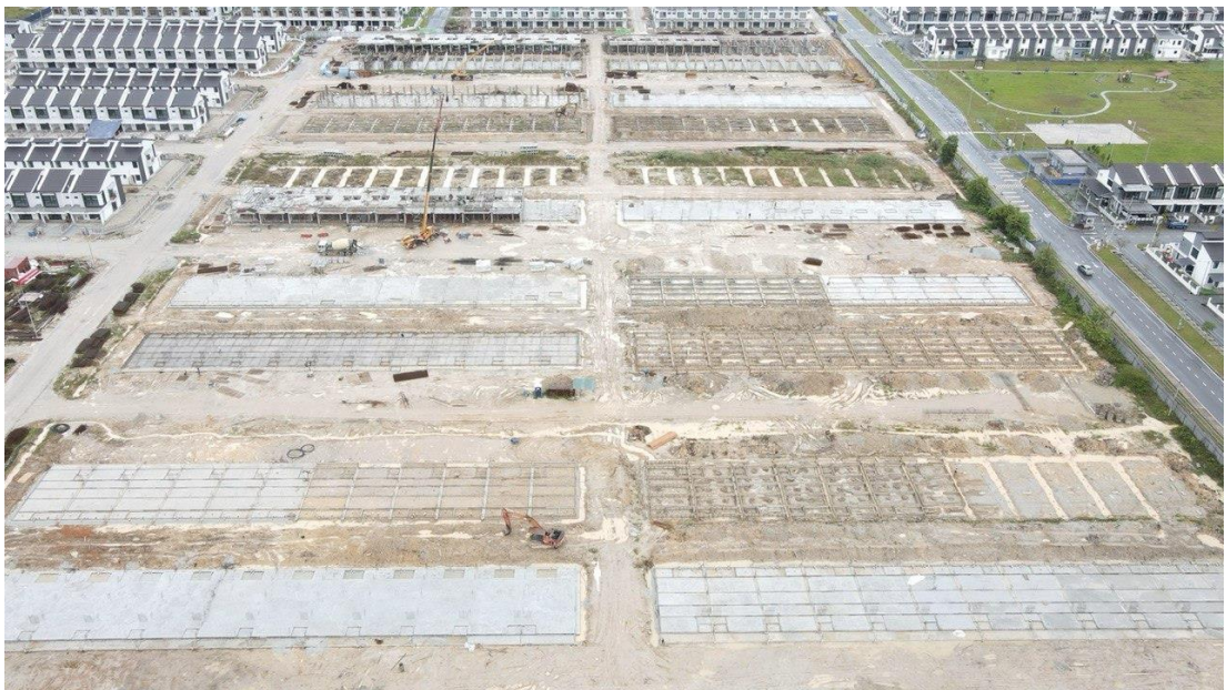
Figure 4: Image shows the site progress as of 3/1/2022
