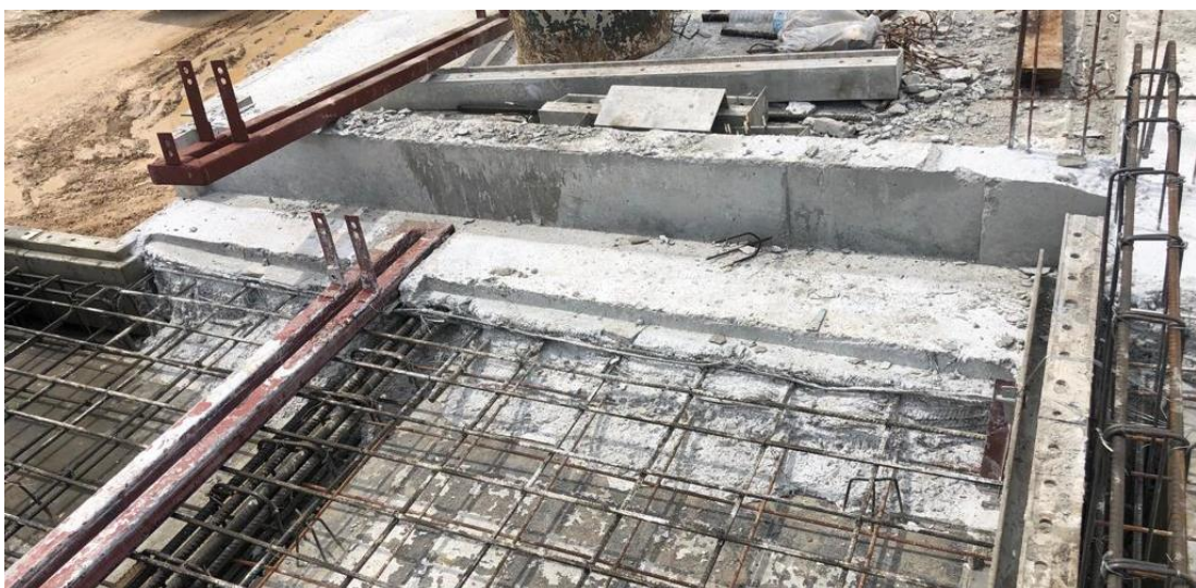
Figure 24: Image shows a construction joint for 1st floor slab.
