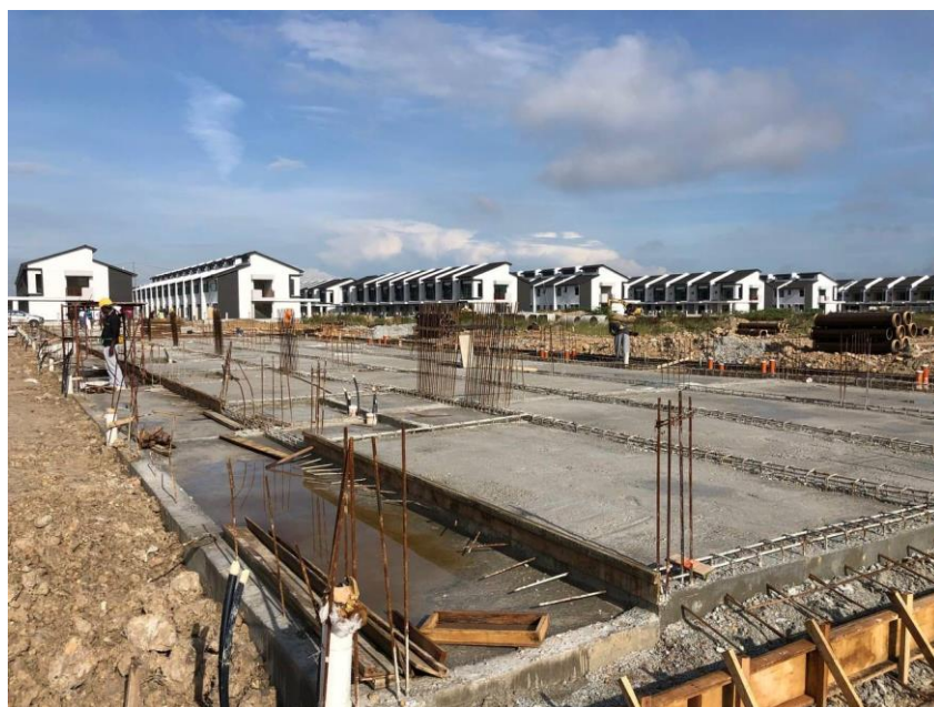
Figure 42: Image shows completed lean concreting of ground slab.
