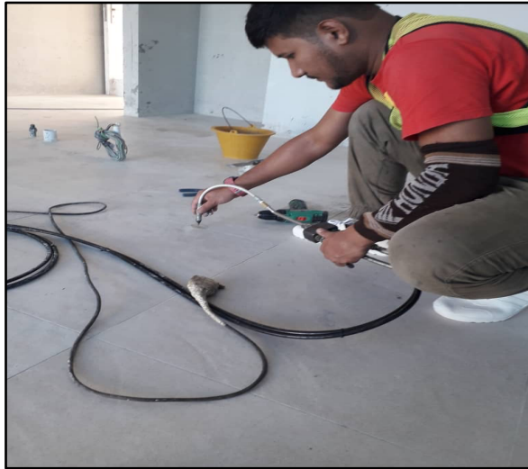
Figure 19 : Stop injection after the pressure remains unchanged
