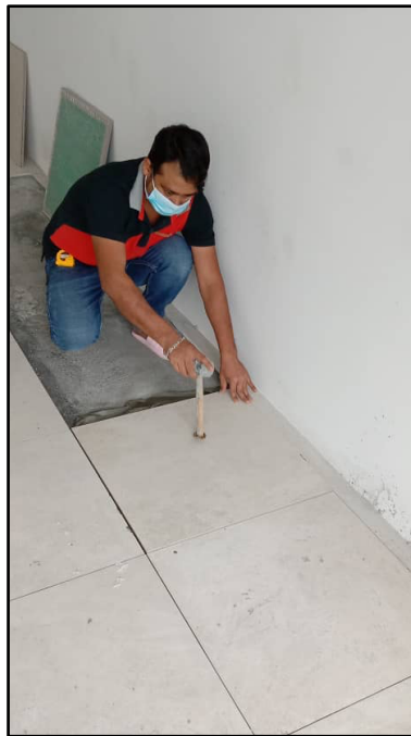
Figure 22 : Checking for hollowness
