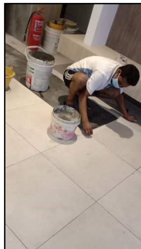
Figure 20 : Laying floor tiles
