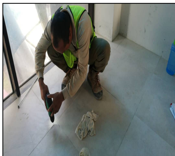
Figure 17 : Drill holes at tiles jointing
