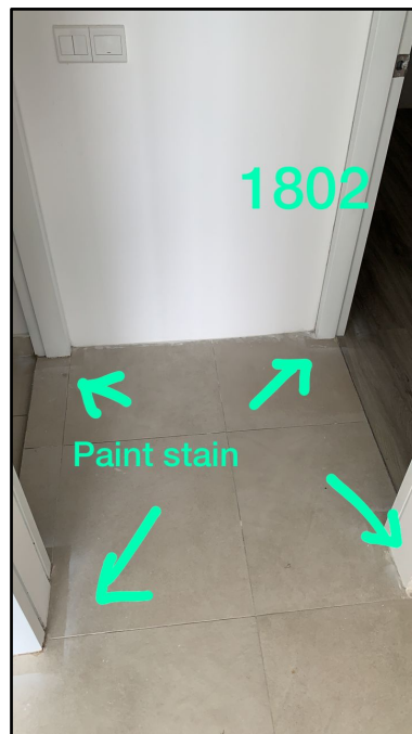
Figure 25 : Paint Stains
