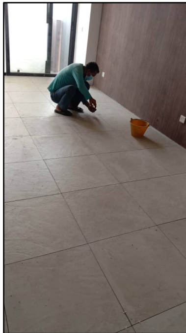
Figure 21 : Remove Surplus Dust And Cement
