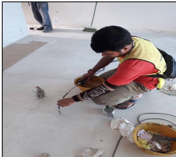
Figure 18 : Ready for injection
