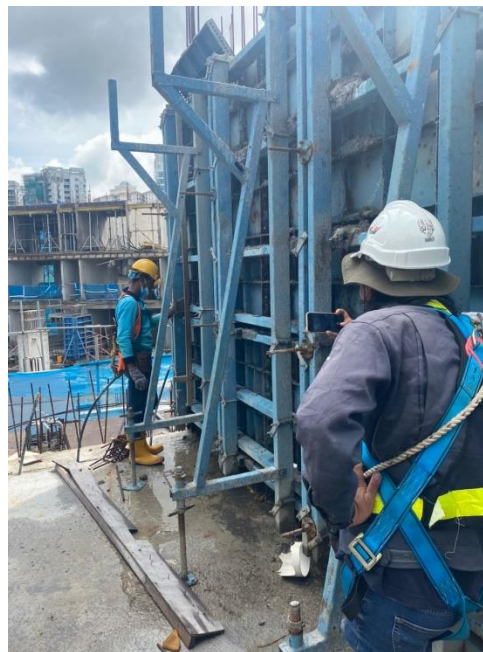
Figure 3.29: Shows the verticality inspection process by main contractors and consultant
