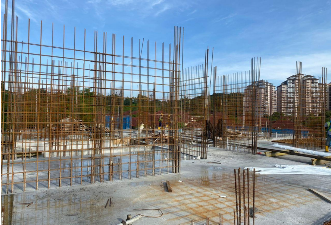
Figure 3.34: Block 2 Zone 3 Level 4 before cast
