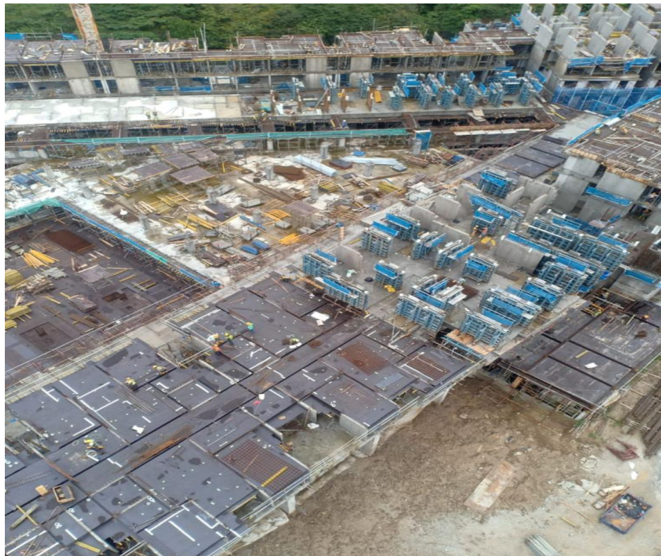
Figure 3.5: Project's view from Tower Crane 2
