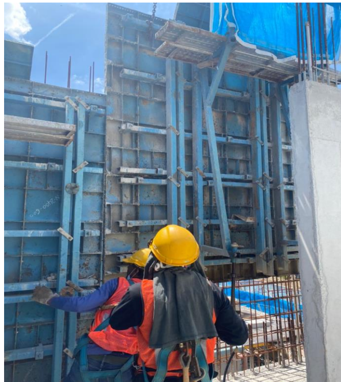
Figure 3.24: Shows the adjacent ganged formwork installation ongoing
