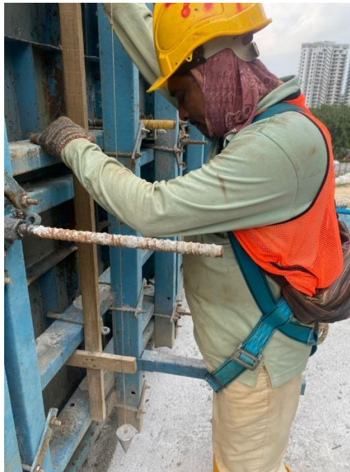
Figure 3.22: Shows the verticality checking of the ganged formwork panels
