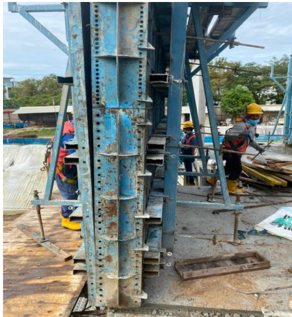
Figure 3.28: Shows the installation of external shear wall opposite side
