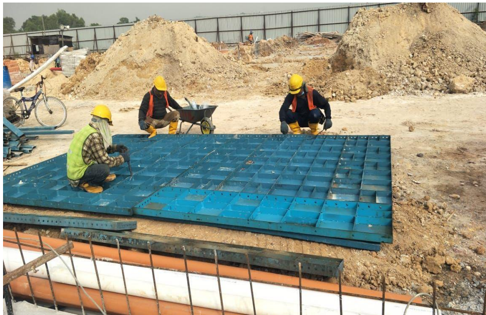
Figure 3.14: Shows the modulation of the formwork panels
