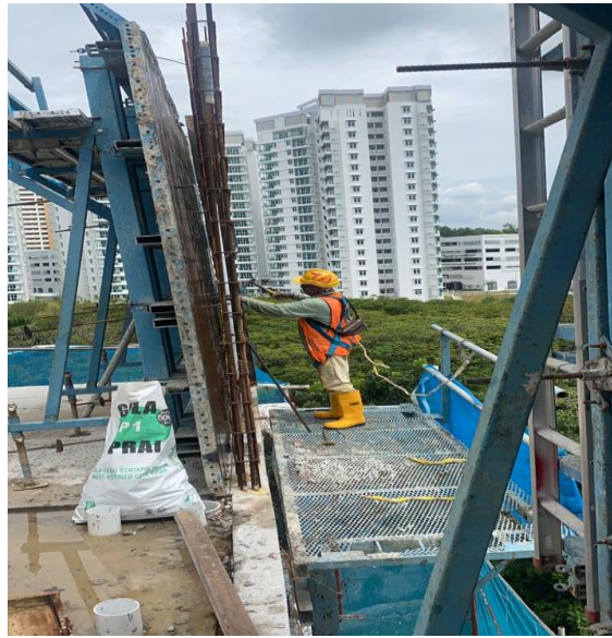
Figure 3.27: Shows the installation of external shear wall one side
