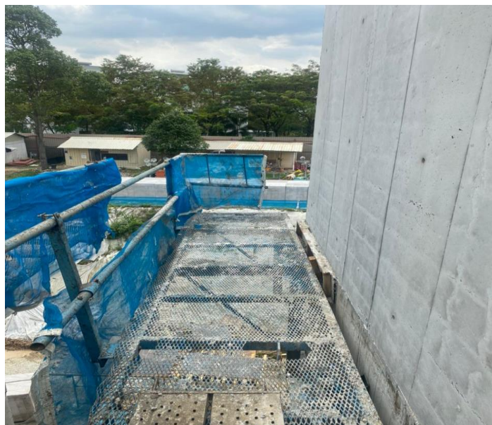
Figure 3.25: Shows the External Working Platform for external shear walls
