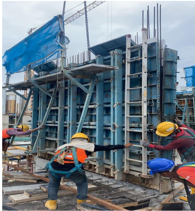
Figure 3.37: Shear walls carried using Tower Crane
