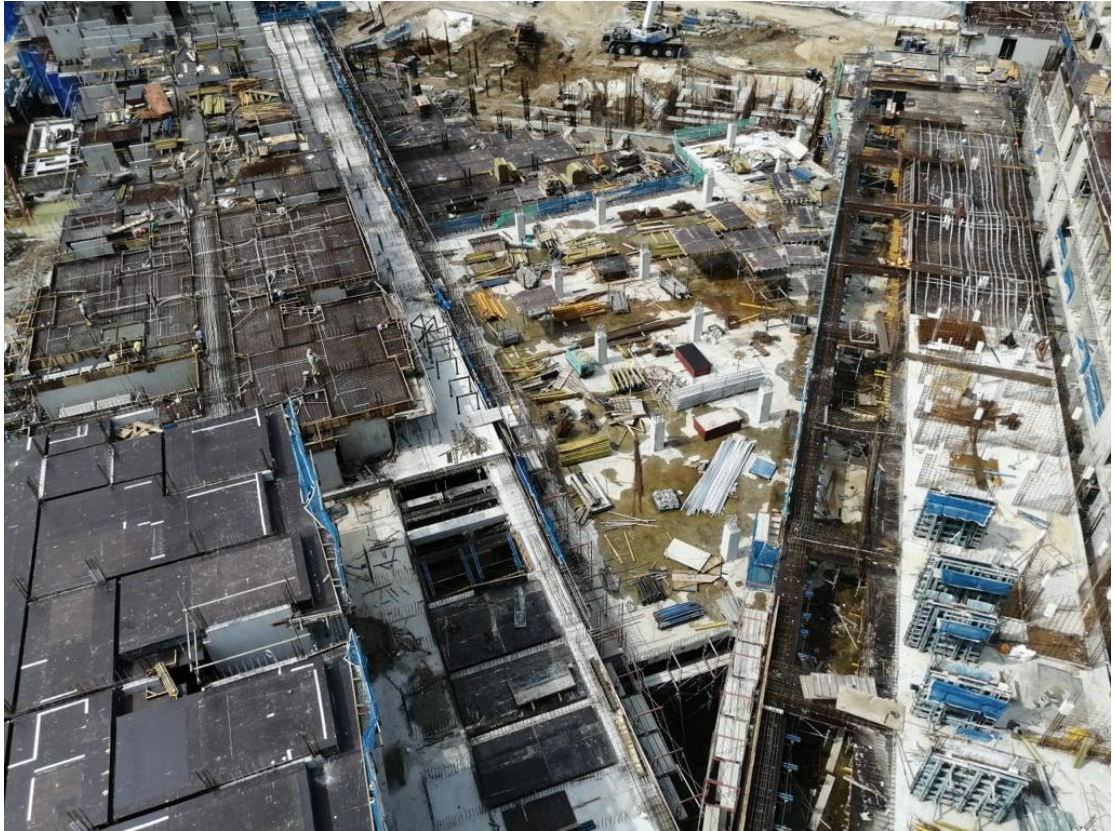
Figure 3.6: Project's view from Tower Crane 3
