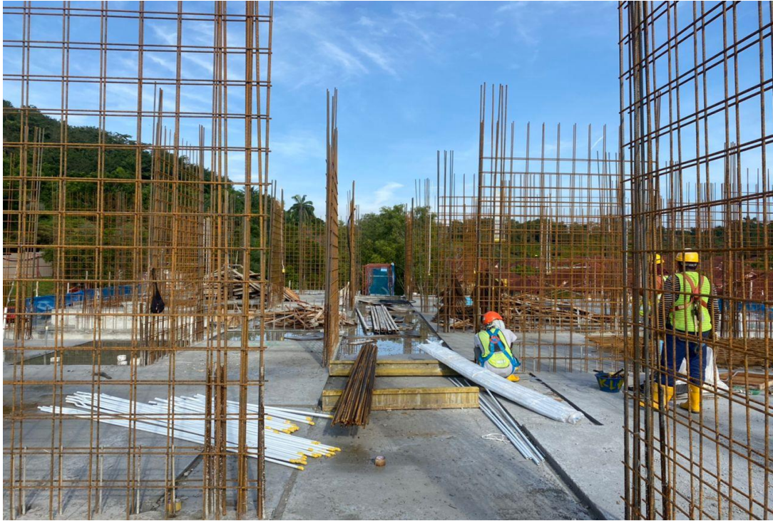
Figure 3.32: Block 2 Zone 1 Level 4 before cast
