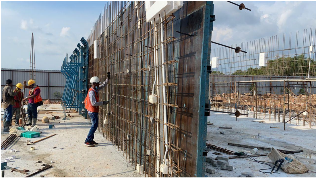
Figure 3.23: Shows the adjacent ganged formwork
