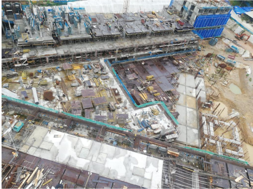
Figure 3.4: Project's view from Tower Crane 1
