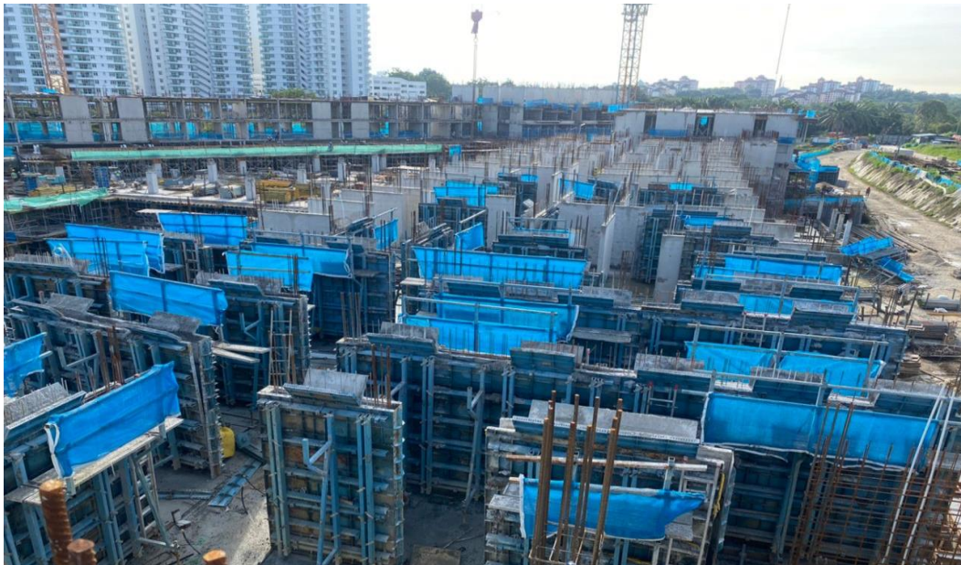
Figure 3.31: Block 2 Zone 2 Level 2 after finish cast
