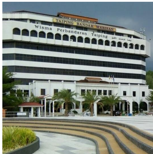
Figure 1.0 : Building of Taiping Municipal Council (MPT)
