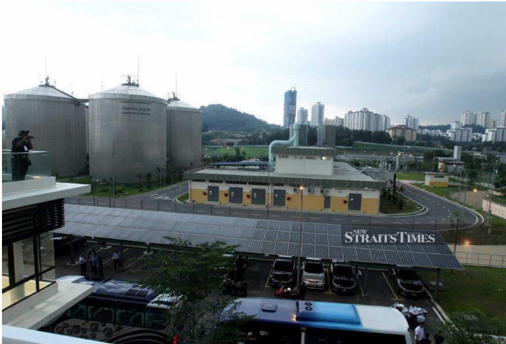
Figure 1.3 (1) IWK main hub at Pantai Eco Park Kuala Lumpur
