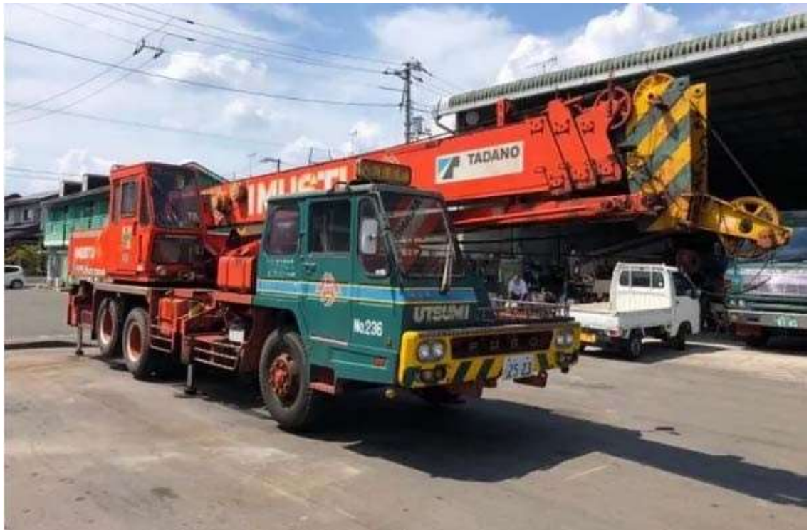
Figure 18: 25-ton crane lift and install PDA Test frame
