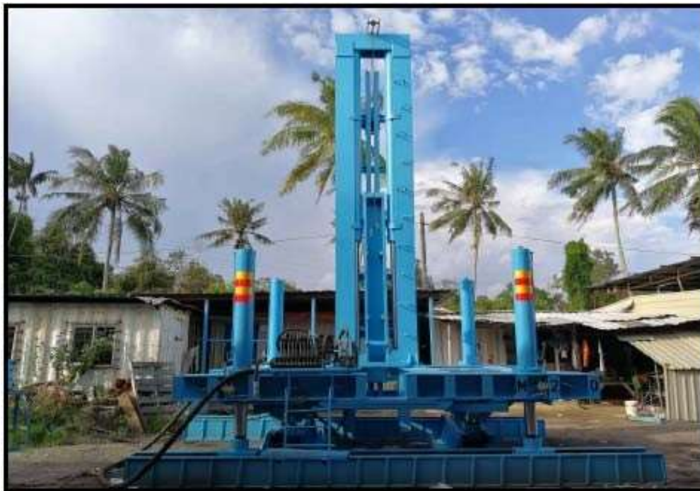
Figure 9: Hydraulic pile driver machine. (M20)
