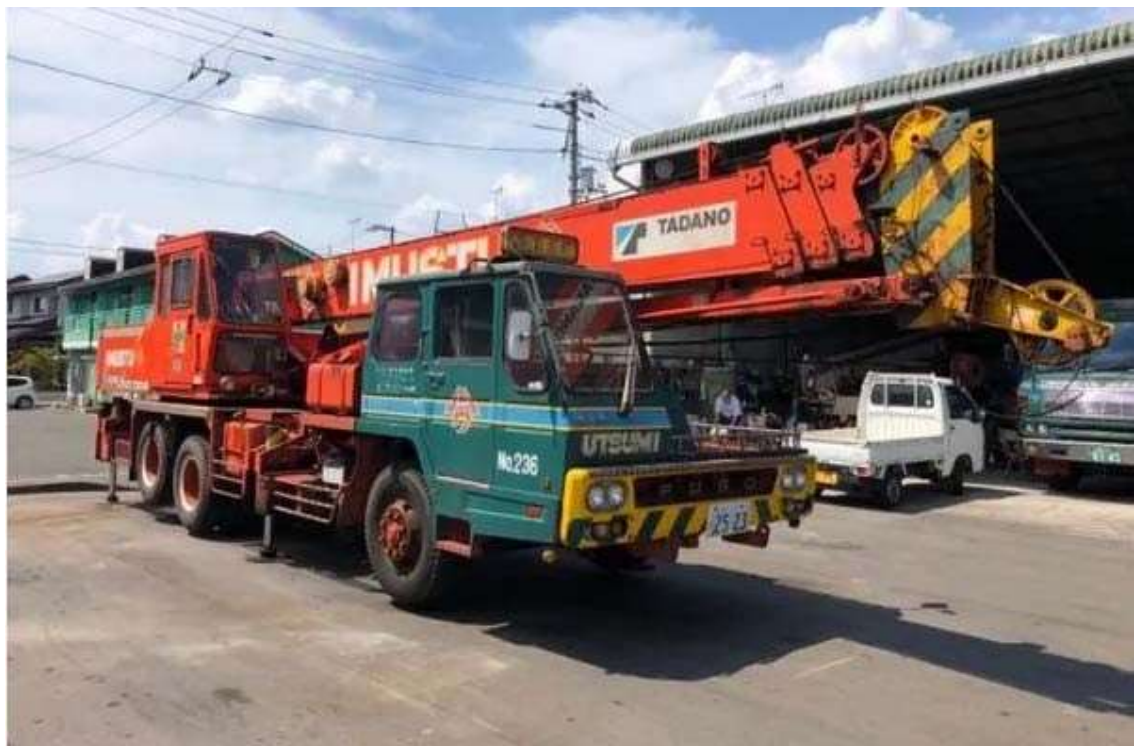
Figure 16: 25-ton crane to assemble piling machine
