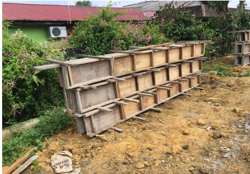
Figure 3.4.6 : Formwork for pad footing
