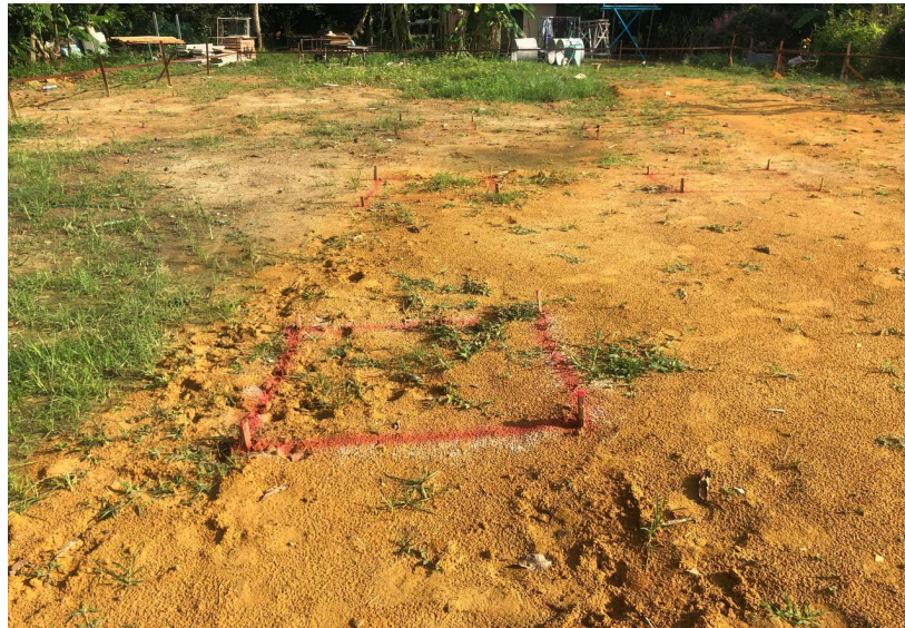
Figure 3.4.8 : Setting out point
