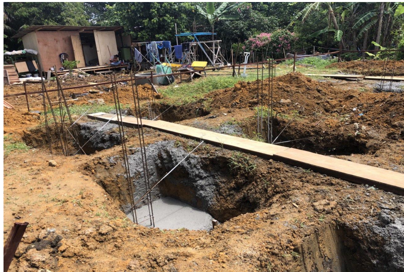
Figure 3.4.13 : Concreting work
