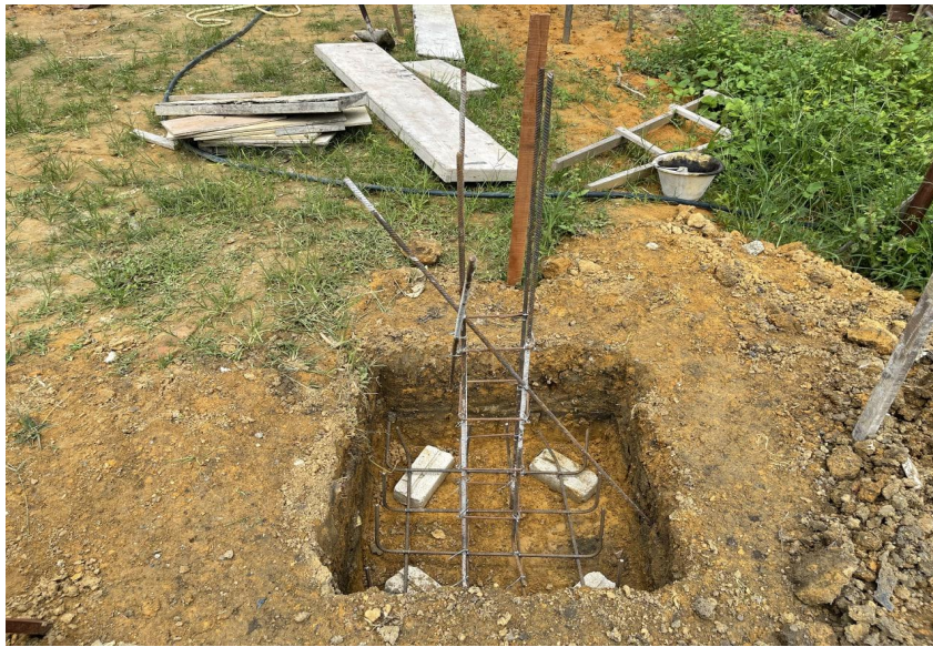
Figure 3.4.12 : Reinforcement bar installation
