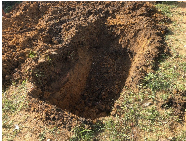
Figure 3.4.10: Footing hole
