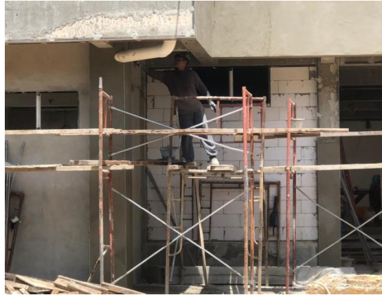
Figure 3.2.4 Put finishing coat to the top of surface
