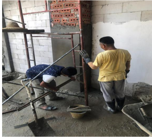
Figure 3.2.2 Checking for the thickness of plastering by looking to plumb-bob
