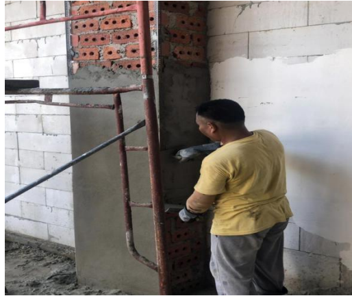
Figure 3.2.3 A trowel is using to put the first layer of plaster
