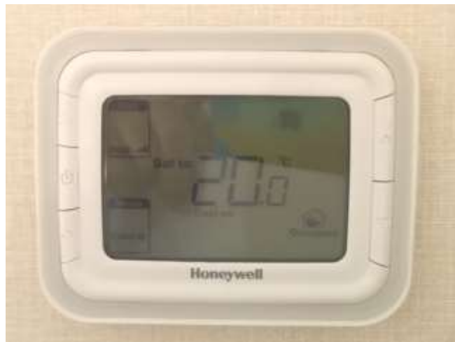
Figure 3.17 : Air conditioner thermostat
