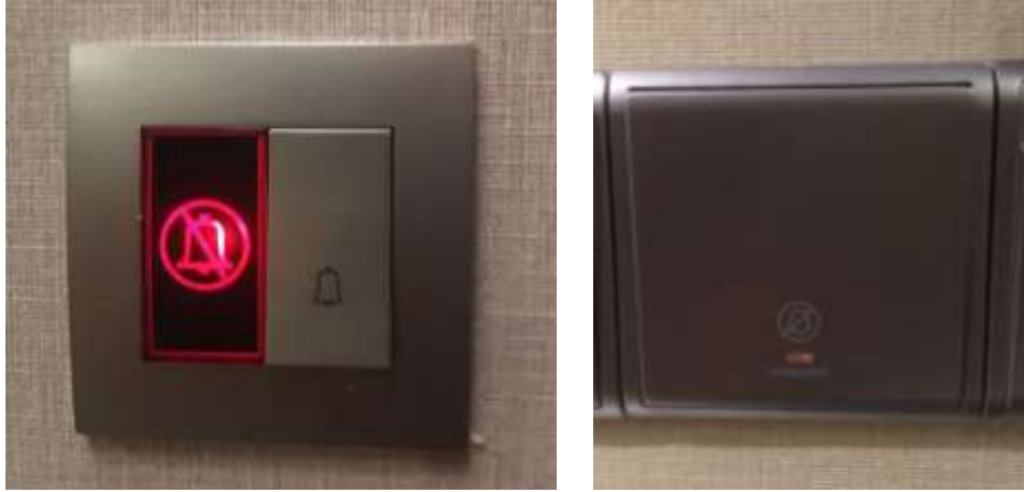
Figure 3.10 : Do not disturb interlock
