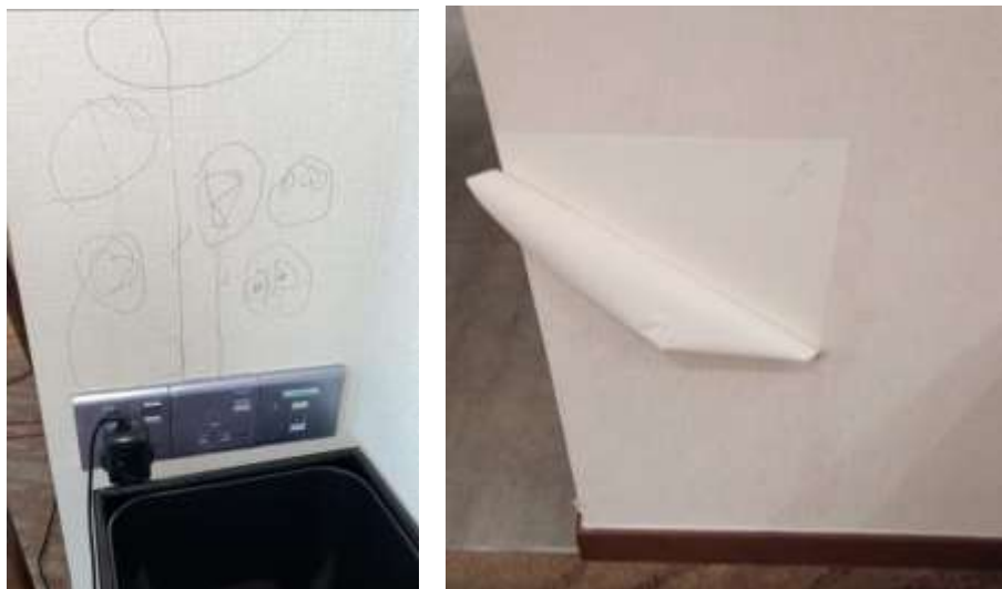
Figure 3.54 : Wallpaper defect
