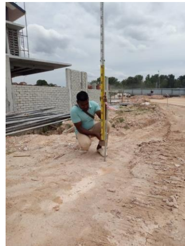
Figure 10: Surveyor used dumpy level to marking construction level.
