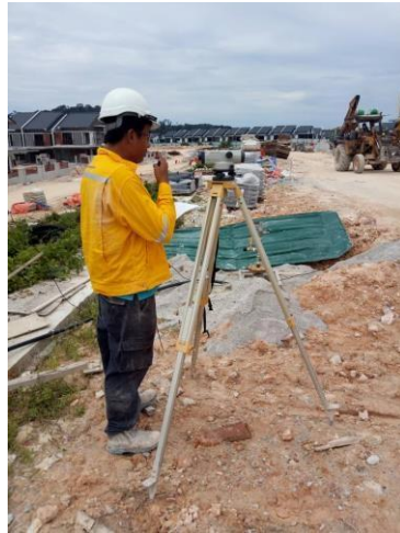
Figure 10: Surveyor used dumpy level to marking construction level.
