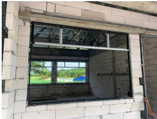
Photo 3.2.9: Opening part of windows and doors
