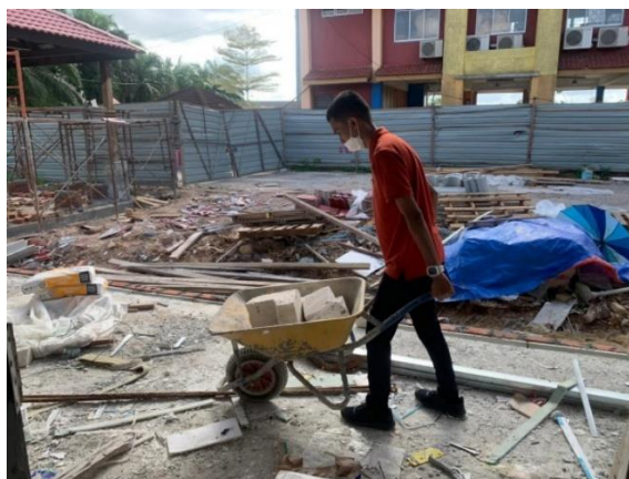
Photo 3.2.3: The brick was lifted by the workers using wheelbarrow
