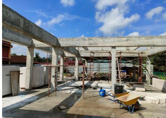
Photo 3.2.1: Building Site Construction.
