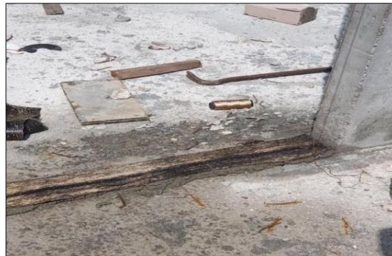
Photo 3.2.7: Pasting the Damp Proof Course (DPC) on the Bitumen
