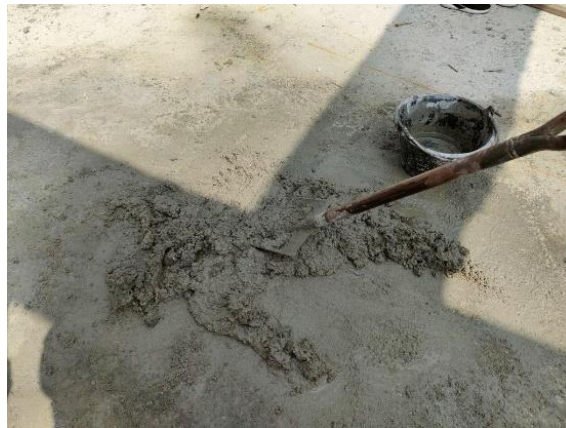
Photo 3.2.4: Mortar are mixed using the shovel
