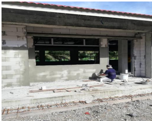
Photo 3.2.11: Plastering Work
