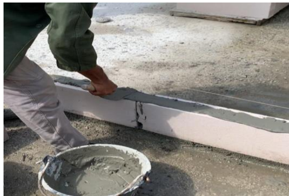
Photo 3.2.8: Starthen cement on the first brick
