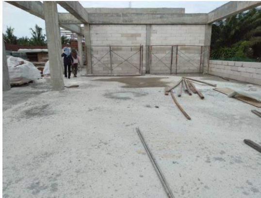
Photo 3.2.2 : The floor of building that have been cleaned before bricklaying process.
