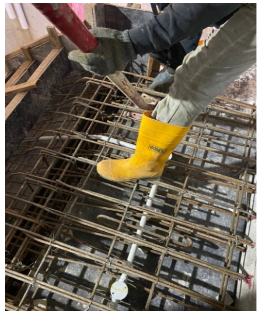
Figure 9: M&E Item Installation
