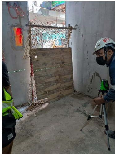
Figure 17: Inspection Staircase Level
