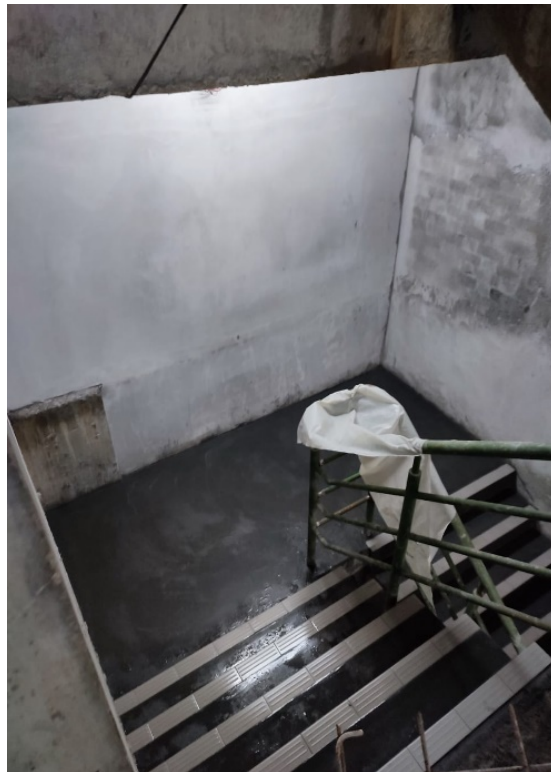
Figure 15: Screeding work And Curing Compound
