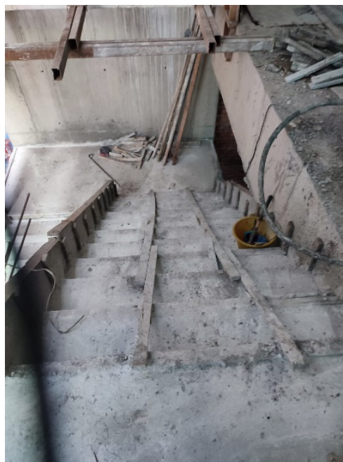
Figure 11: Casted Concrete Formwork
