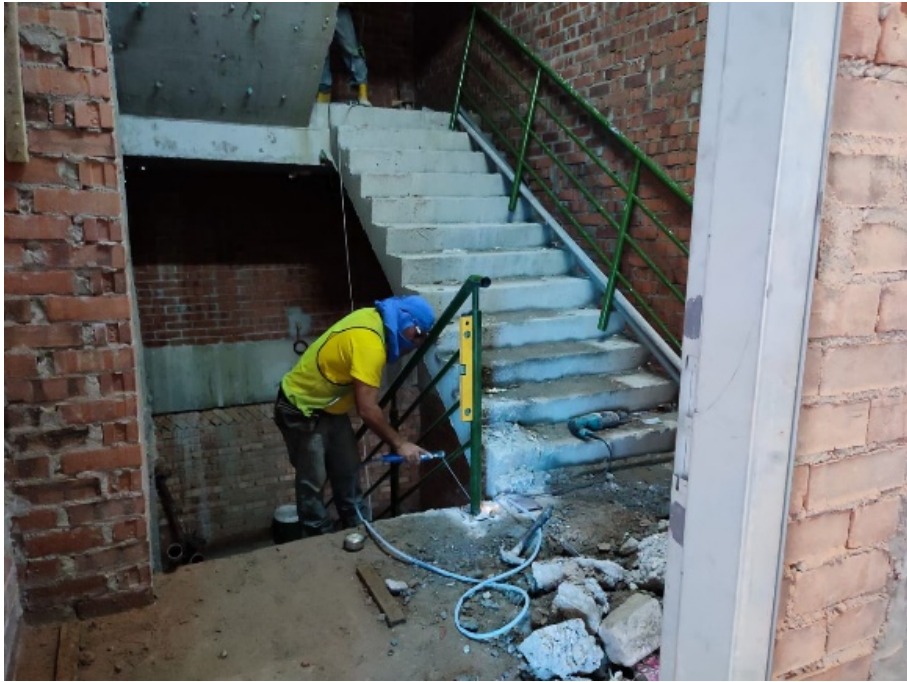
Figure 16: Railing Installation
