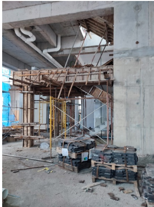
Figure 7: Formwork Installation
