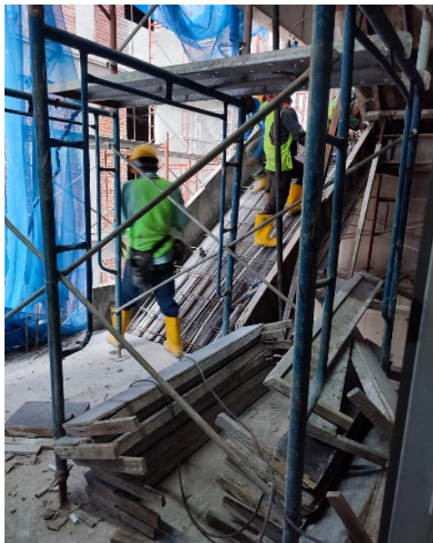
Figure 8: Rebar Installation
