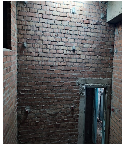
Figure 14: Level Peg Work
