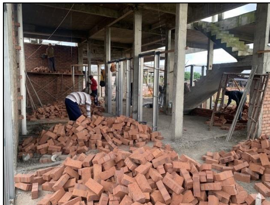
Figure 15: Install door frame before brickwork start
