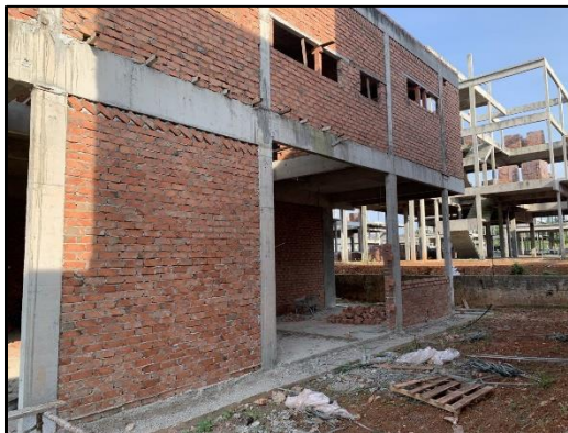
Figure 33: Completed wall surface after bricklaying work
