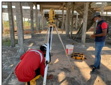
Figure 13: Setting out for bricklaying work
