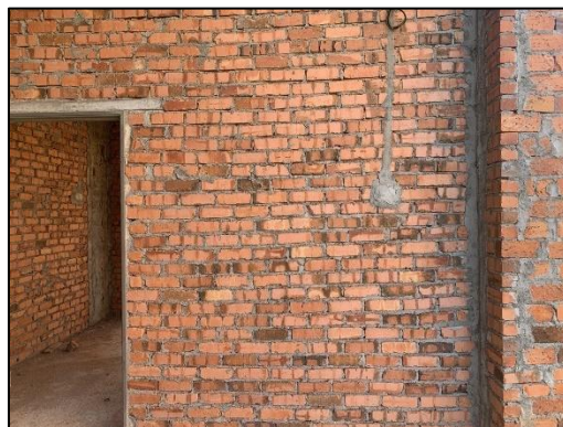
Figure 28: Stretcher bond
