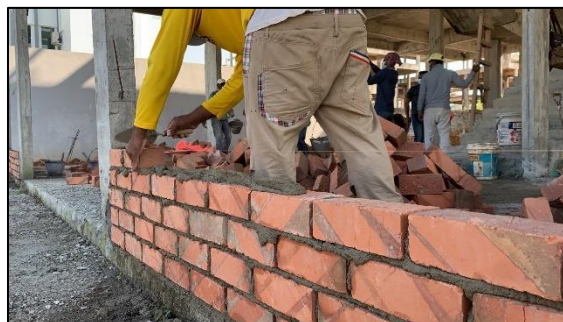
Figure 23: Move string line to for the next row
