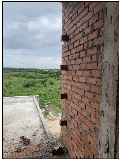
Figure 30: T-joint
