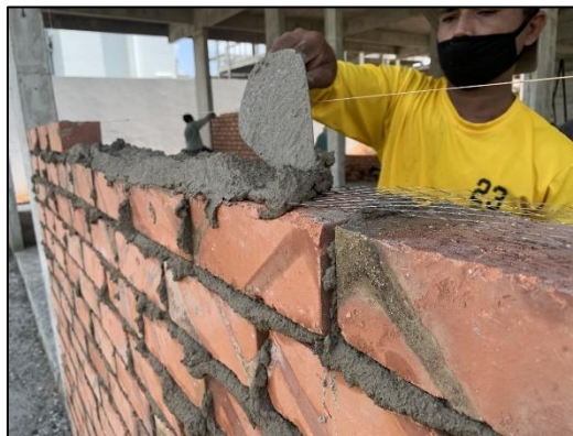
Figure 26: Exmet wire applied in every fourth
