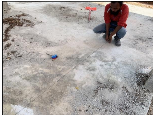
Figure 14: String marker used to make a reference line
