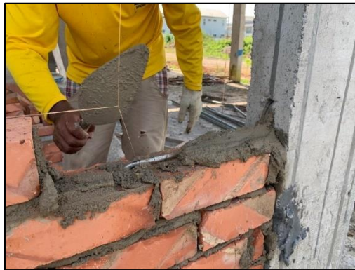
Figure 39: Mortar for bricklaying work
