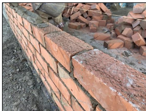
Figure 40: Exmet wire laid on fourth layer
