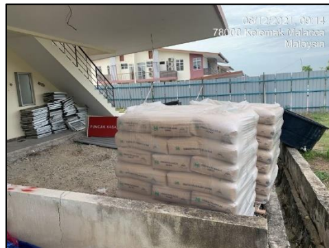
Figure 38: Couple pallets of cement
