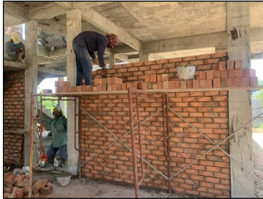
Figure 27: Scaffolding used to help bricklayer reach top height
