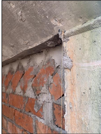
Figure 41: Pins and line
