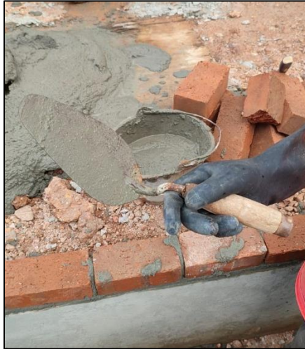
Figure 43: Bricklaying trowel
