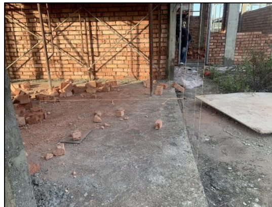
Figure 42: Pins and line on interior corner of brick line
