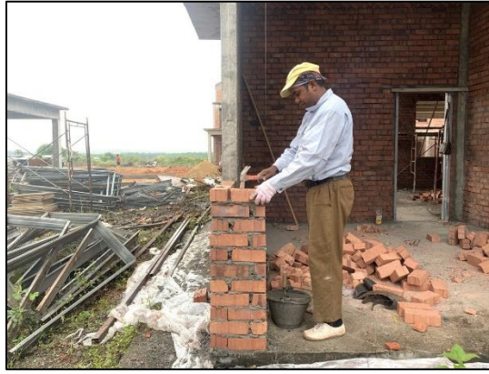
Figure 29: Brickwork corner
