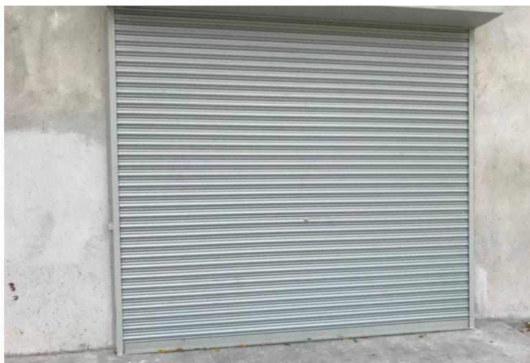
*Figure 3.6 Roller shutter has been installed*
