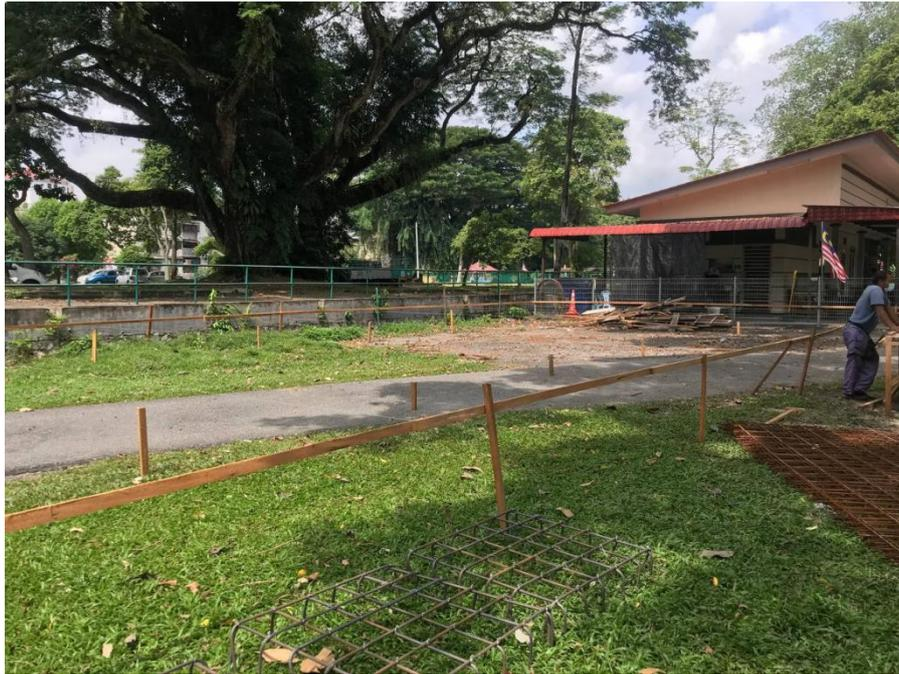
*Figure 3.1 Contractor marks the area to be excavate*
