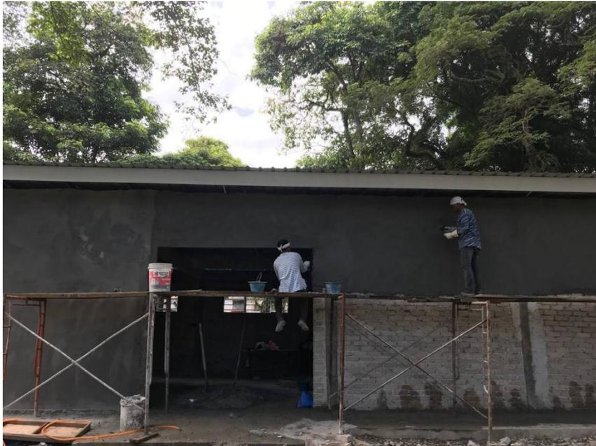
*Figure 3.5 The contractor plaster the wall*
