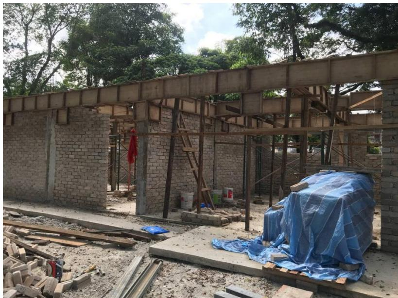
*Figure 3.4 Beam has been installed*
