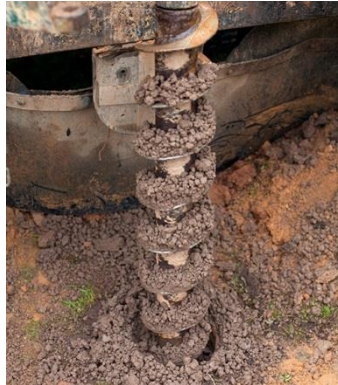
Figure 3.6: Pre-Bore works (Source: Internet)
