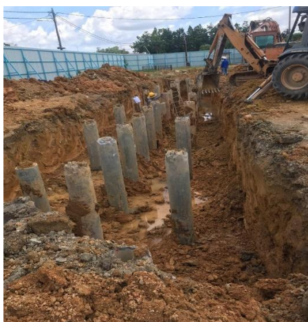
Figure 3.8: Excavation for pile cap
