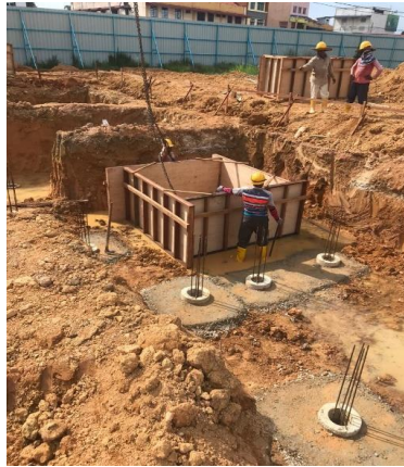
Figure 4.2: General Working installing Formwork
