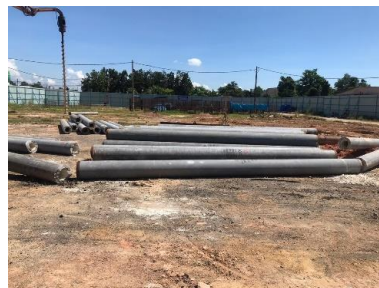
Figure 3.2: Extension Pile
