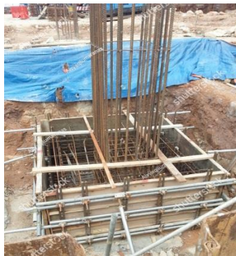
Figure 4.3: Rear in the pile cap formwork
