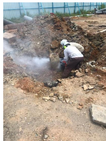
Figure 3.9: Pile Cut-off
