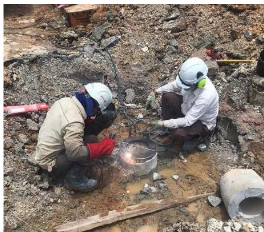
Figure 3.7 Mild Steel Welding
