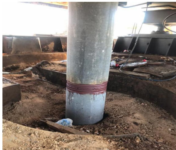
Figure 3.5: Connection between two piles
