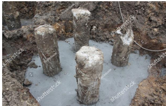
Figure 4.1: Example of lean Concrete (source: Internet)
