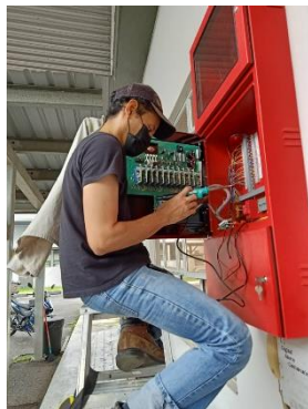
Figure 16: Technician repairing diode and checking electric current
