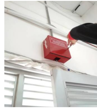
Figure 21: Inspecting fire curtain box
