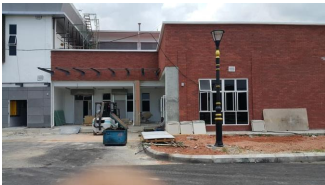
Figure 3: The view right side of Klinik Kesihatan Muar
