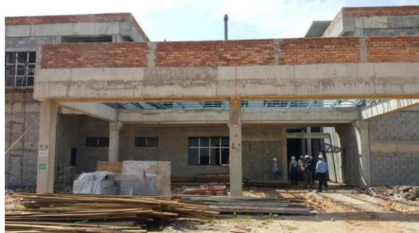
Figure 2: The view left side of Klinik Kesihatan Muar
