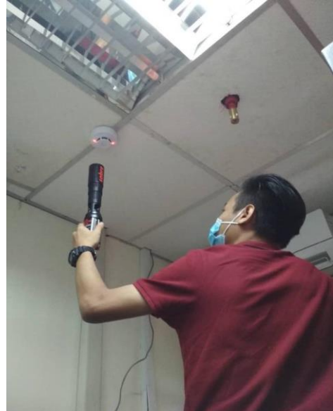
Figure 6: Inspecting smoke detector
