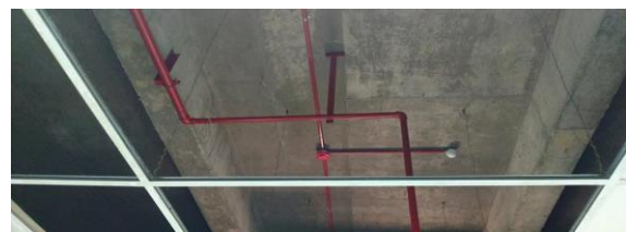
Figure 7: Smoke detector location
