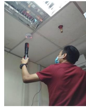
Figure 18: Checking rate of rise smoke detector
