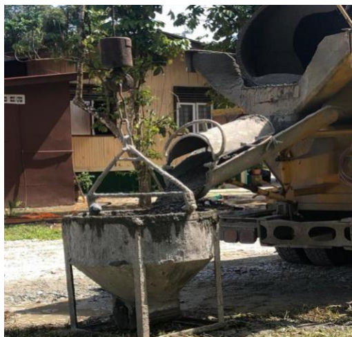
Figure 7.0 : Ready mix concrete
