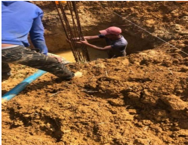
Figure 6.0 : Positioning reinforcement of footing and stump
