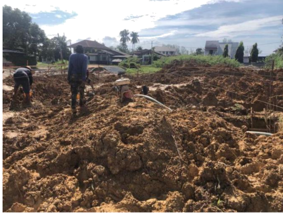
Figure 5.0 : Excavation of foundation
