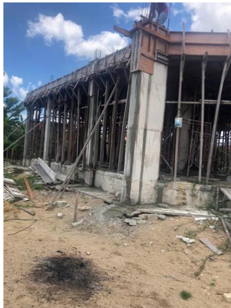
Figure 10.0 : Concreting and formwork for slab
