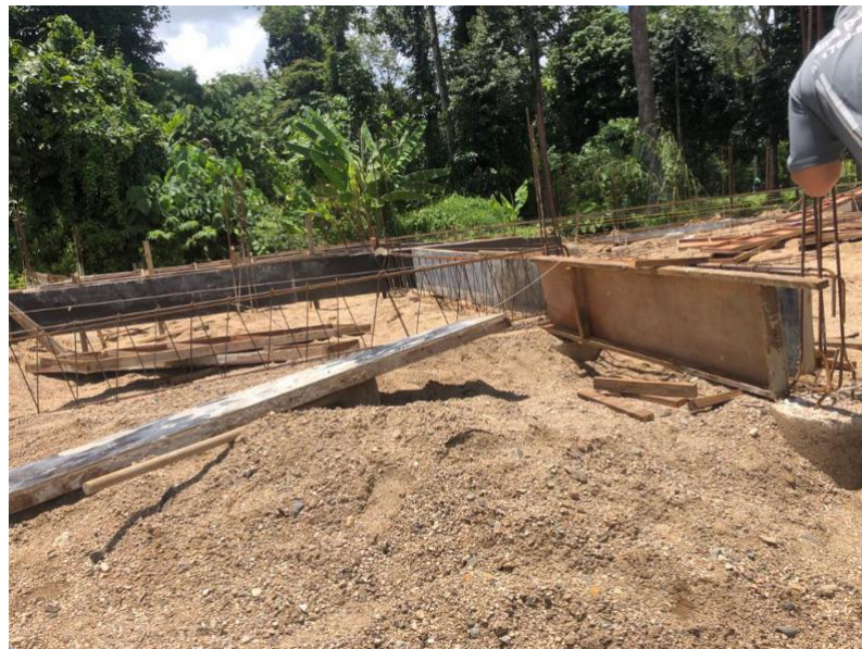
Figure 8.0 : Beam formwork and concreting
