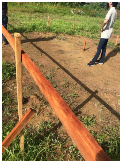
Figure 4.0 : Making the foundation position
