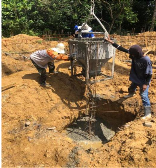
Figure 7.0 : Concreting and footing
