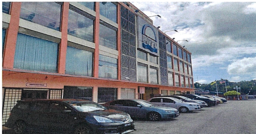
Building of Majlis Perbandaran Port Dickson (Block C)
