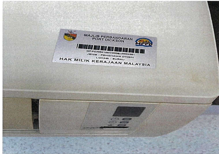
Sticker on the asset contained details or location, type of asset and number of registered.
