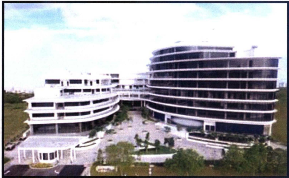
Figure 1.4: New building CUCMS at Persiaran Bestari
