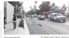
Safe separation of pedestrian vs vehicles
