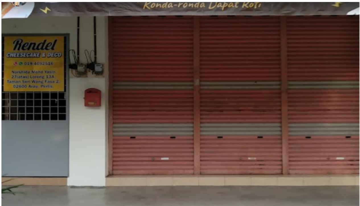
Figure 4: Rendel Cheesecake & Deco shop stairs beside Roti Ronda Shop
