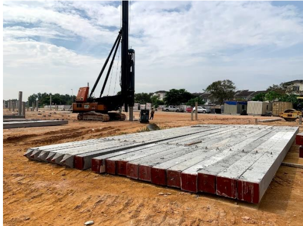
Figure 3.1 Reinforced Concrete Piles
