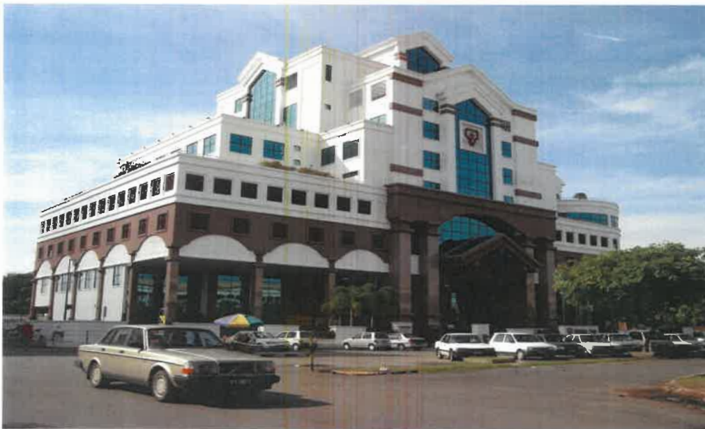
Figure 1: Tenaga Nasional Berhad Alor Setar Building
