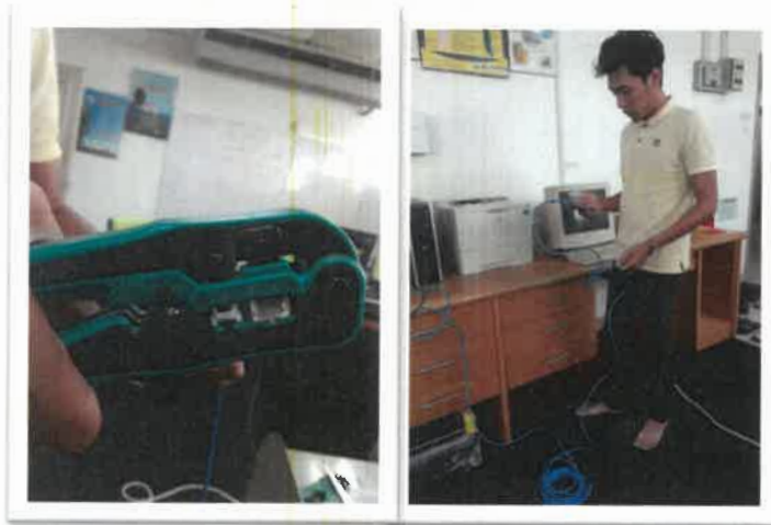
Figure 24: Network cable crimping
