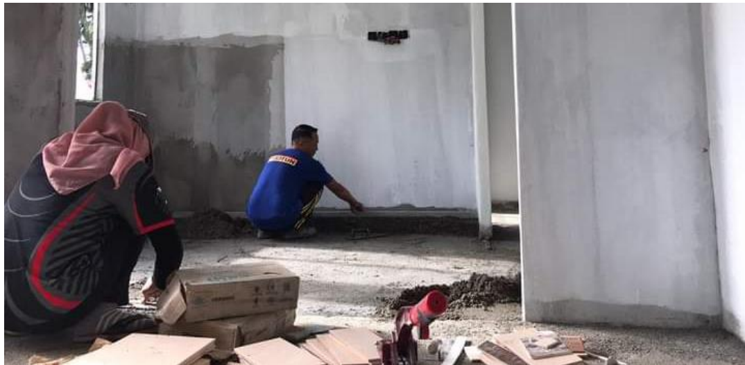
Figure 3.3 Installation of a cement board underlayment
