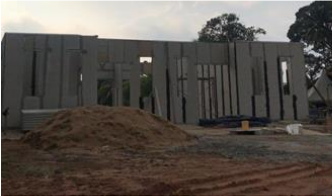
Figure 3.2 picture of worksite at Bukit Tembakau
