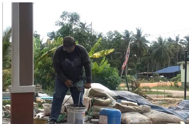
Figure 3.5 The process of making thin-set mortar
