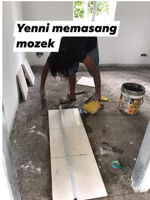
Figure 3.4 One of the worker install tile
