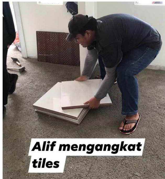
Figure 3.18 Example of bad handling tile
