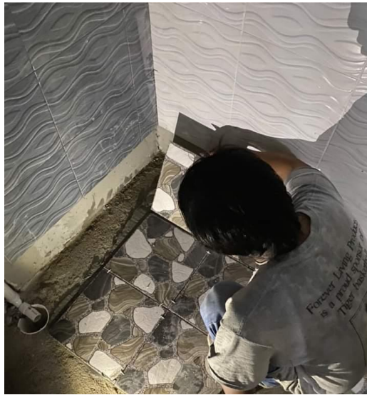
Figure 3.9 A worker installing tile in bathroom floor
