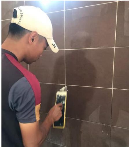
Figure 3.7 Process of installing the grout
