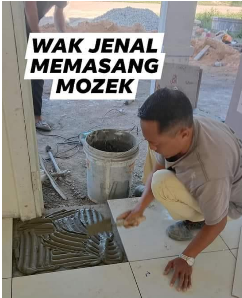
Figure 3.6 One of the worker reinstall a tile with a thicker glue
