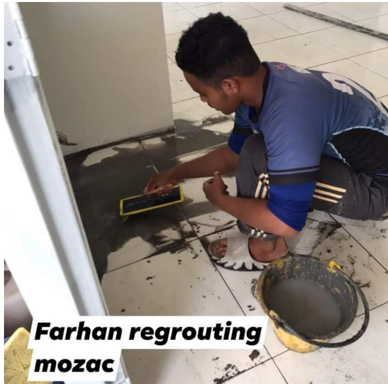
Figure 3.16 Process of refill under the tile using molten state mortar
