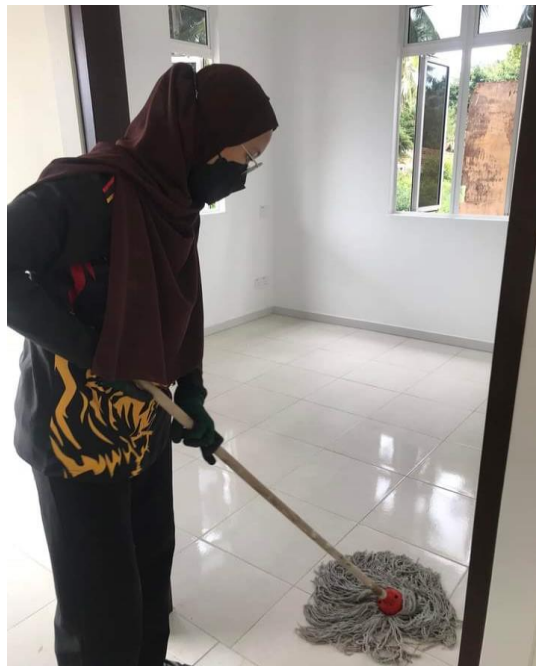
Figure 3.8 Process of washing some leftover grout
