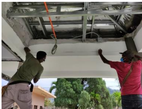
Figure 3.3.4(1) Worker are marking before installing frame
