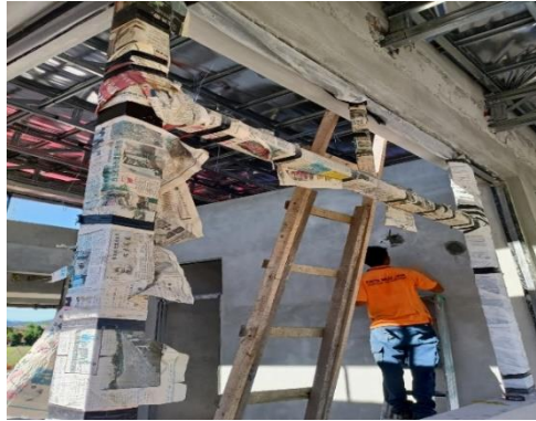
Figure 3.3.1(1) Worker doing an electrical wiring work inside guard house
