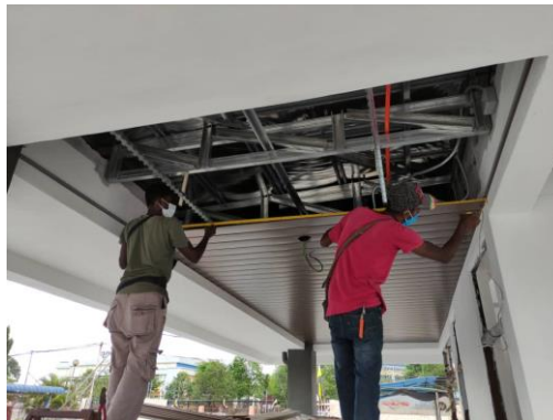
Figure 3.3.7(1) Worker installing the aluminium strip panel
