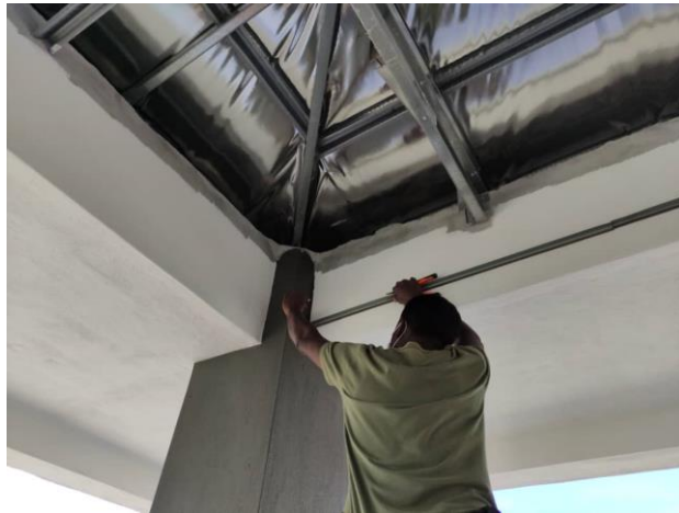
Figure 3.3.5 Worker installing frame
