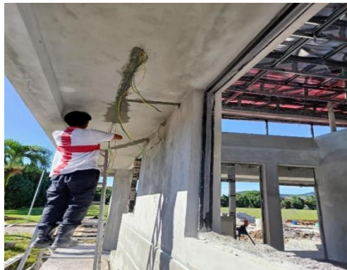
Figure 3.3.1(2) Worker doing an electrical wiring work outside guard house
