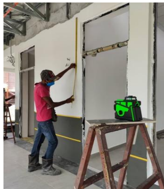
Figure 3.3.3(2) Worker measuring the height to mark for installation of ceiling
