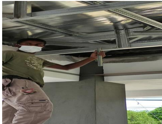
Figure 3.3.6(1) Worker install hanger to hold the main keel later.
