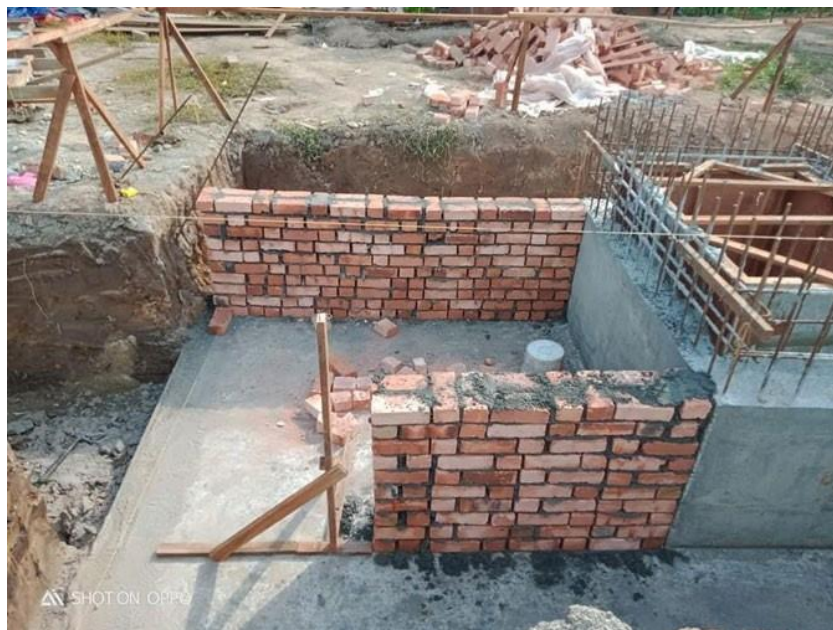
Figure 3.18: Construct brickwall
