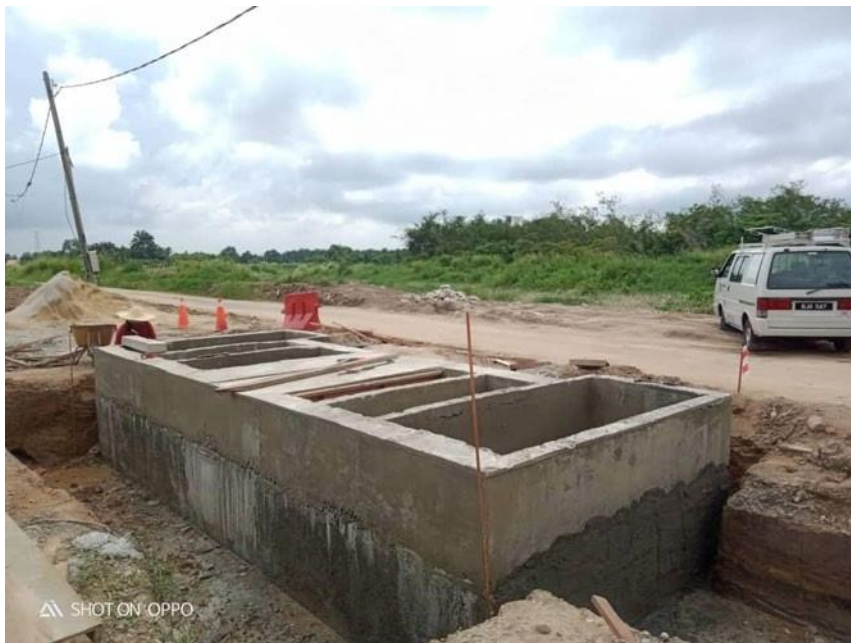
Figure 3.23: After the formwork for upper beam and slab were removed
