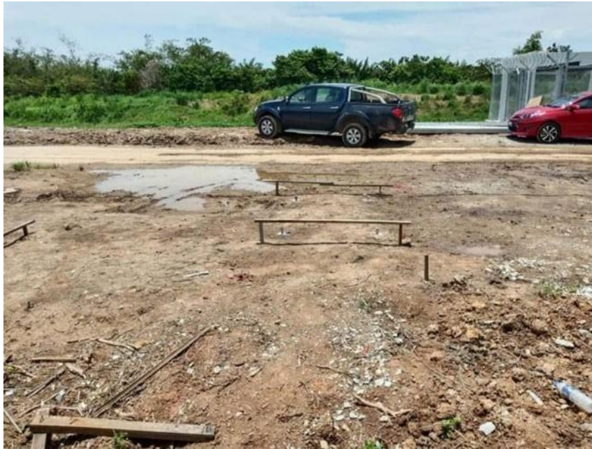
Figure 3.9: Marking piling point
