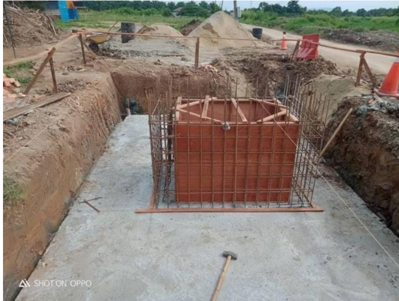
Figure 3.15: Concrete fully dried for foundation of compact substation
