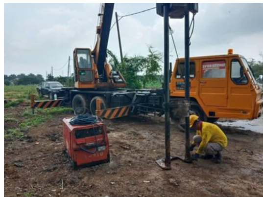
Figure 3.6: Hammer for piling
