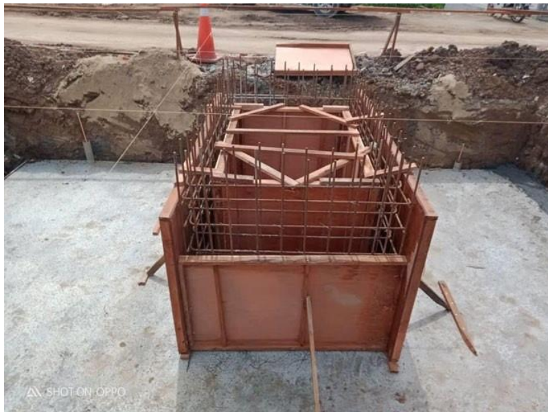
Figure 3.16: Formwork for conc trench
