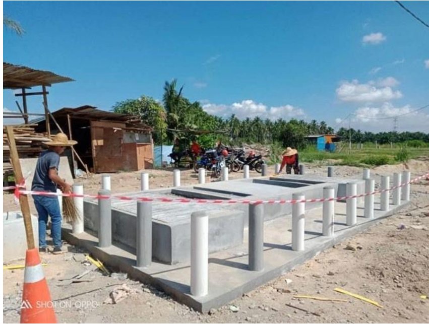
Figure 3.33: Plastering work complete
