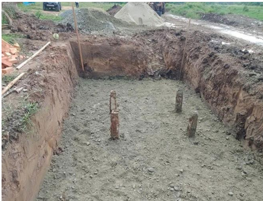
Figure 3.12: The condition of lean concrete at the evening.
