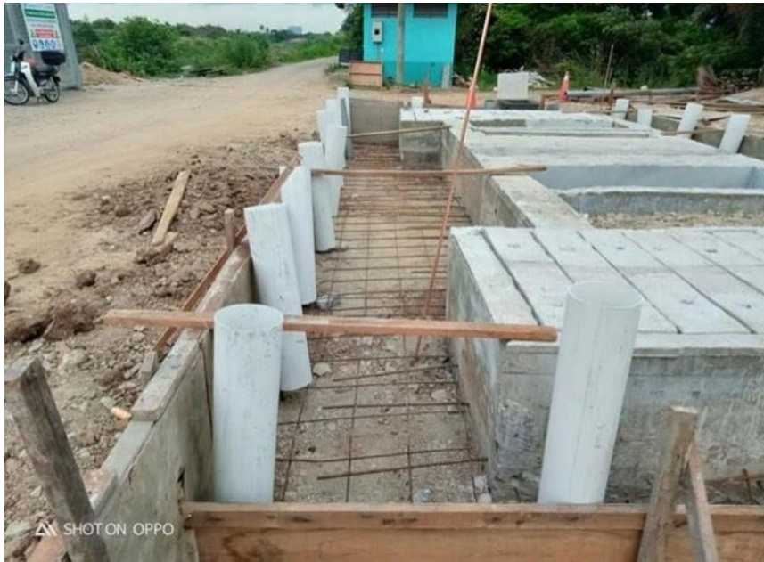
Figure 3.30: Installation rebar for apron
