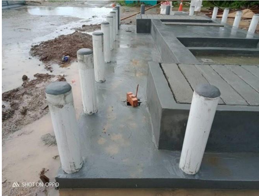
Figure 3.31: Process preparing apron and bollard were completed
