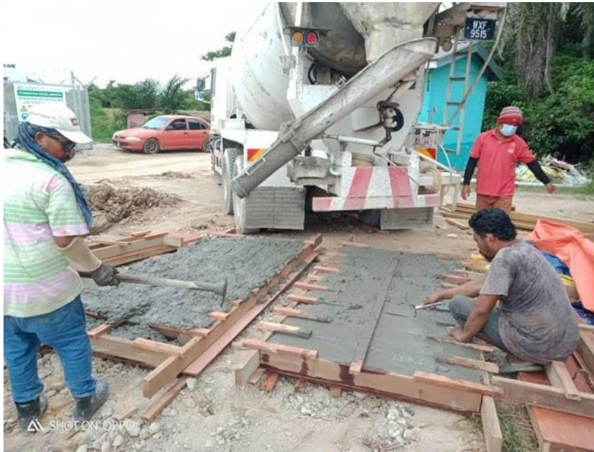
Figure 3.22: Poured concrete on formwork of cover slab and let it dried
