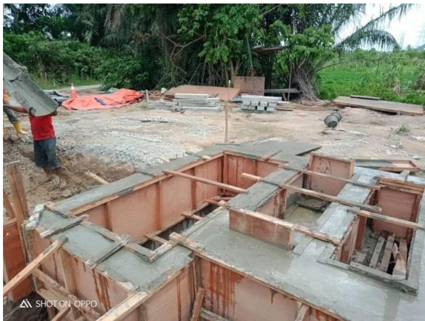
Figure 3.21: Formwork for upper beam and slab poured with concrete grade 25
