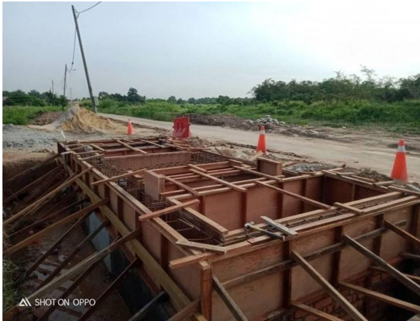
Figure 3.20: Formwork for upper beam and slab
