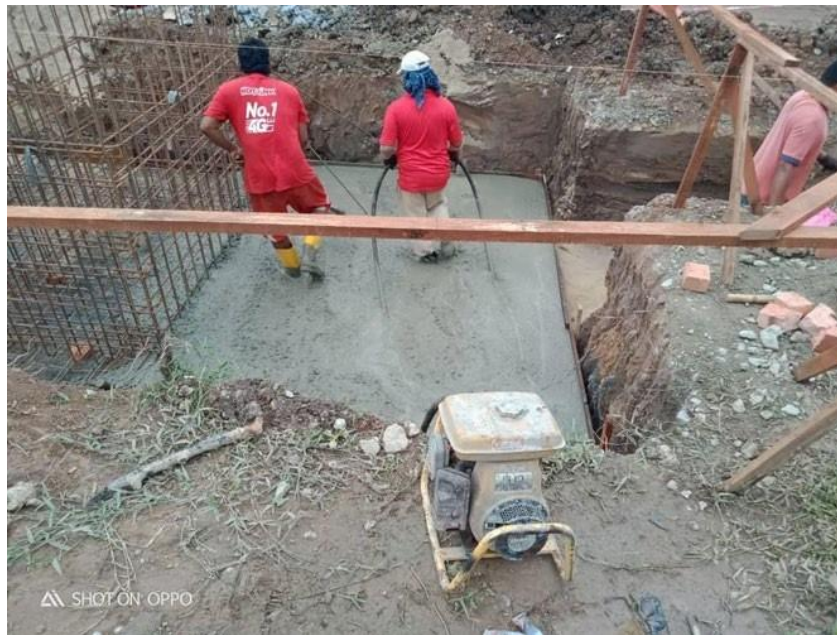
Figure 3.14: vibrator electric is use in pouring concrete to avoid honeycomb
