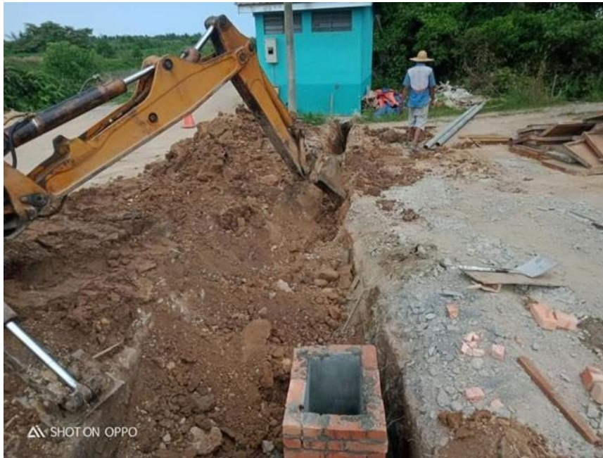
Figure 3.28: Excavation process before laying HDPE pipe
