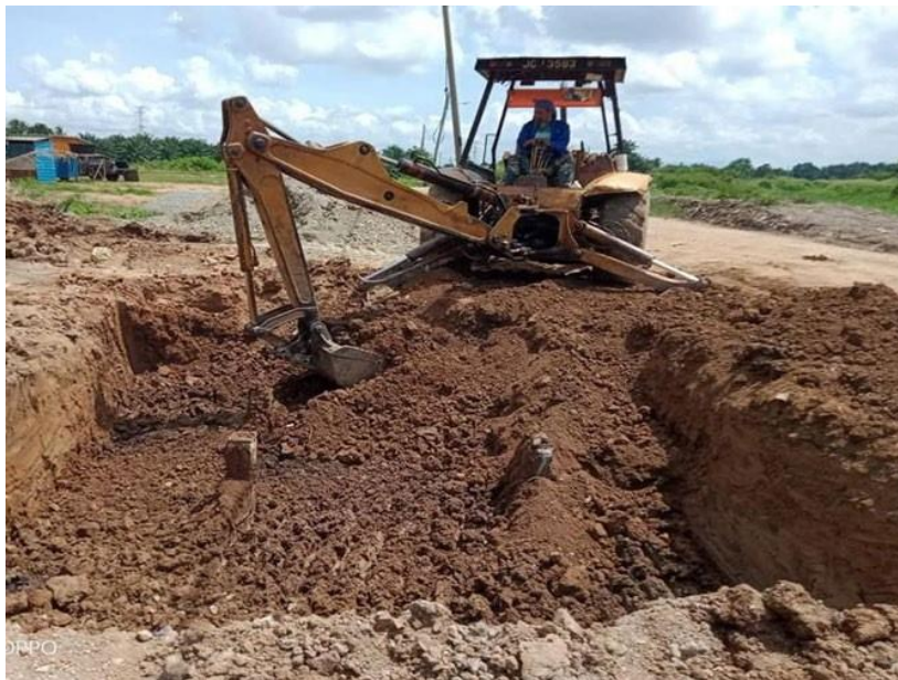
Figure 3.11: Excavate the area of compact sub after finish piling work
