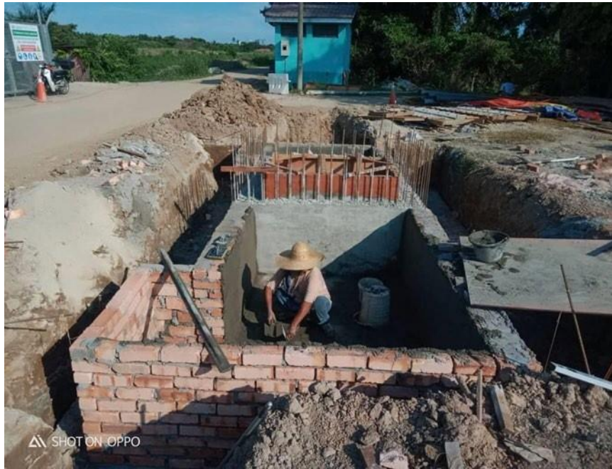
Figure 3.19: Plastering the brickwall
