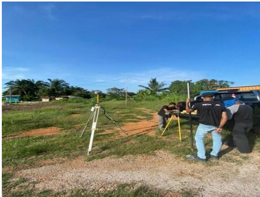
Figure 3.8: The workers setup the level machine at site
