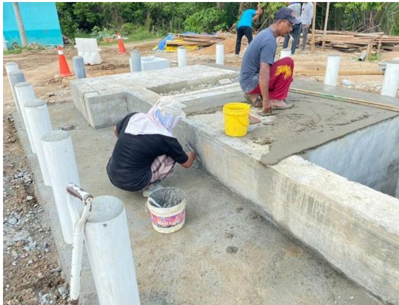
Figure 3.32: Progress of plastering work
