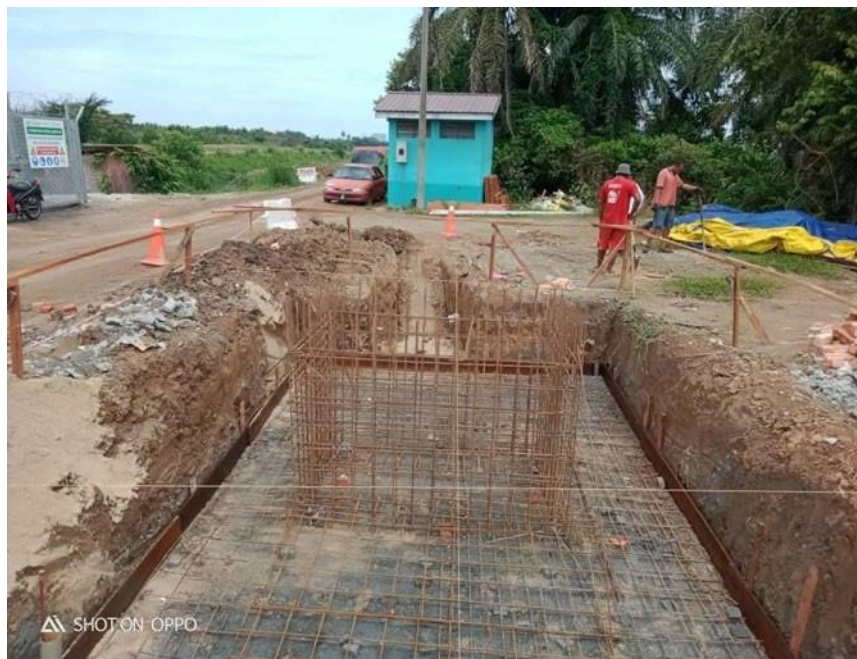
Figure 3.13: Installation rebar for foundation and conc trench process was completed
