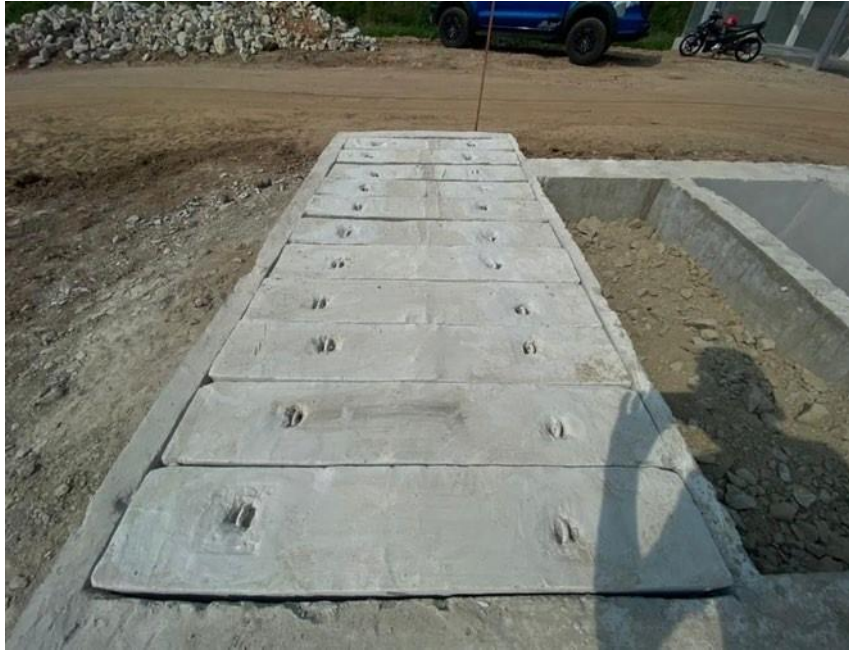
Figure 3.24: The cover installed to compact substation
