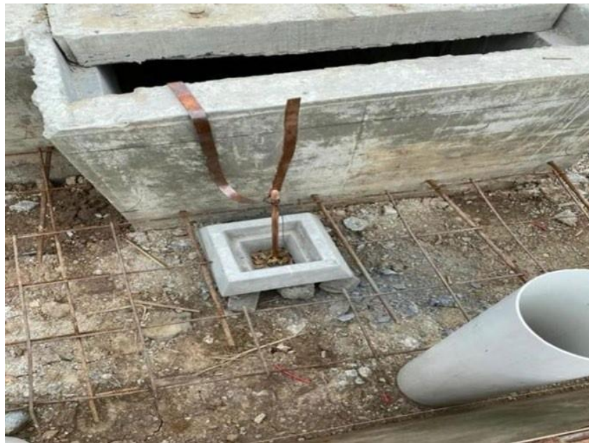
Figure 3.26: Complete install the copper road outside compact substation
