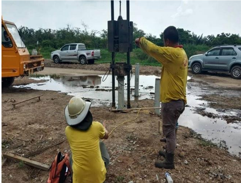
Figure 3.10: The span pile was driving with hammer help.
