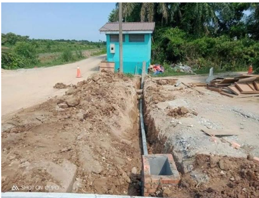
Figure 3.29: Installation the pipe as cable protection complete
