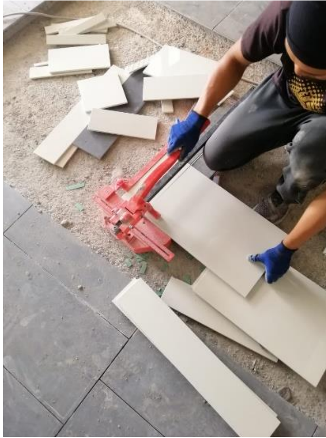
Figure 3.2.3 cutting the tile using tile cutter
