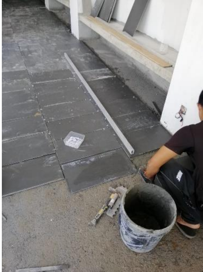
Figure 3.2.4 The tiles laid on the floor
