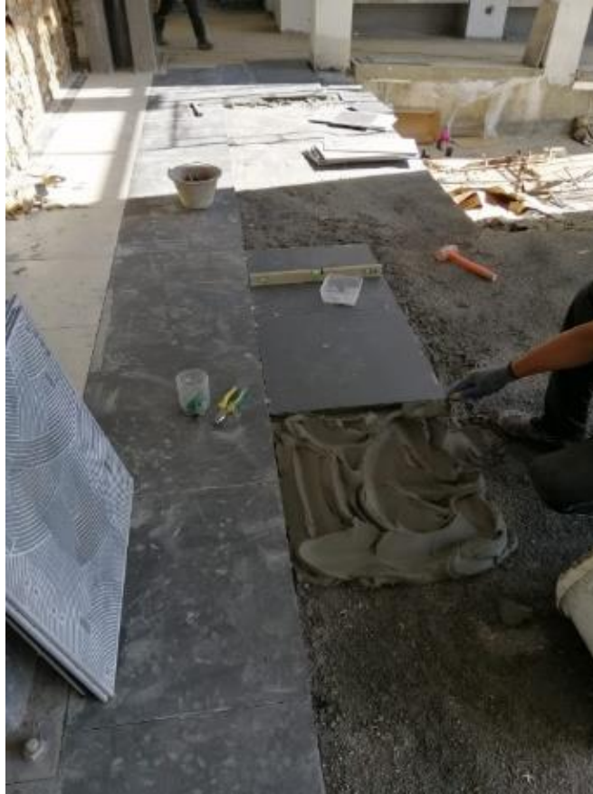
Figure 3.2.2 Lay cement gum before installing tile
