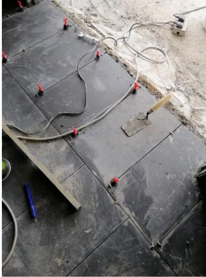
Figure 3.2.5 Install tile spacer and tile levelling system
