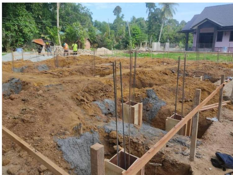
*Figure 3.7 Reinforced for Column*
