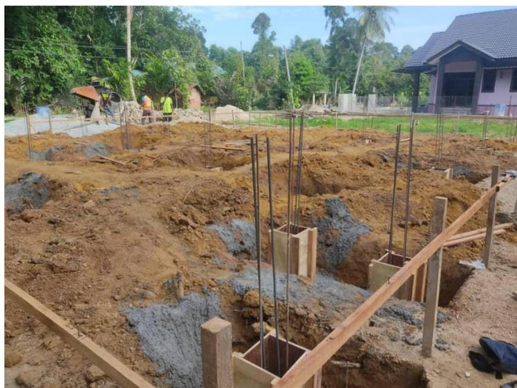
*Figure 3.7 Reinforced for Column*
