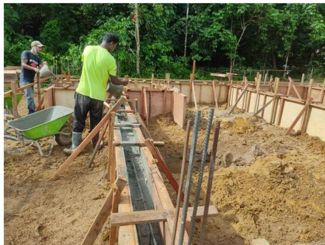
*Figure 3.4 Pouring the Concrete*
