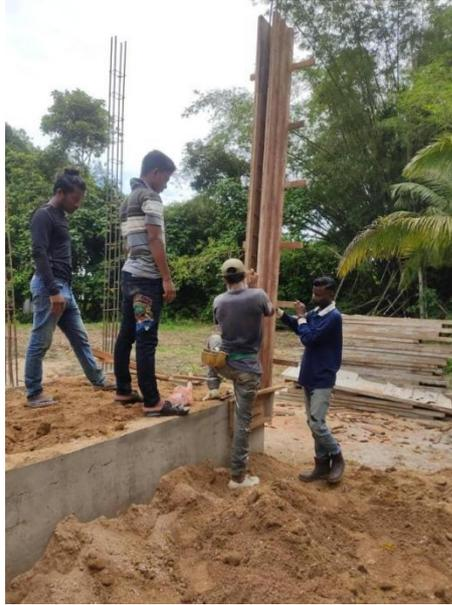
*Figure 3.8 Formwork for Column*
