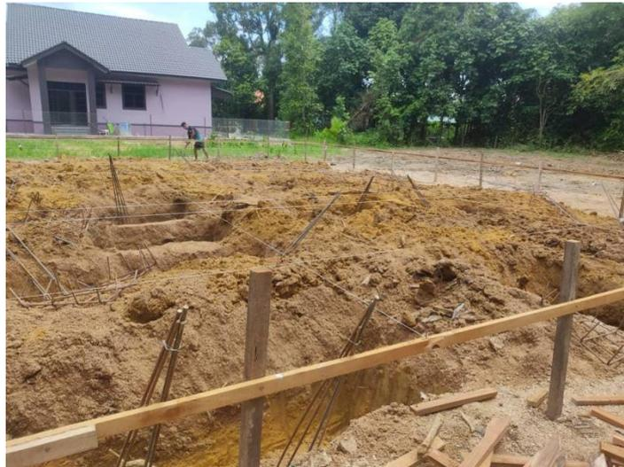
*Figure 3.6 Setting Out for Column*
