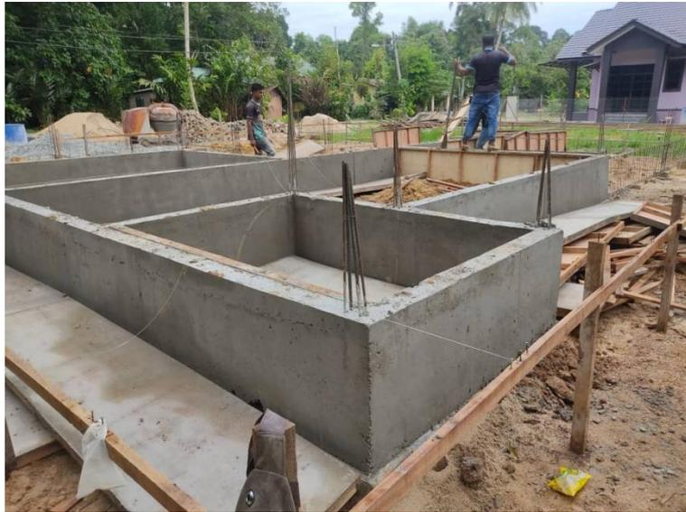
*Figure 3.5 Complete Ground Beam*
