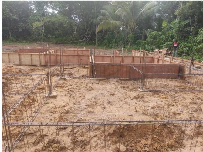
*Figure 3.3 Ground Beam Formwork*
