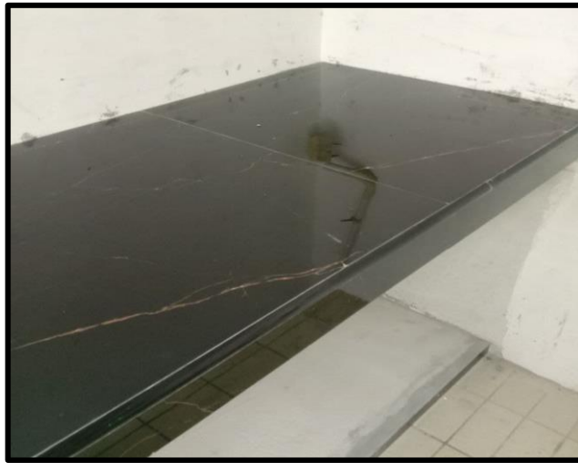
Figure 12: Tiles Finishes Work Had Been Done
