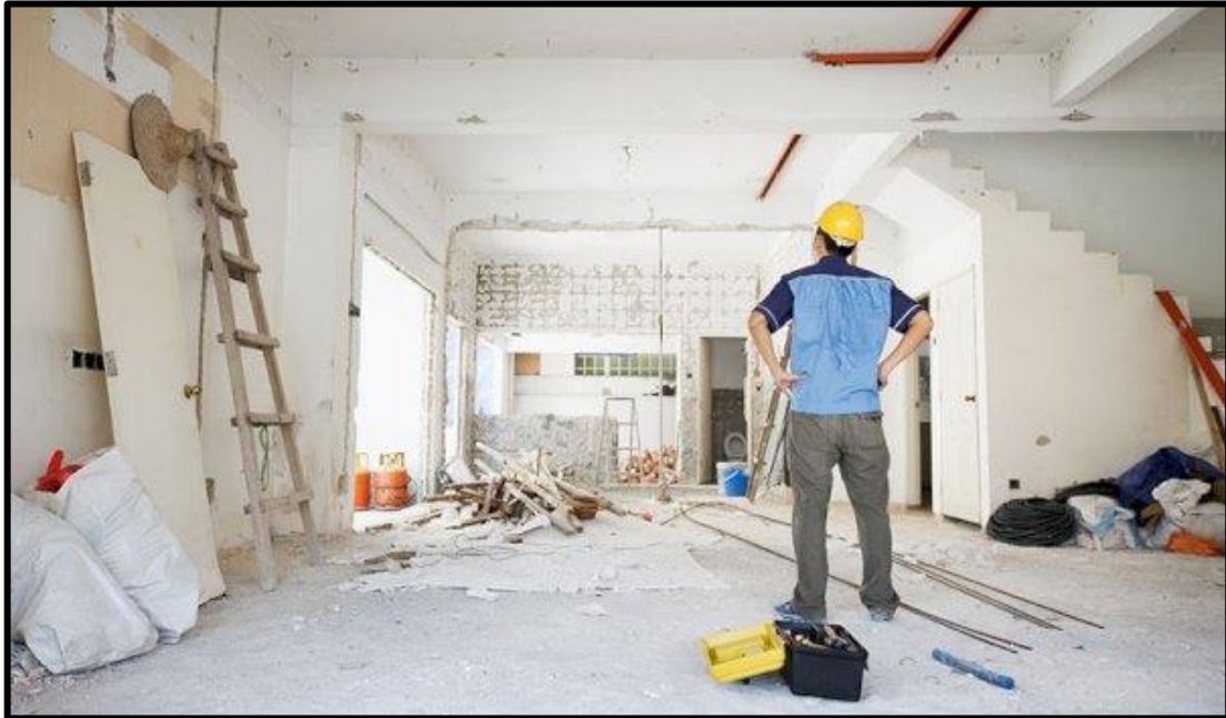
Figure 1: Example of Renovation Work
