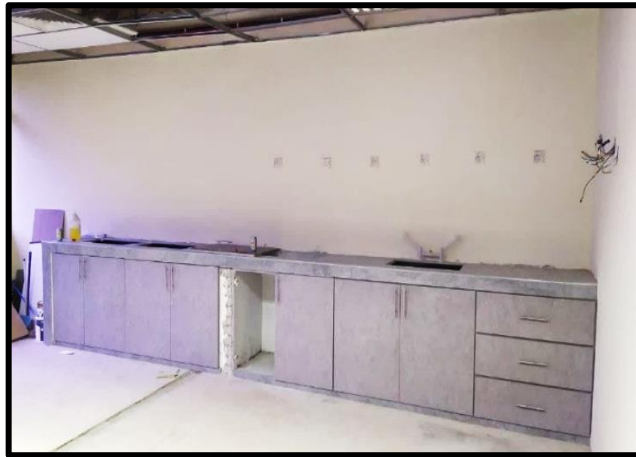
Figure 11: Example of Concrete Bench
