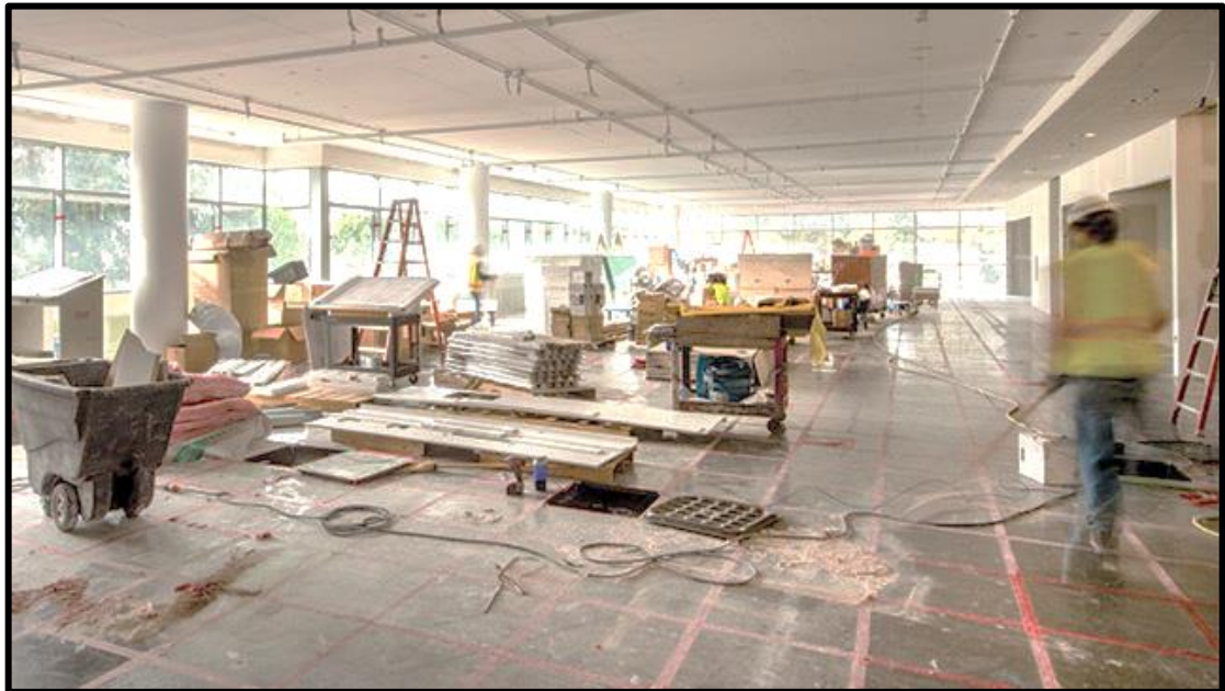
Figure 5: Example of Ongoing Renovation Project
