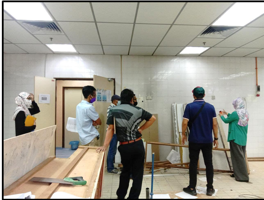
Figure 7: Site Inspection by main contractor, sub-contractor, and client
