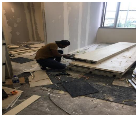
Figure 3.3.1: The workers cut the demountable partition
