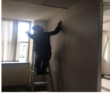
Figure 3.2.13: The installation of net at the gypsum board
