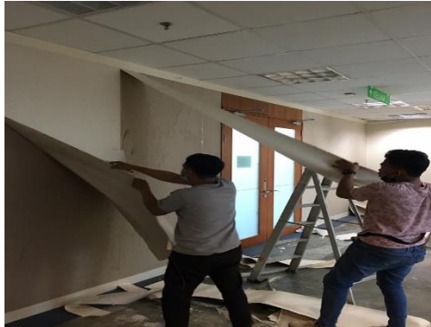
Figure 3.2.8: The wallpaper has been removing
