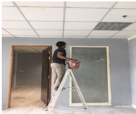
Figure 3.2.18: The second coating paint for the partition wall Source: Fadlhlin Engineering project document
