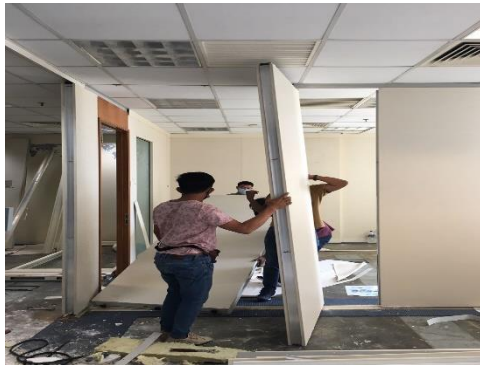
Figure 3.2.9: The workers dismantle the current partition.
