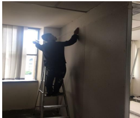
Figure 3.3.2: The installation of net at the gypsum board
