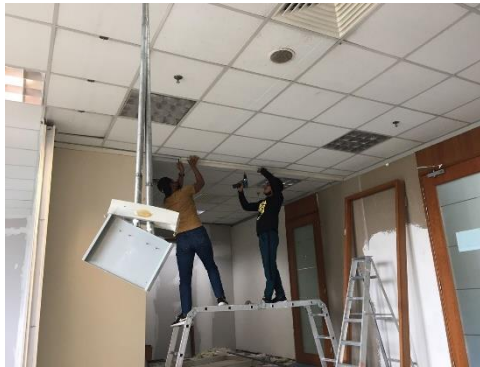
Figure 3.2.10: The installation of the partition
