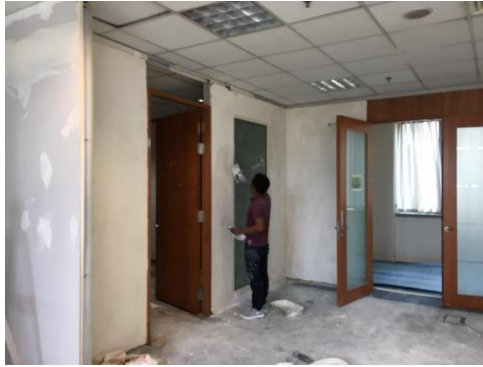
Figure 3.2.11: The workers do the skimming process
