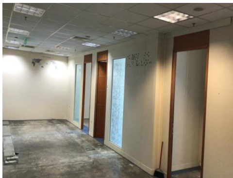
Figure 3.2.7: The room area that have been cleaned
