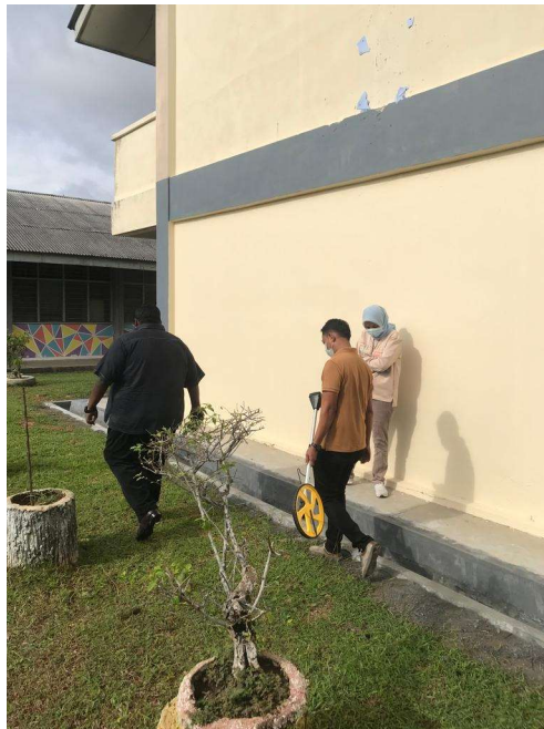
Figure 3.7: Preliminaries measurement for the drains using roller.
