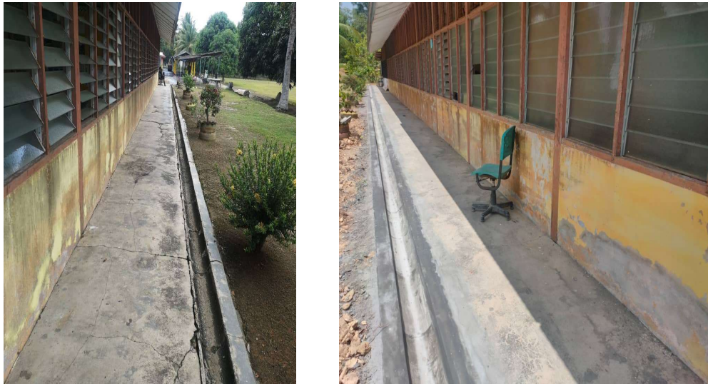
Figure 3.8: Before and after for drains installation
