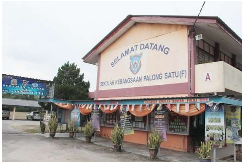
Figure 3.1 Construction site for building maintenance work source : Sekolah Kebangsaan Palong 1
