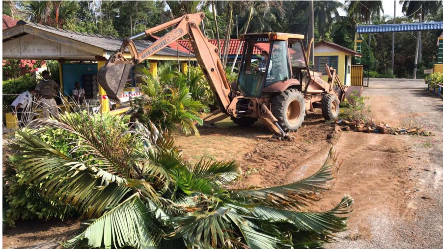
Figure 3.11: Clearance site for pavement work (premix)
