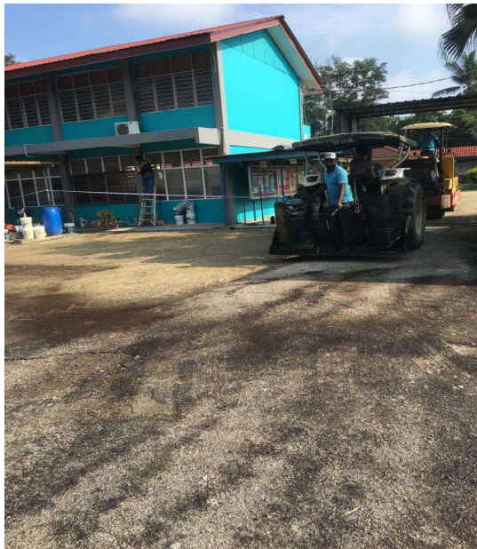
Figure 3.12: The workers spray the tack coat follow the specification.
