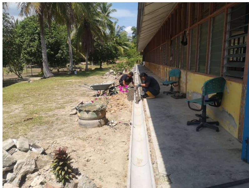
Figure 3.9: Checking and inspection size of drain following the specification.
