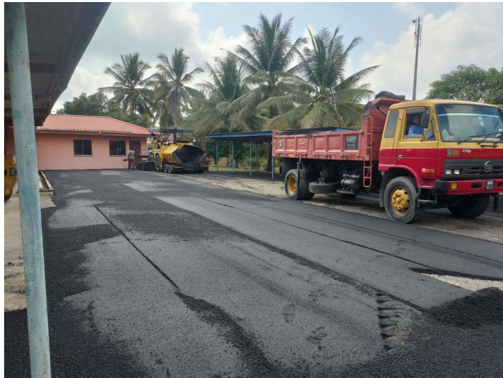
Figure 3.13: The paver hopper used to lay asphalt on roads
