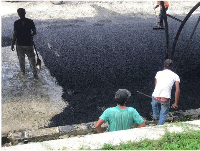
Figure 3.15: The workers spread the premix
