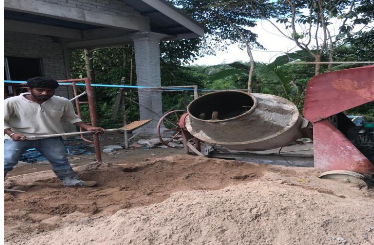
Figure 3.5: Mortar are mixed by hand using a shovel
