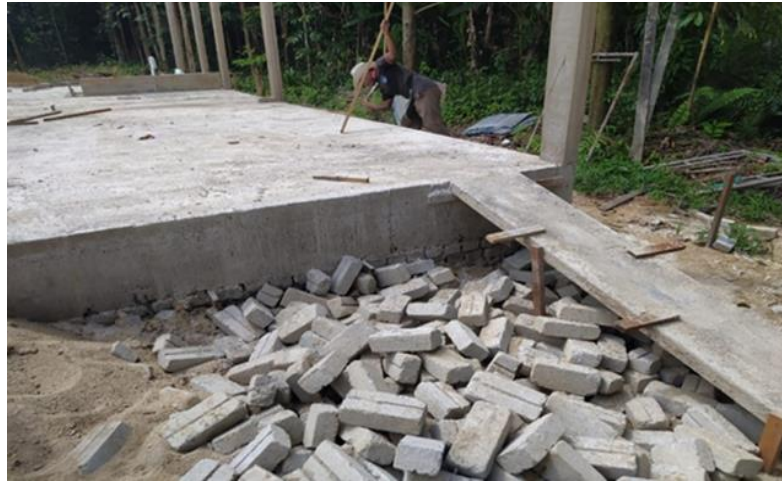
Figure 3.3: The floor of building that have been cleaned before bricklaying process.
