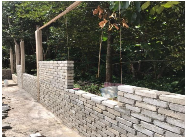
Figure 3.19: the bricklaying process for opening section
