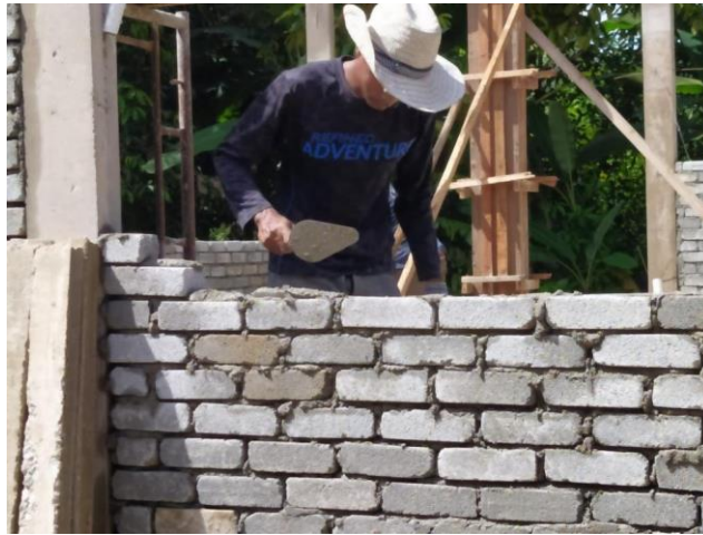
Figure 3.18: the bricklaying for 3 bedrooms area
