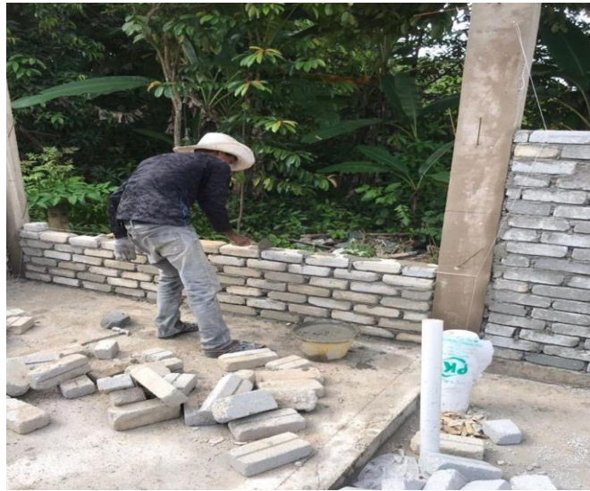
Figure 3.22: The Bricklaying process at bathroom area
