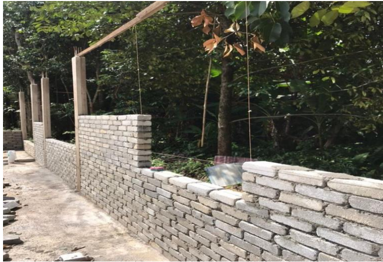
Figure 3.6: Strings that pinned together in between column.
