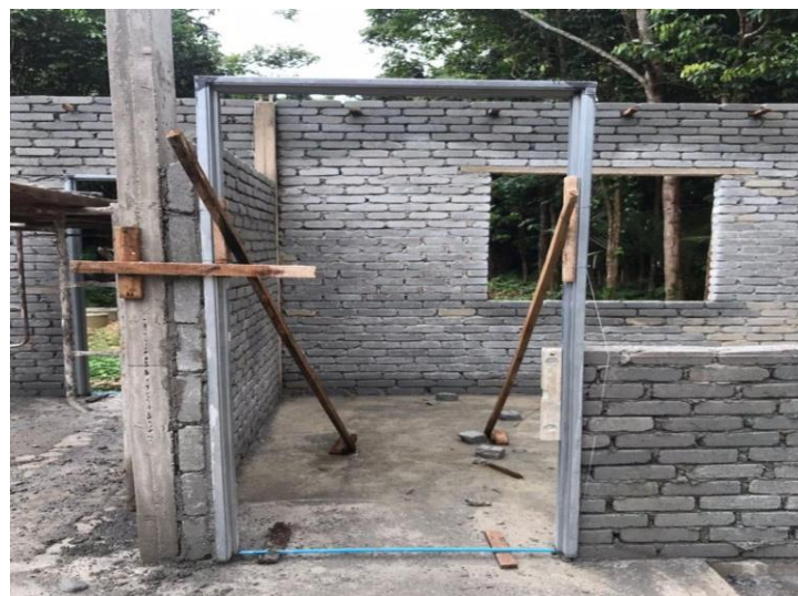
Figure 3.9: The door opening part of the wall.
