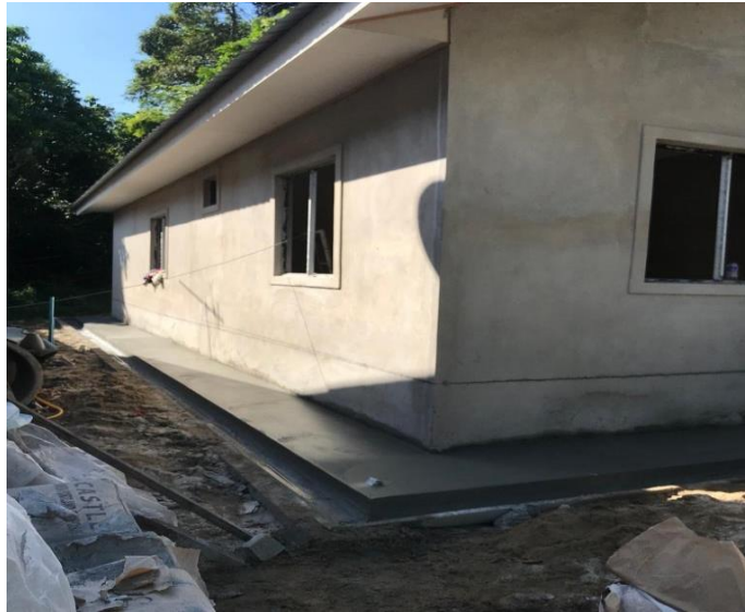
Figure 3.12: The wall after plastering process finish.
