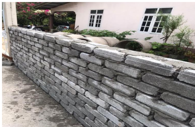
Figure 3.7: Bricklaying wall process
