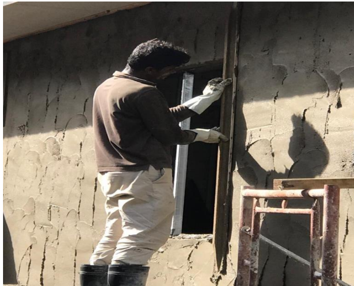
Figure 3.11: Plastering wall process
