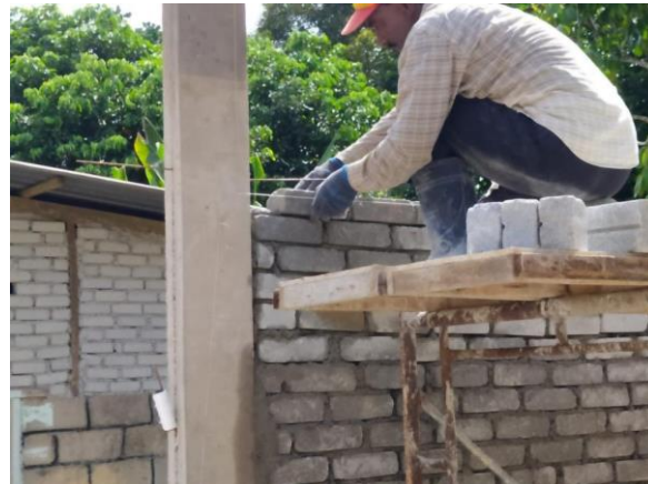
Figure 3.20: the bricklaying process at dining area
