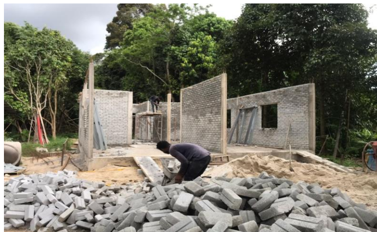
Figure 3.4: The brick that lifted from stockpile to the construction site.
