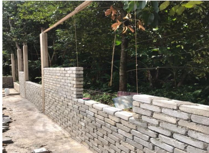
Figure 3.8: The window opening part of the wall.
