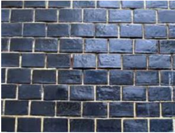
Figure 3.2-21 HEADER BOND
