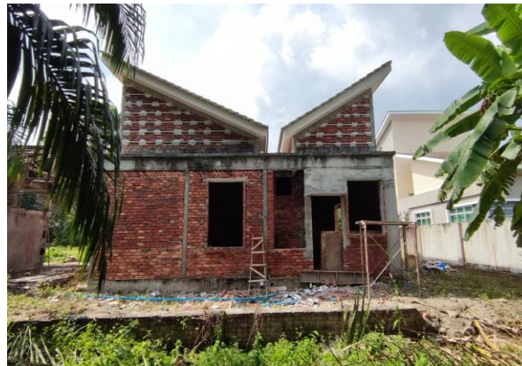
Figure 3.1-7 REAR VIEW OF BUNGALOW
