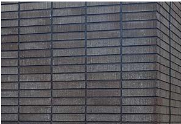
Figure 3.2-22 STACK BOND
