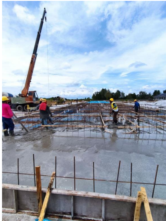
Figure 3.20 Concrete compacting
