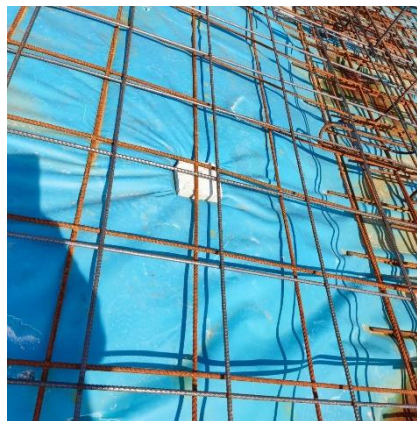
Figure 3.17 Concrete spacer
