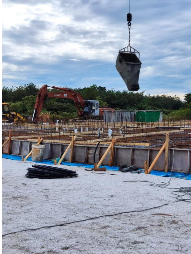
Figure 3.19 Pouring concrete
