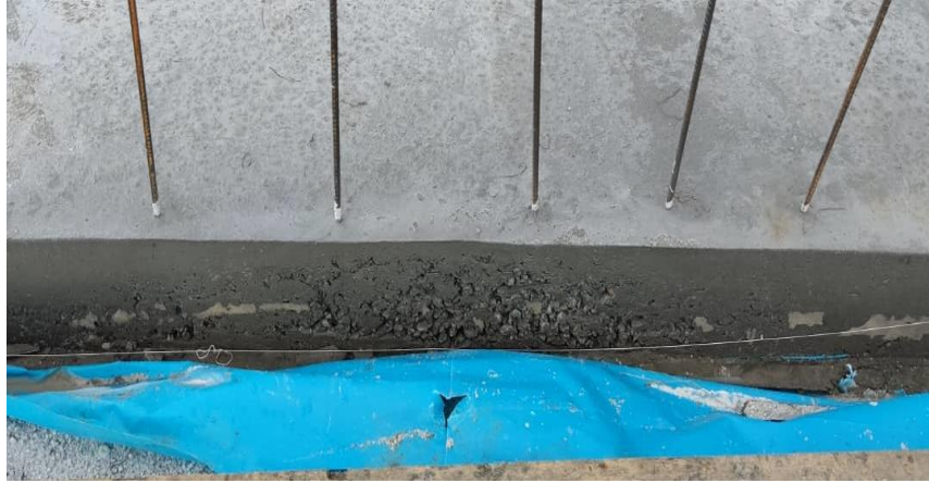
Figure 3.22 Honeycomb
