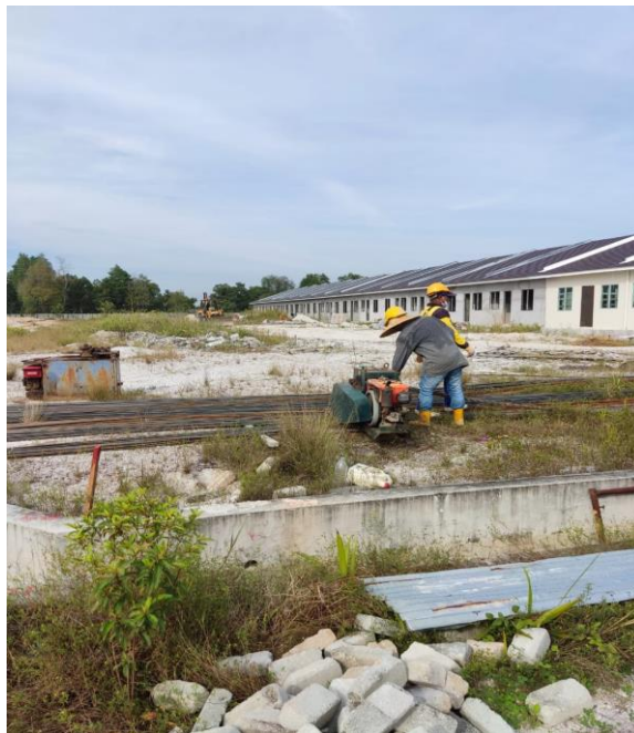
Figure 3.14 Cutting reinforcement bar
