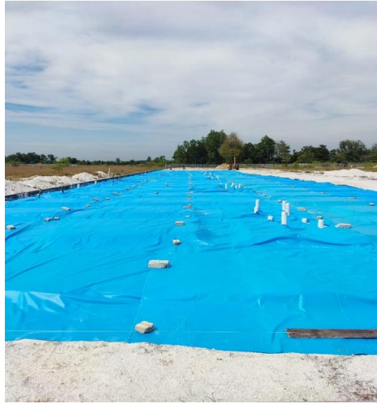
Figure 3.15 Laying DPM sheet
