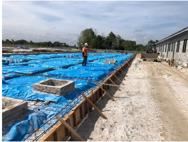
Figure 3.11 Strip footing and slab formwork
