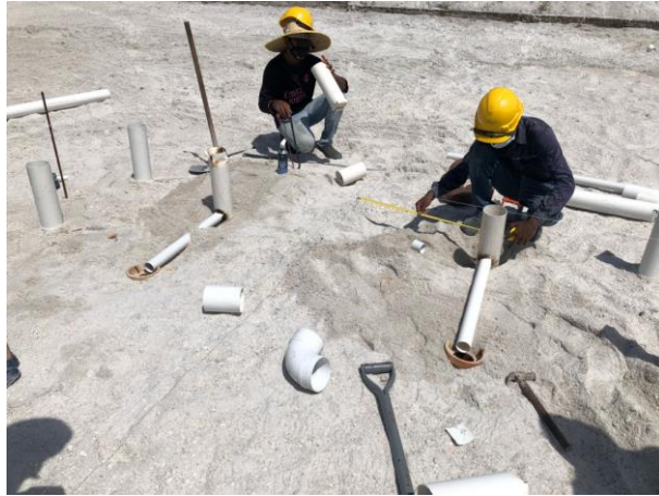
Figure 3.9 Installing sanitary pipe
