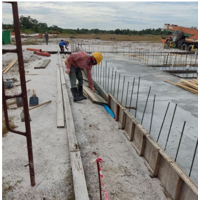
Figure 3.21 Formwork removal
