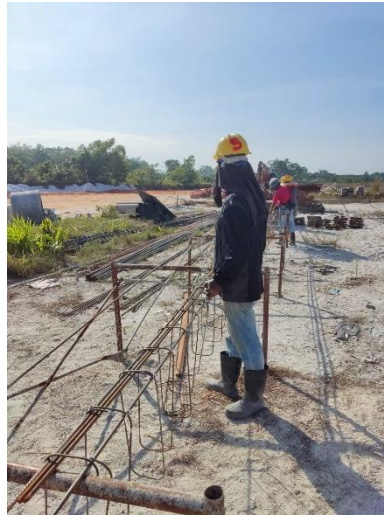
Figure 3.16 Fixing reinforcement bar
