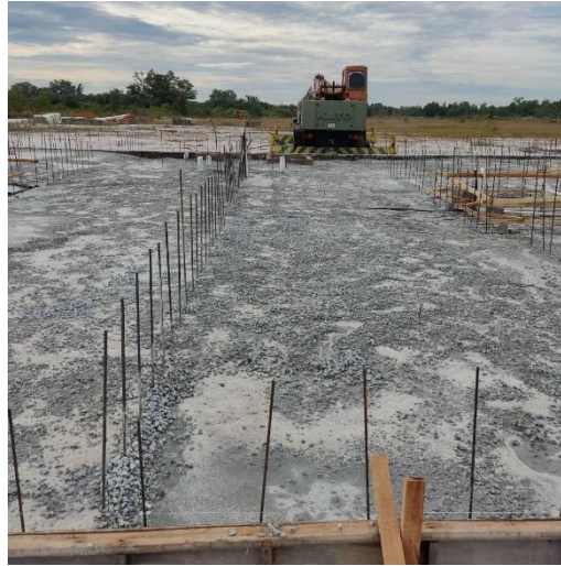
Figure 3.23 Concrete segregation
