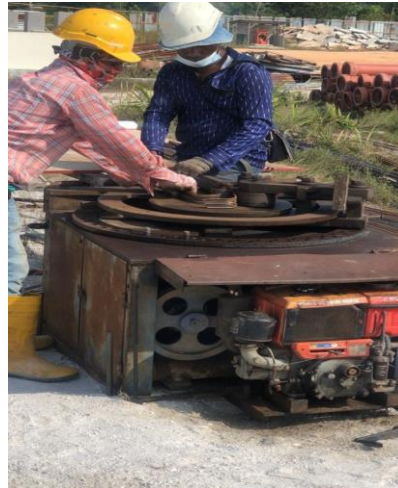
Figure 3.12 Bending reinforcement steel
