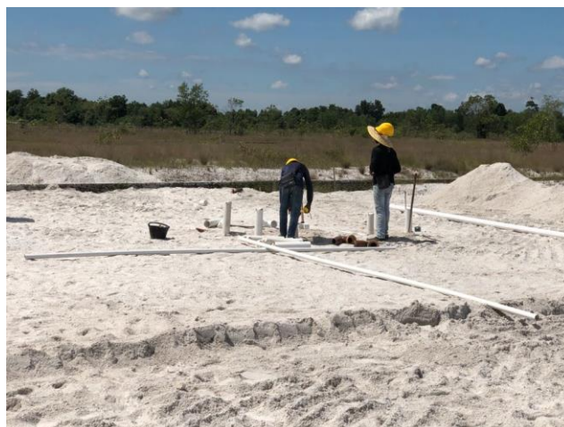
Figure 3.10 Installing sanitary pipes
