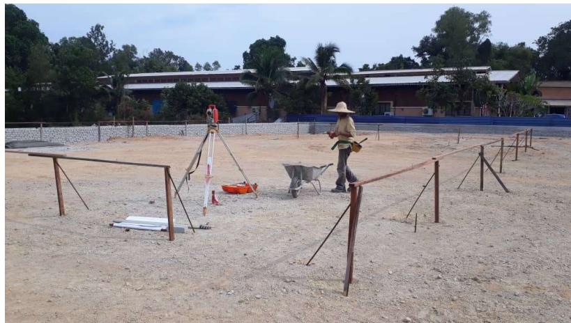
Figure 3.1 Levelling Process
