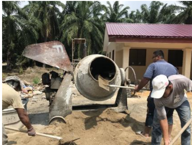
Figure 2 : The workers mixed cement mortar
