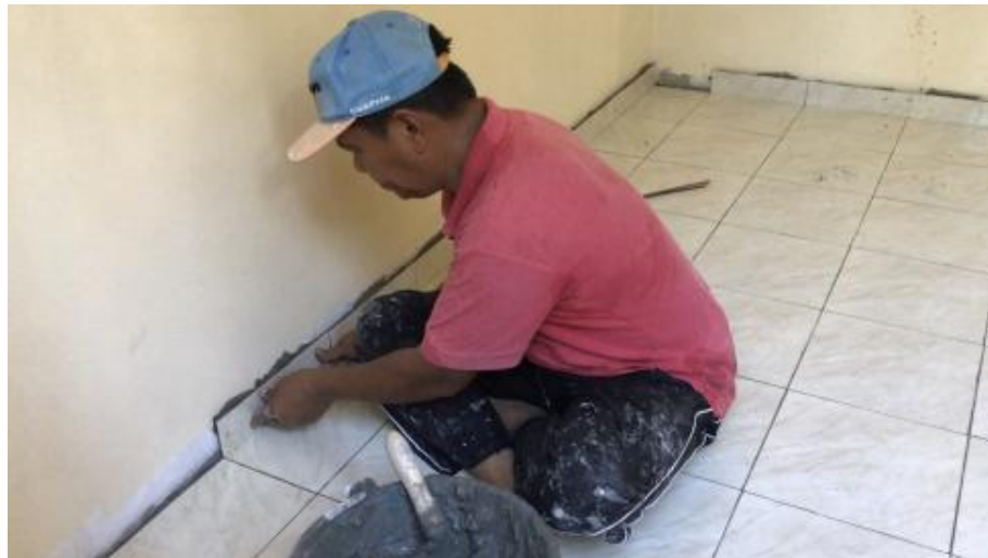
Figure 18 : Ceramic tile placed on the bottom wall
