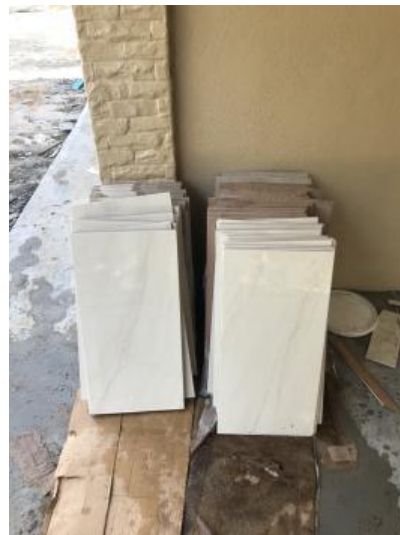
Figure 7 : Tiles dried after soaking
