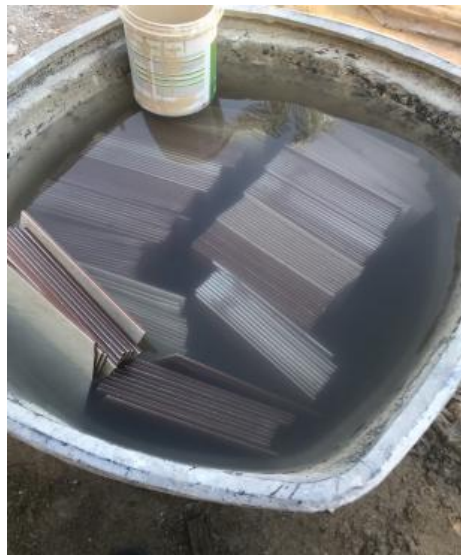
Figure 6 : The tiles soaked in water tank before installation
