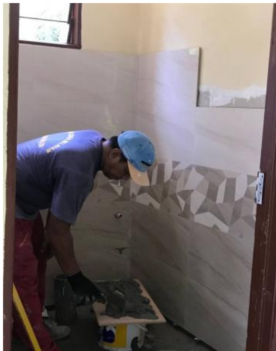
Figure 35 : The installation ceramic tiles for bathroom and toilet
