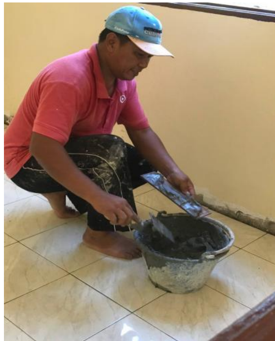
Figure 19 : The installation ceramic tiles for bedroom 1, bedroom 2, bedroom 3.
