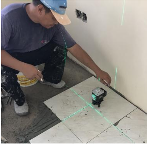
Figure 13 : Identify the tile level.
