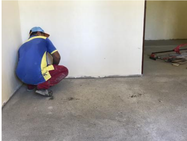
Figure 8 : The worker installed string and pins
