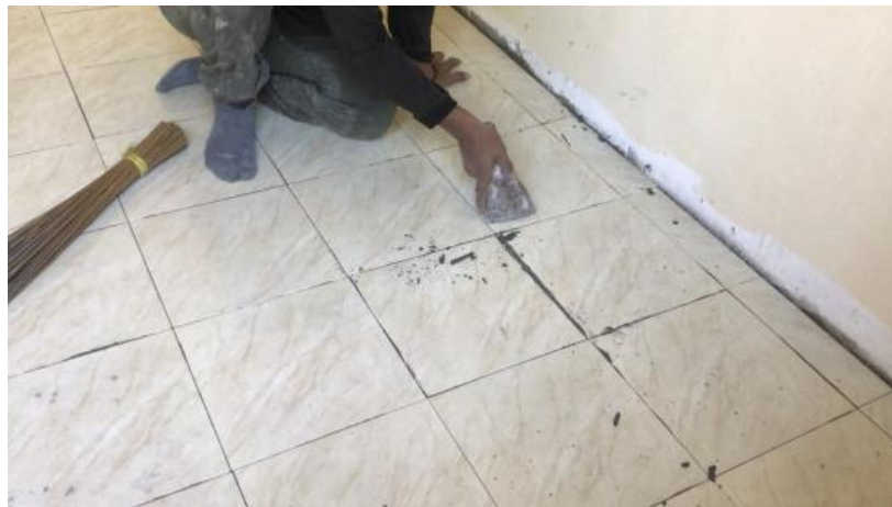
Figure 14 : The mortar removed using scrapper.
