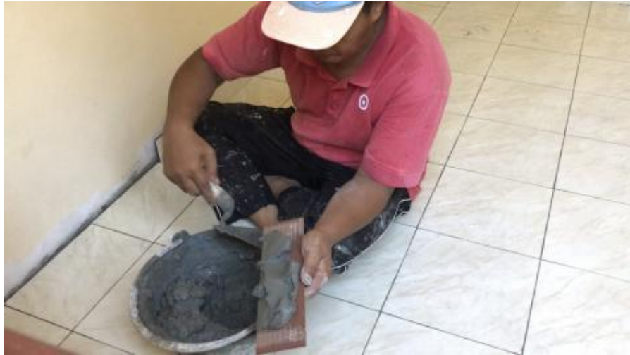
Figure 17 : The worker placed the cement tile
