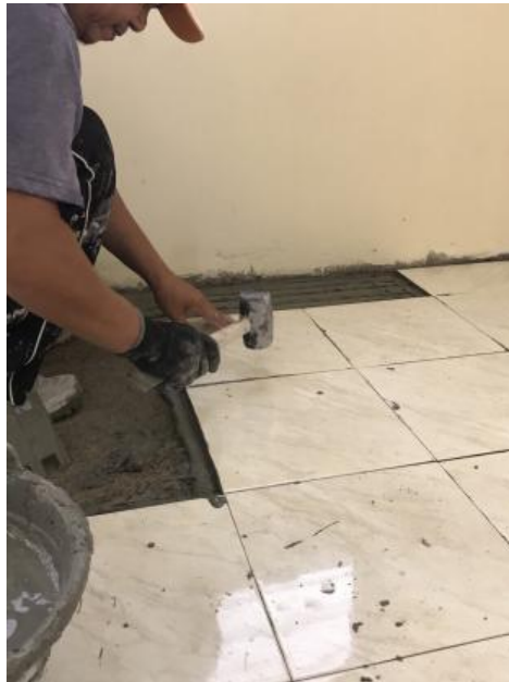
Figure 12 :Ceramic tiles knocked by using rubber hammer
