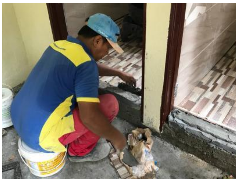
Figure 37 : The installation ceramic tiles for bathroom and toilet.
