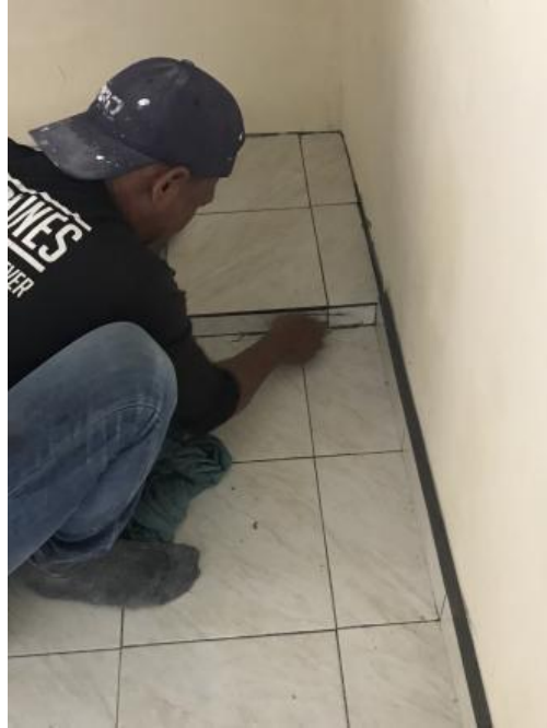
Figure 30 : The installation ceramic tiles for bedroom 3 and kitchen.
