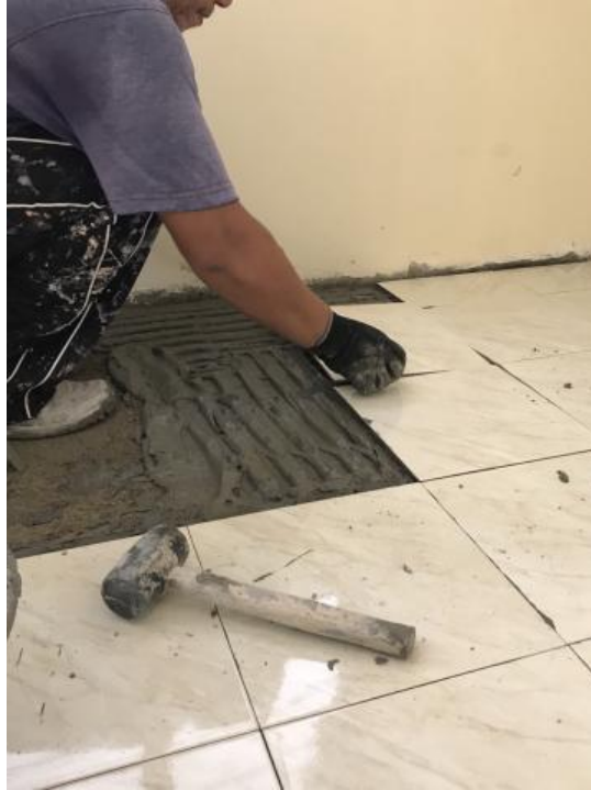
Figure 11 : Ceramic tiles placed on cement tile.
