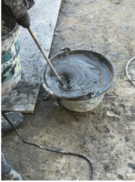
Figure 9 : Cement tile are mixed by using electric mixer.
