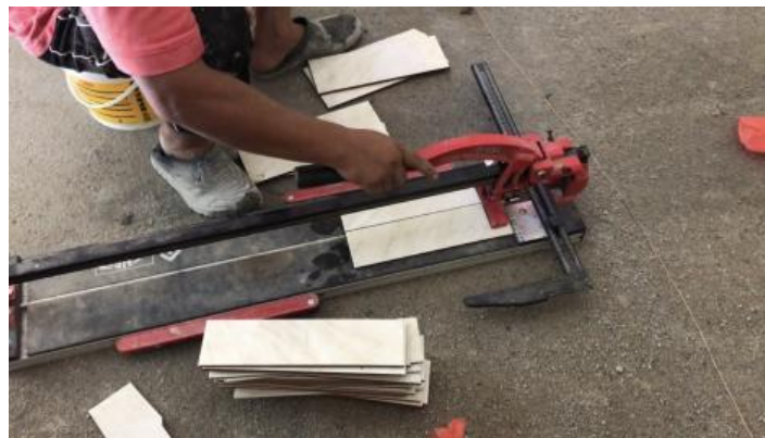
Figure 16 : Cutting the tiles using manual tile cutter
