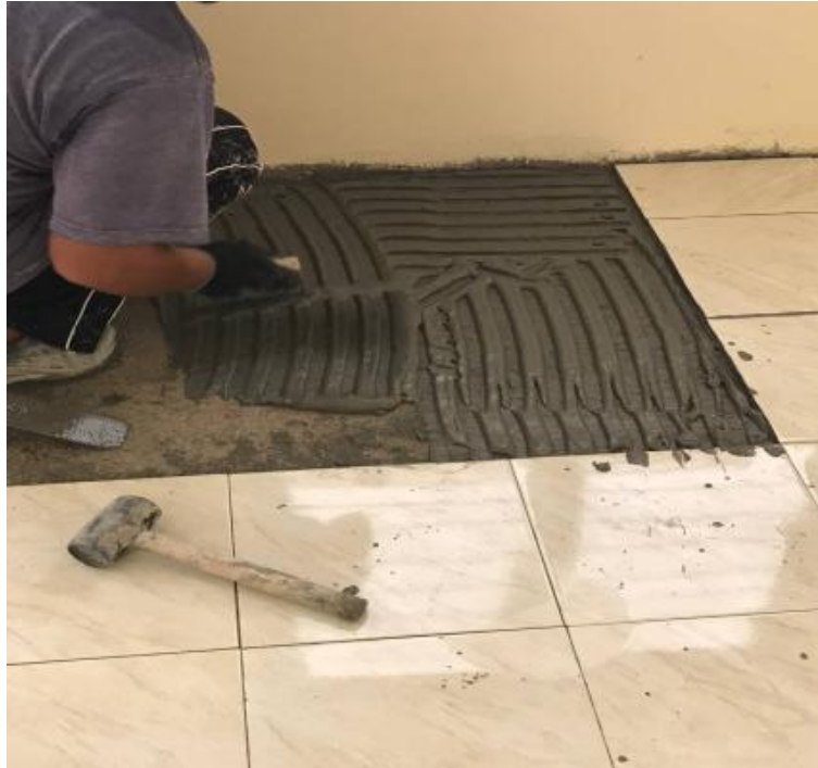
Figure 24 : The installation ceramic tiles for living room
