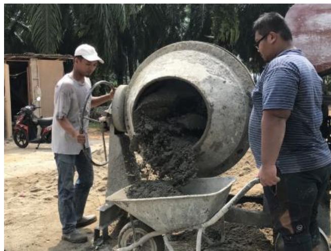
Figure 3 : Cement mortar lifted by worker using wheelbarrow
