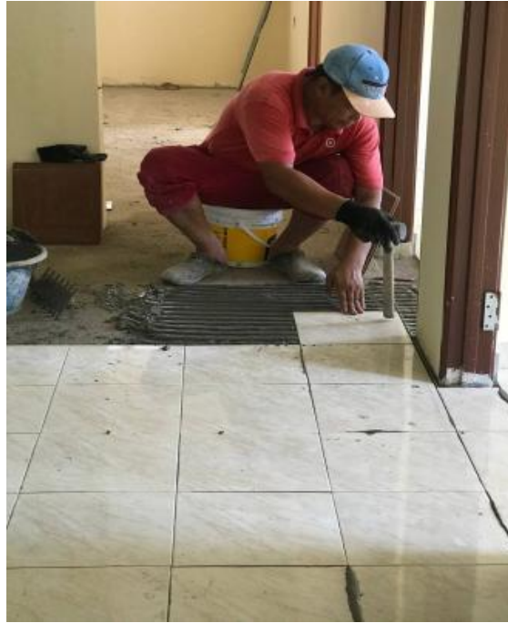
Figure 22 : The installation ceramic tiles for bedroom 3 and kitchen.
