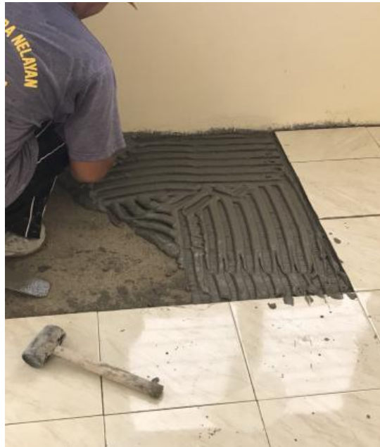
Figure 10 : Cement tile levelled on the floor.
