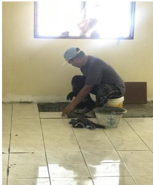
Figure 33 : The installation ceramic tiles for living room
