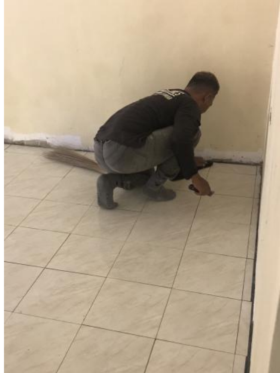
Figure 15 : Wiping the mortar
