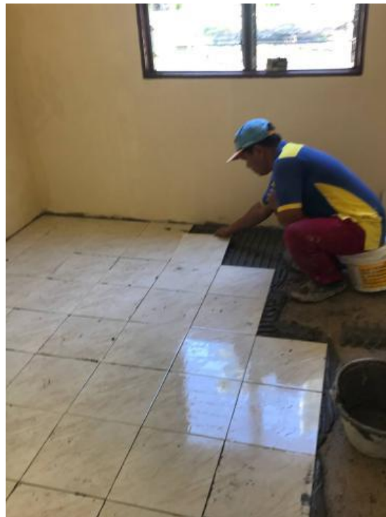
Figure 27 : The installation ceramic tiles for bedroom 1, bedroom 2, bedroom 3
